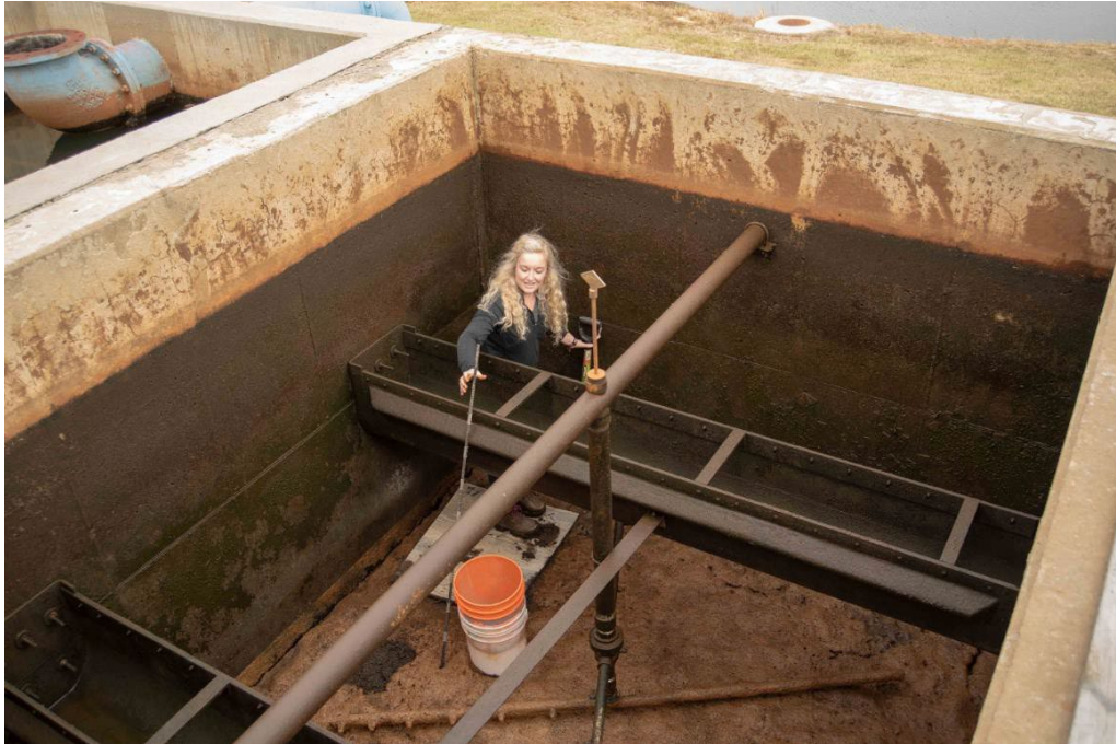
Figure 2: Conducting a Filter Study during the Eufaula CPE.
