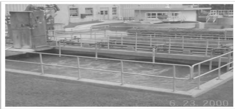
Photo of a working aerated grit chamber
