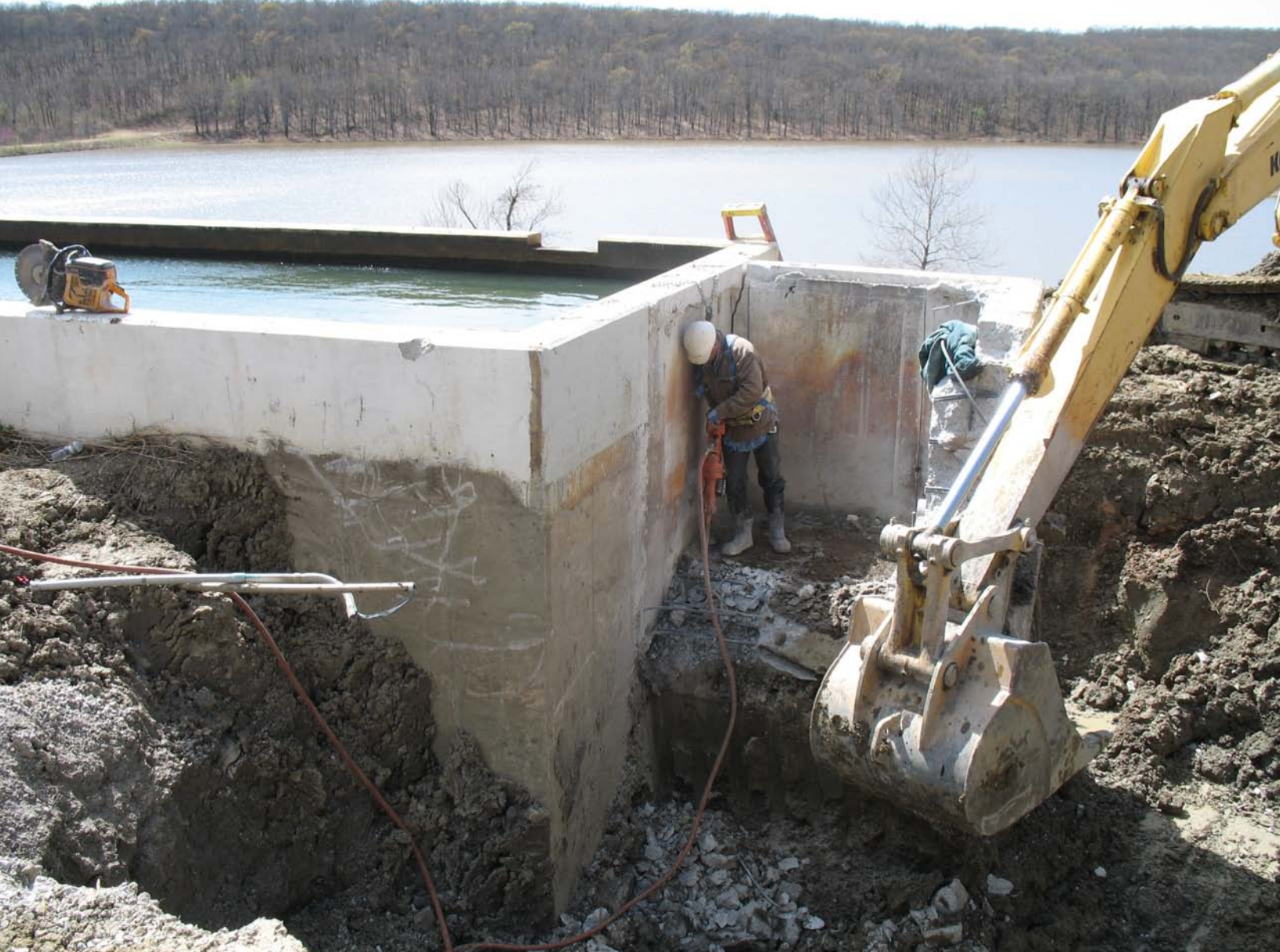
Above: Creek #7 Demolition of the Pre-Sedimentation Basin #2.
