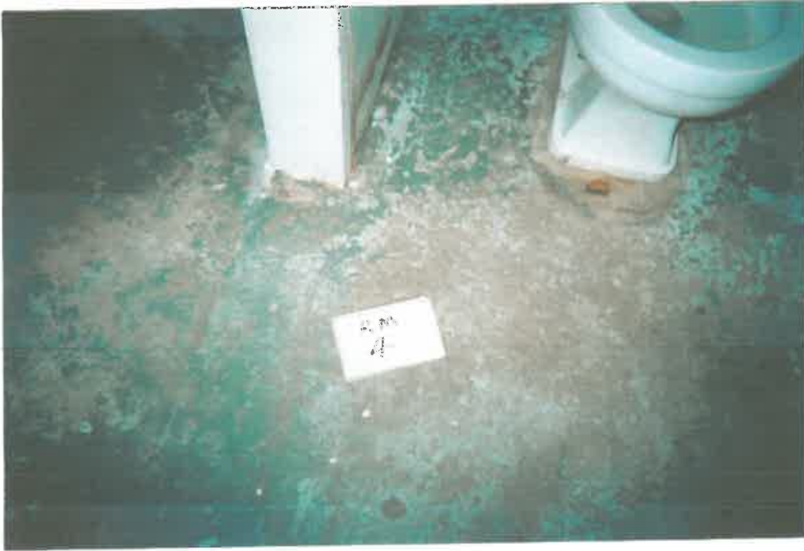
Room 4 - baseboards removed.
