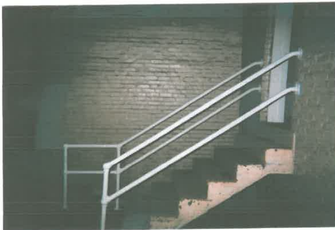
Stair railings after abatement and encapsulation.
