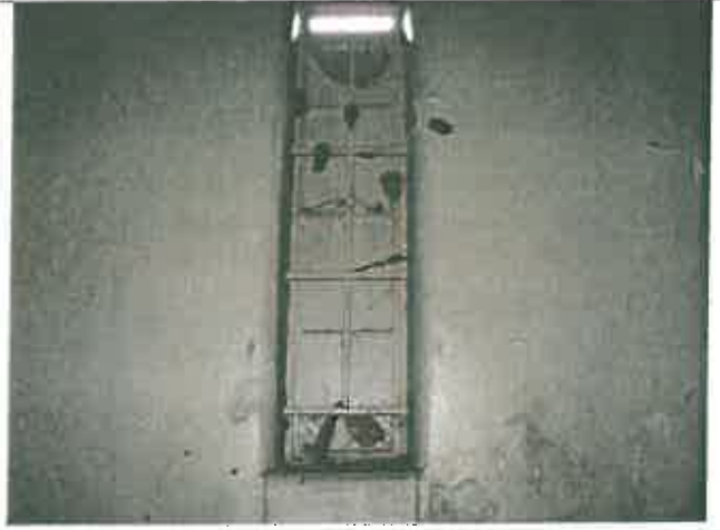
Reading 62, Room 5, Side A, Window guard
