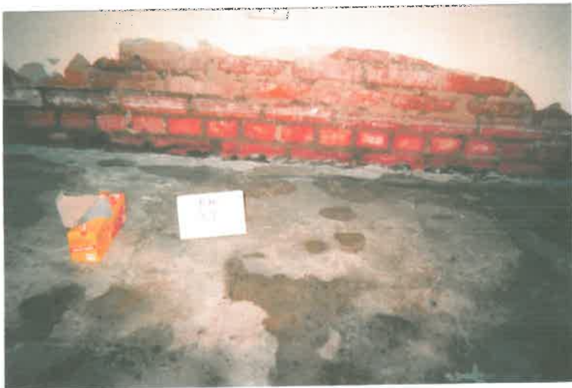
Room 29 - baseboards removed.
