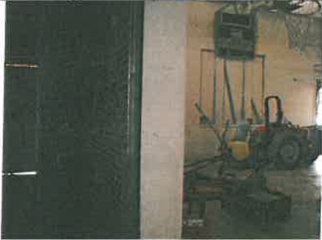
Reading 235, Room 31, Side A, Garage door casing
