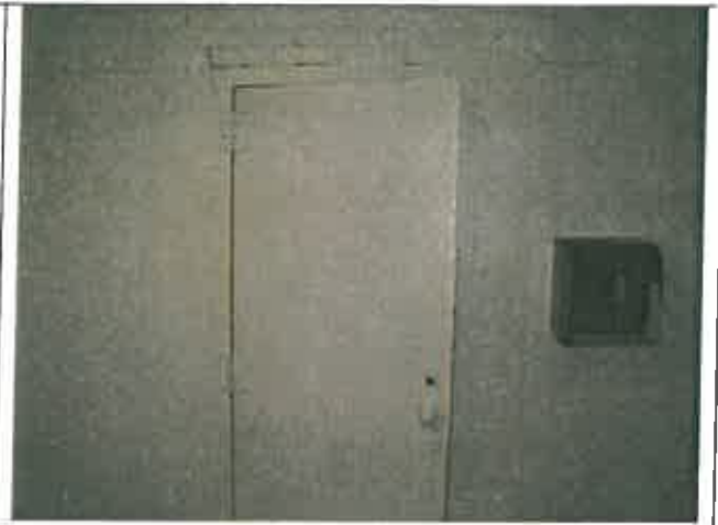
Reading 75, Room 6, Side C, Door
