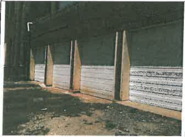
Reading 248, Exterior, Side D, Garage door casing
