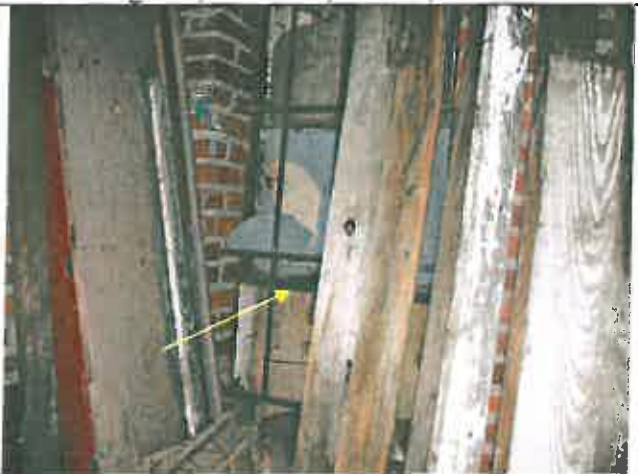
Reading 232, Room 30, Side C, Window sash
