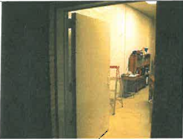
Readings 45 & 46, Room 34, Side A, Door and casing
