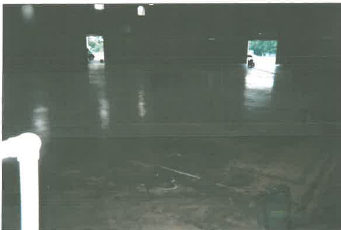
Drill floor after cleaning.
