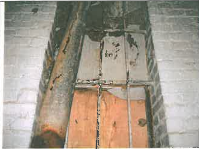
Reading 36, Room 2, Side A, Window guard
