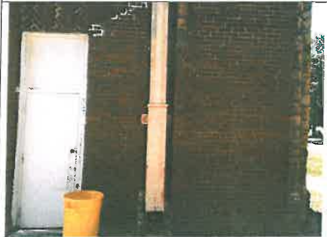
Reading 244, Exterior, Side B, Gutter downspout
