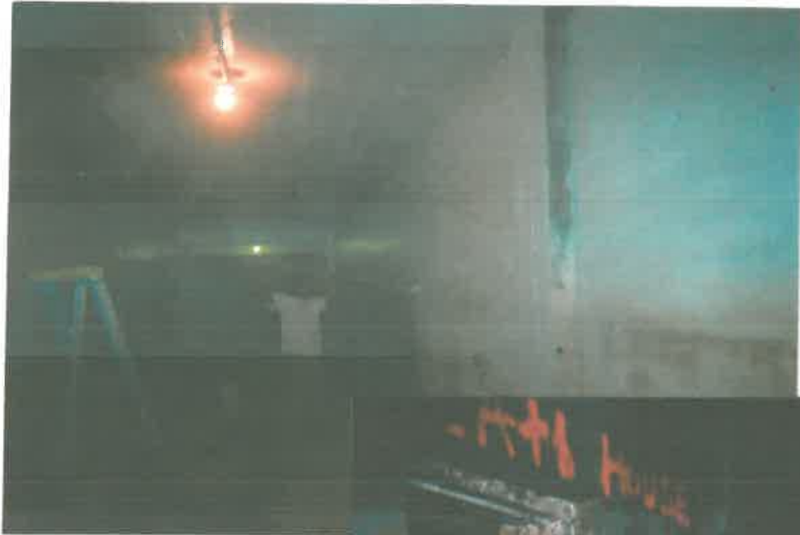
IFR - walls being encapsulated.
