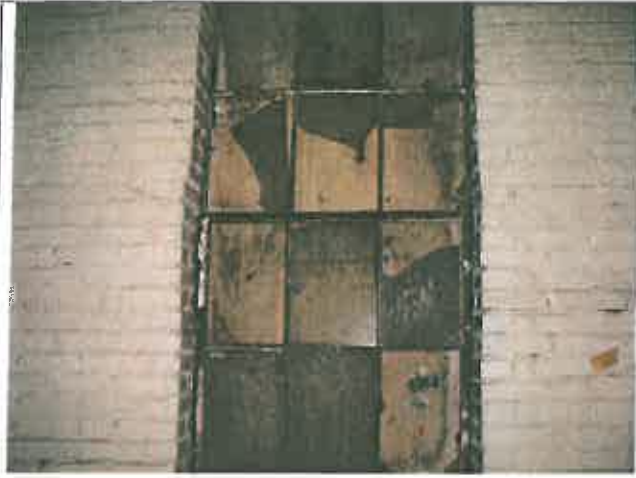
Reading 146, Room 17, Side B, Window sash
