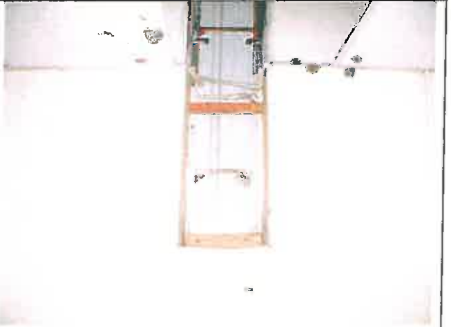
Reading 224, Room 28, Side C, Window sash
