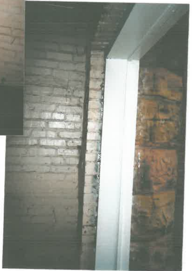
Door frame encapsulated.
