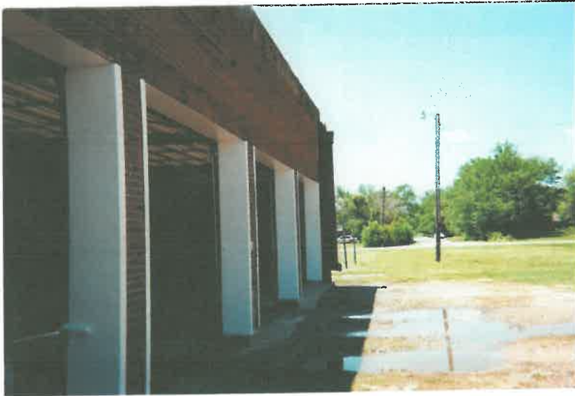
Garage door frames being encapsulated.
