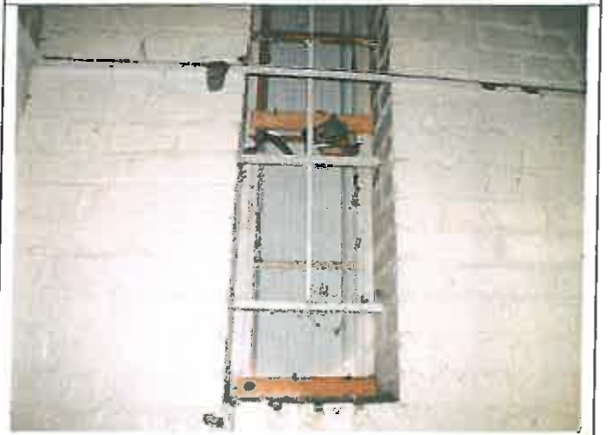
Reading 203, Room 25, Side C, Window sash
