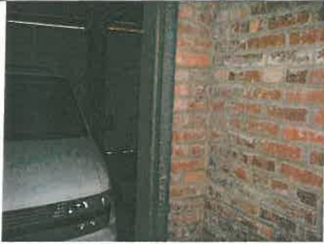
Reading 233, Room 30, Side D, Door casing
