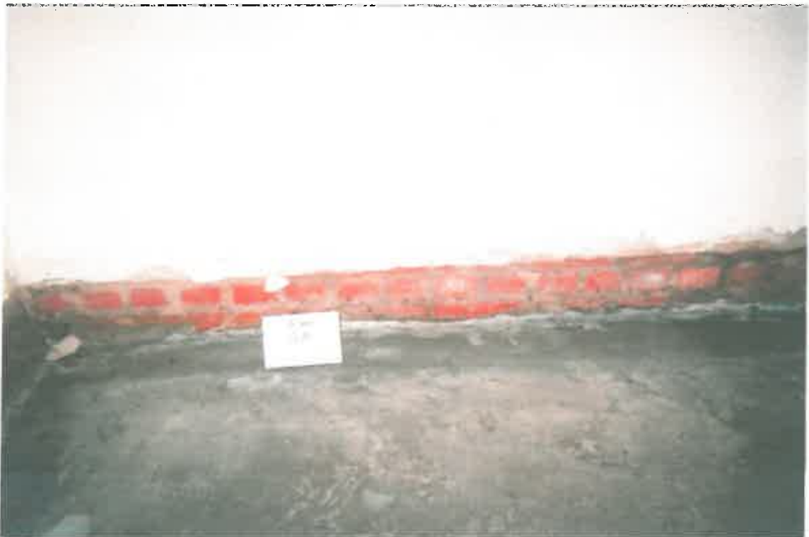
Room 28 - baseboards removed.
