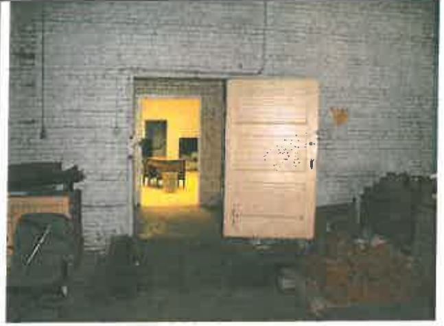
Readings 38 & 39, Room 2, Side B, Door and casing
