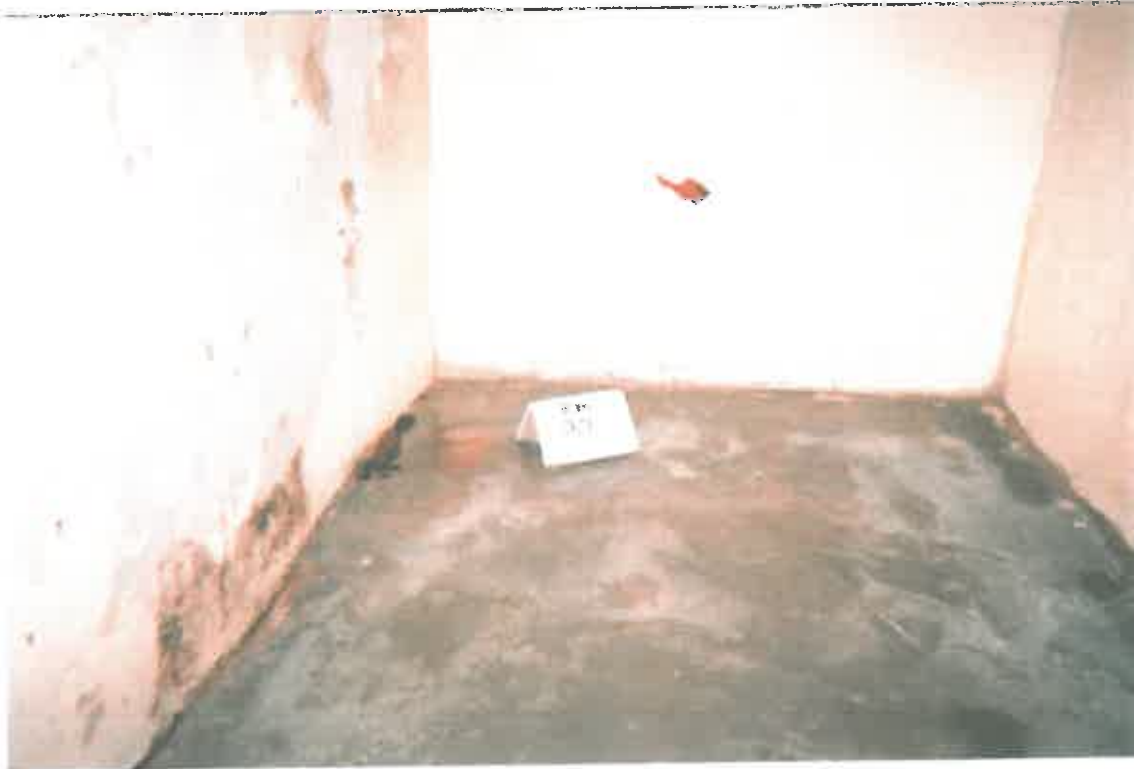
Room 29 - baseboards removed.
