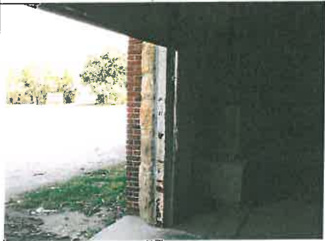
Reading 25, Room 1, Side D, Garage door casing
