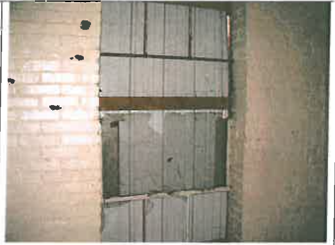
Reading 147, Room 18, Side B, Window sash
