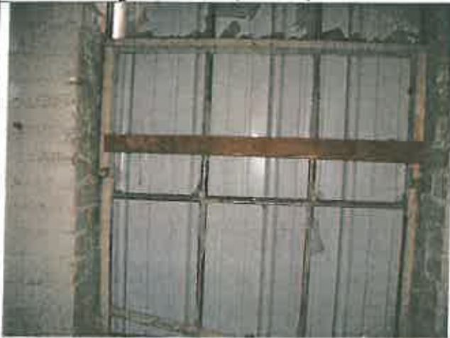
Reading 121, Room 14, Side B, Window sash
