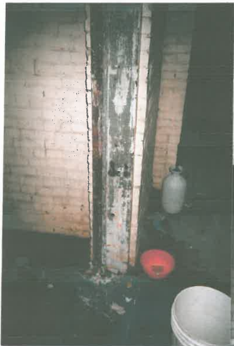
Door frame being abated.
