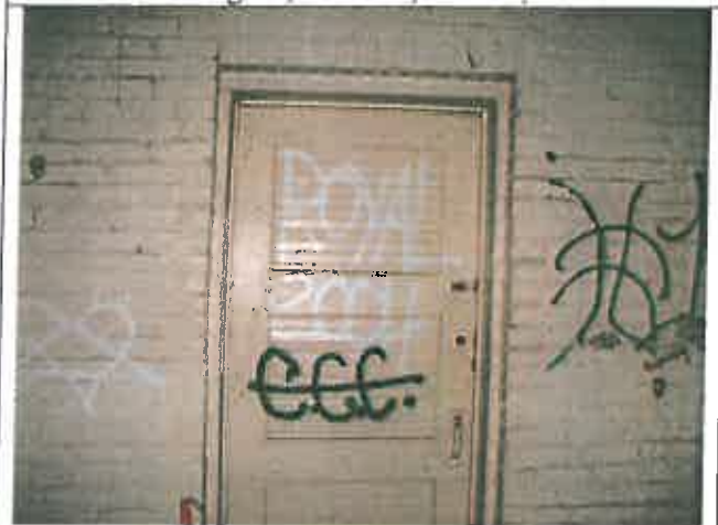
Reading 132 & 133, Room 15, Side A, Door and casing
