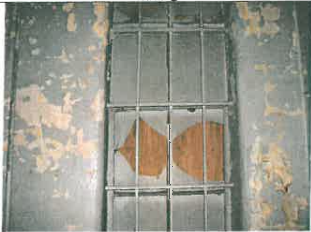
Reading 61, Room 4, Side A, Window guard
