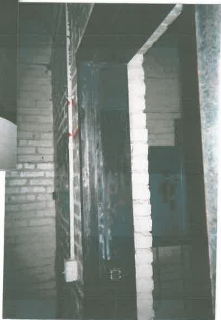
Door frame abated and ready for encapsulation.
