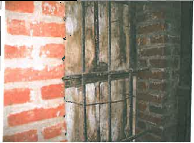
Reading 234, Room 31, Side C, Window sash
