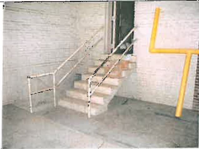
Readings 18-20, Room 1, Side B, Stair handrail, treads, and risers
