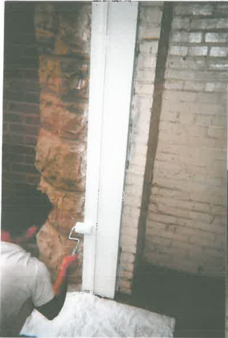
Door frame being encapsulated.
