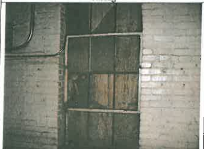
Reading 135, Room 15, Window sash
