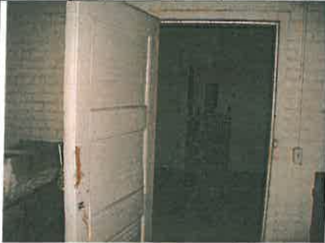
Reading 148 & 149, Room 18, Side A, Door and casing
