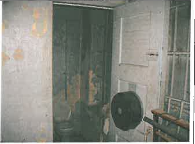
Reading 60, Room 4, Side D, Door casing
