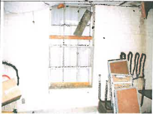
Reading 185, Room 23, Side B, Window sash
