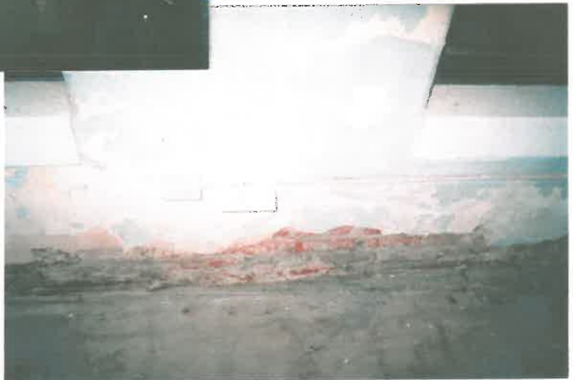
Room 4 - baseboards removed.
