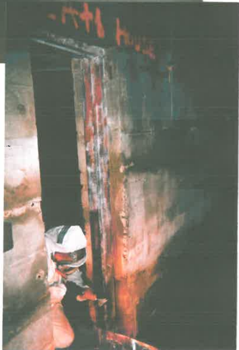
IFR - door frame being abated.
