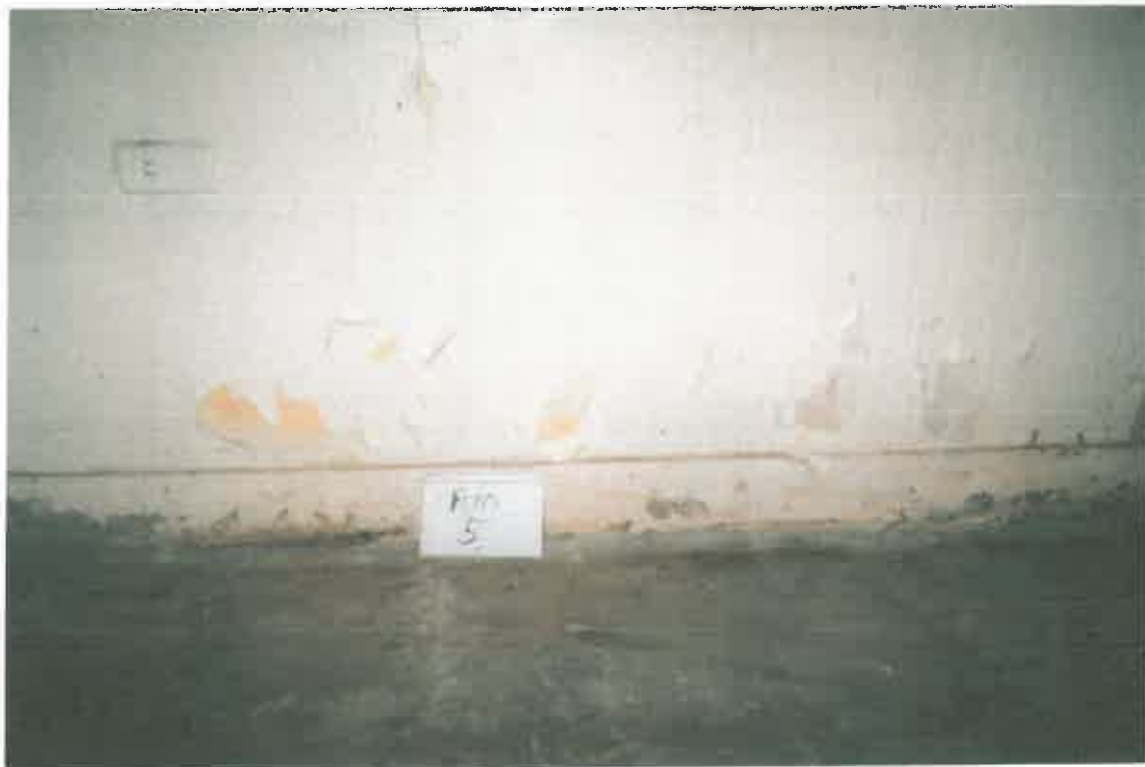
Room 5 - floor tile and mastic removed.
