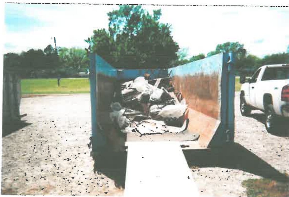
Non-ACM waste in dumpster awaiting disposal.
