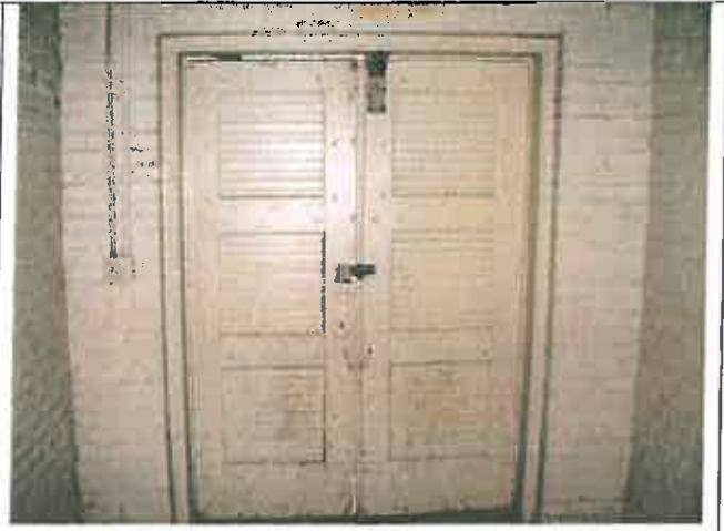
Reading 213 & 214, Room 27, Side C, Door and casing
