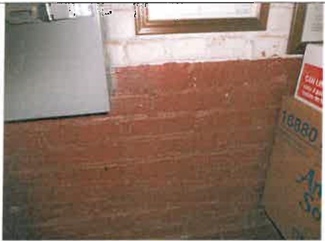
Rd. 5-9, Room 01, Walls
