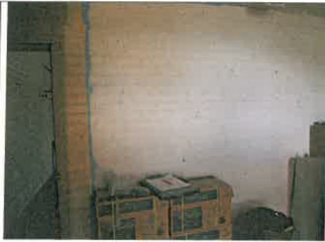
Rd. 39, Room 03 Wall
