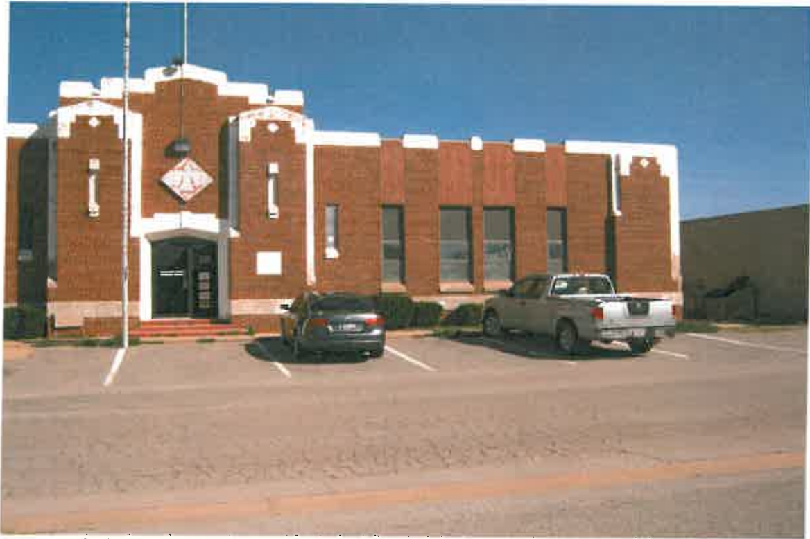
Windows on South Side of Building Have Been Replaced and Do Not Have Asbestos Containing Window Caulking
