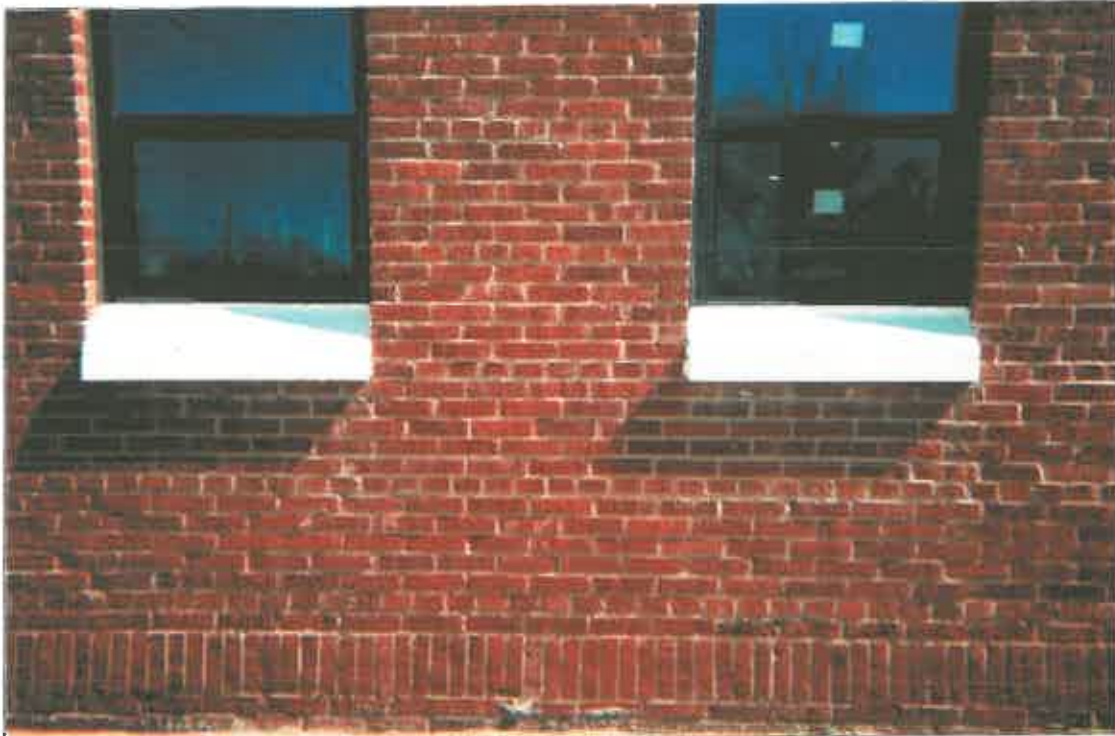
SEALED WINDOW LINTELS AND SILLS
