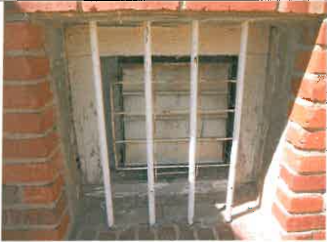
Rd. 181,183, Exterior, IFR Vent, Wood and Bars
