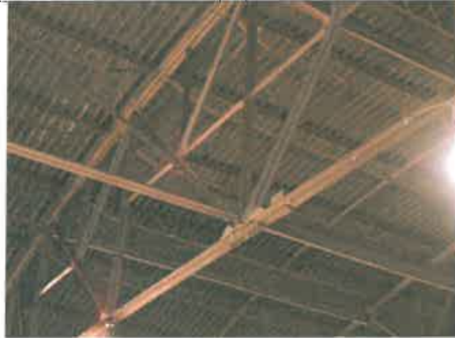
Rd. 194-196, Room 01, Beams, Joist, Braces
