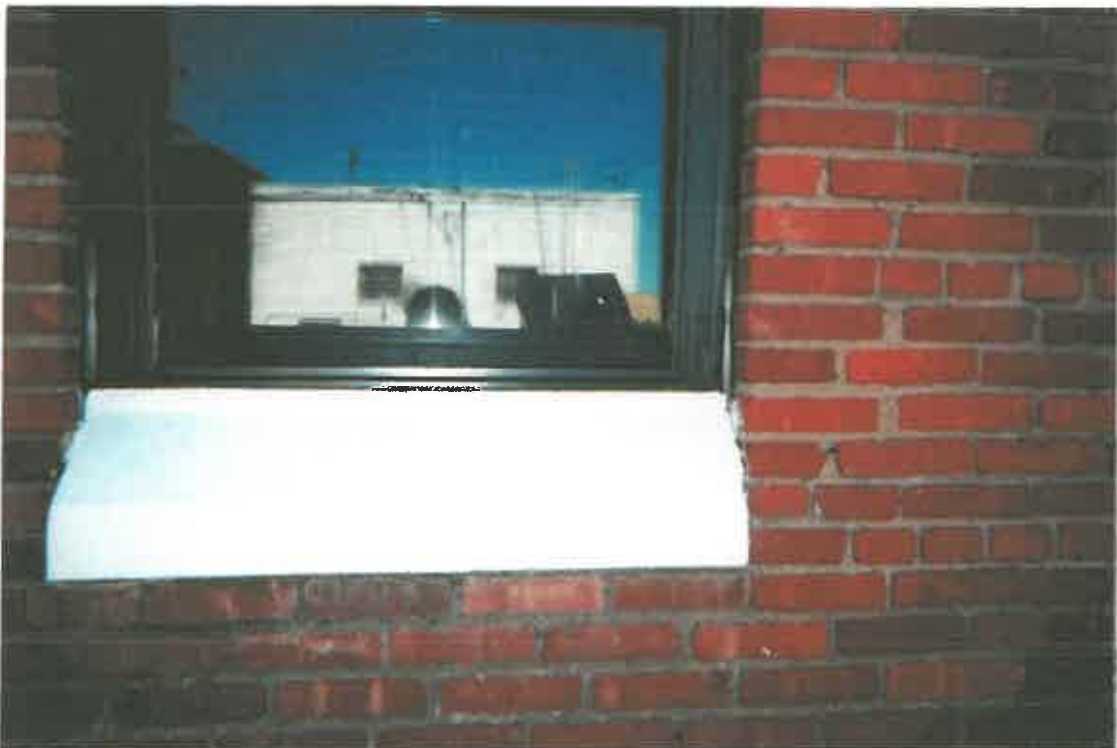
SEALED WINDOW LINTELS AND SILLS
