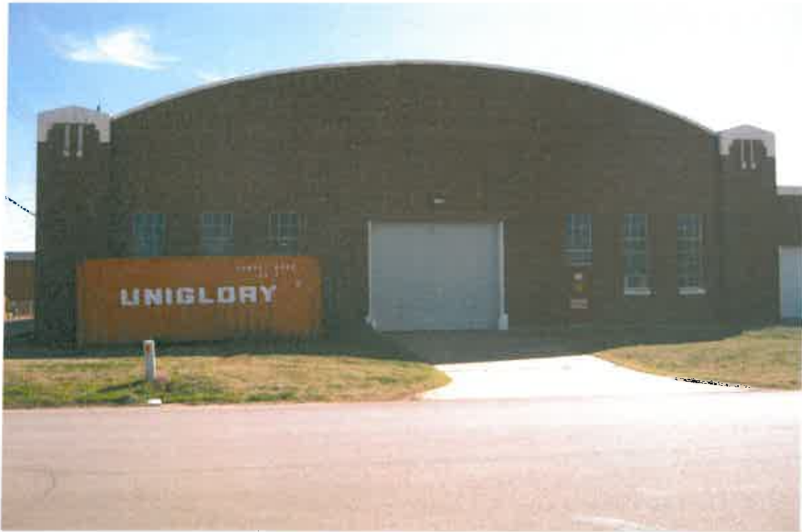
Friable Asbestos Containing Window Caulking, West Side
