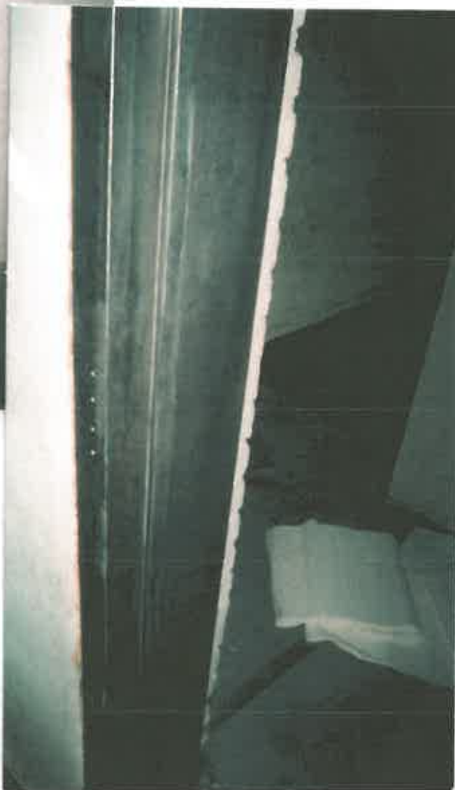
DOOR FRAME - STRIPPED OF LBP TO BARE METAL
