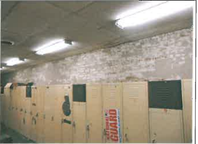
Rd. 168, Room 21, Walls
