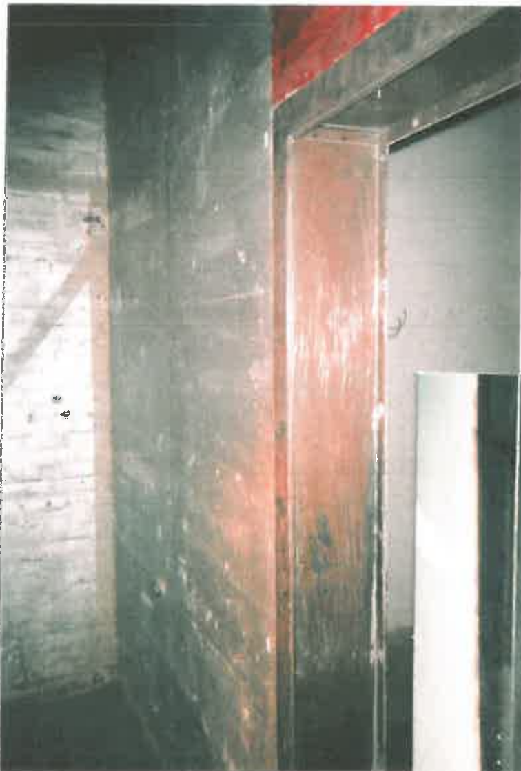
DOOR FRAME - STRIPPED OF LBP TO BARE METAL
