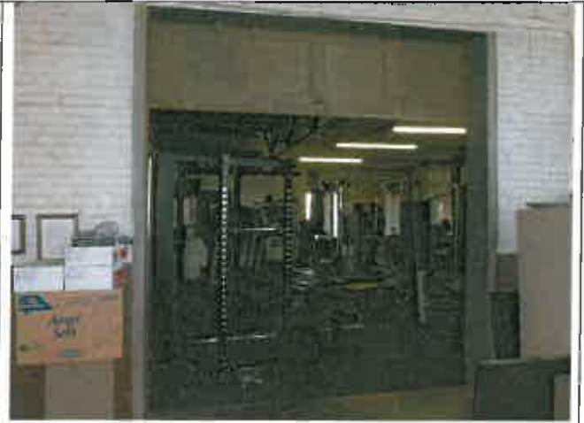
Rd. 23-24, Room 01 Overhead Door, 9' x 10'
