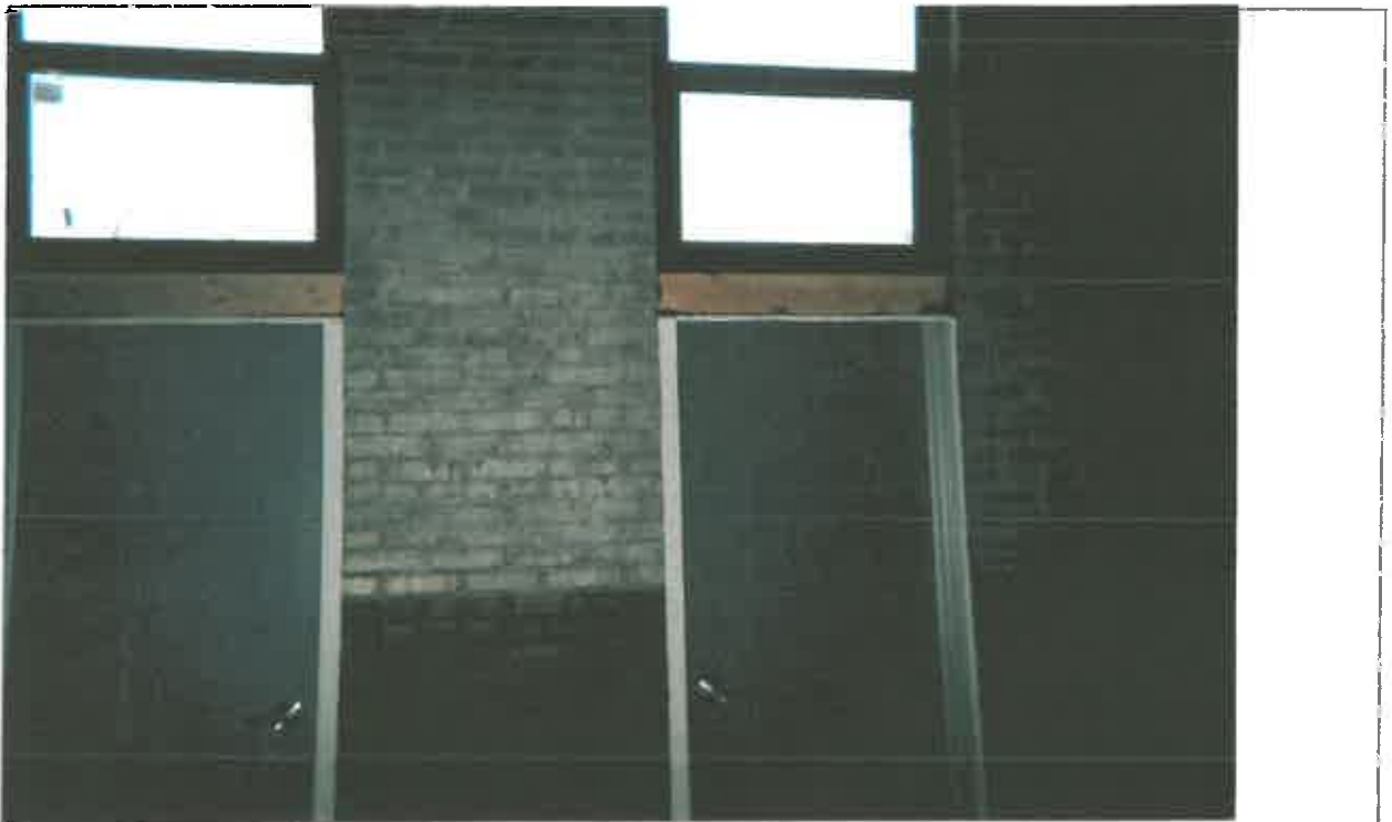
SEALED FRAMES, NEW DOORS AND WINDOWS
