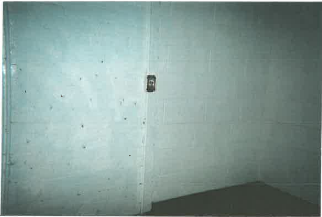
SEALED WALL AFTER LOOSE AND PEELING
