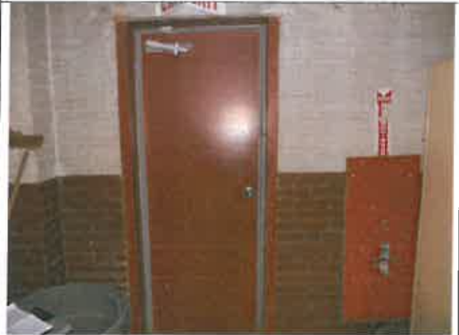
Rd. 27, Room 01 Door Frame, "84 x 36"
