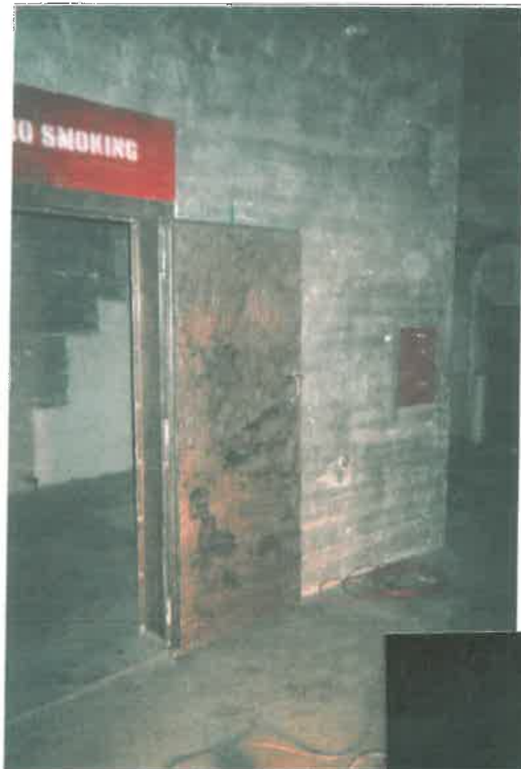
VAULT DOOR AND FRAME - STRIPPED TO BARE METAL
