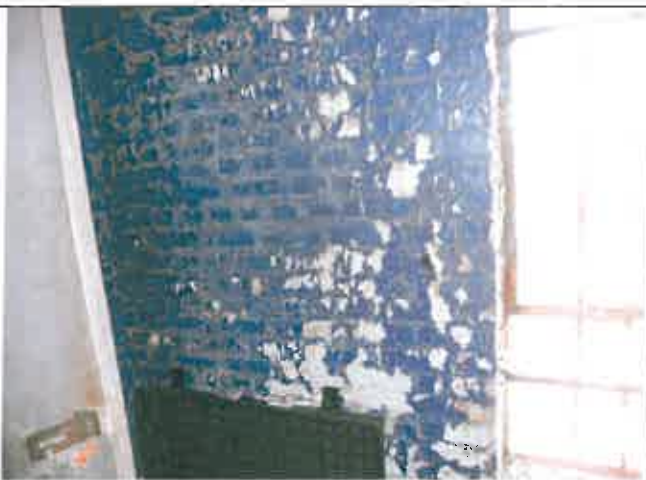
Rd. 31, Room 02 Wall
