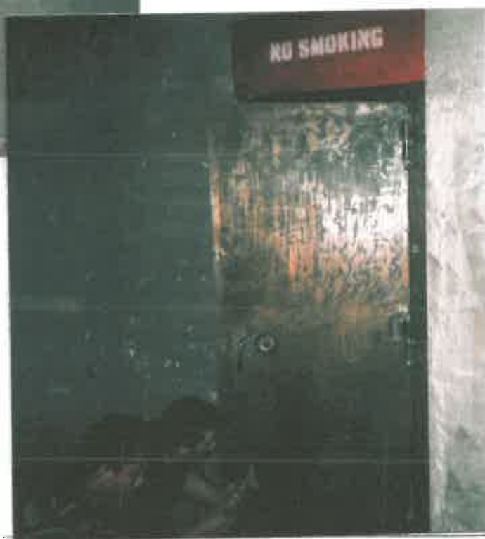
VAULT DOOR AND FRAME - STRIPPED TO BARE METAL
