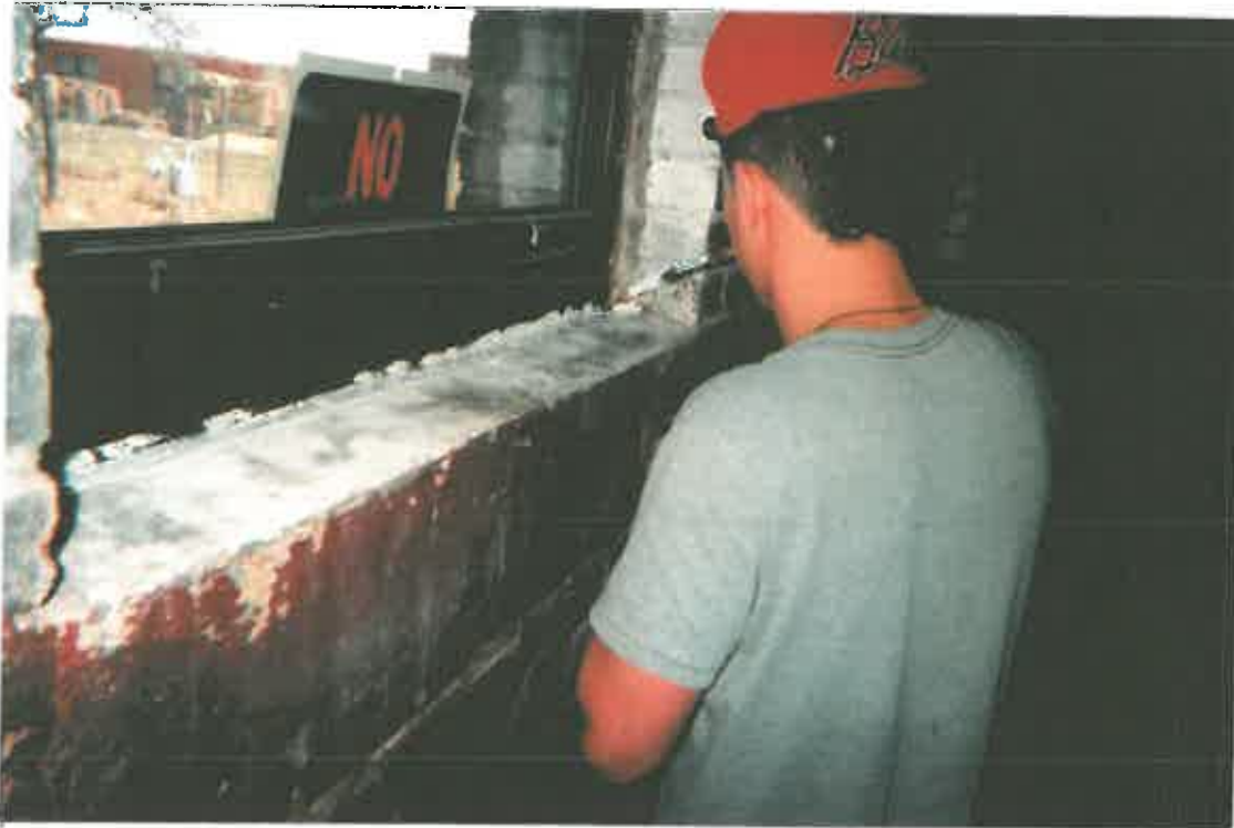
WINDOW SILL - STRIPPED OF LOOSE AND PEELING PAINT
