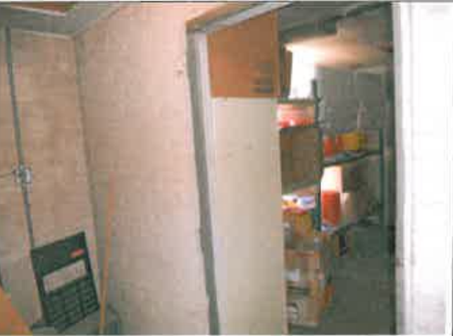
Rd. 156, 159, Room 20, Walls
