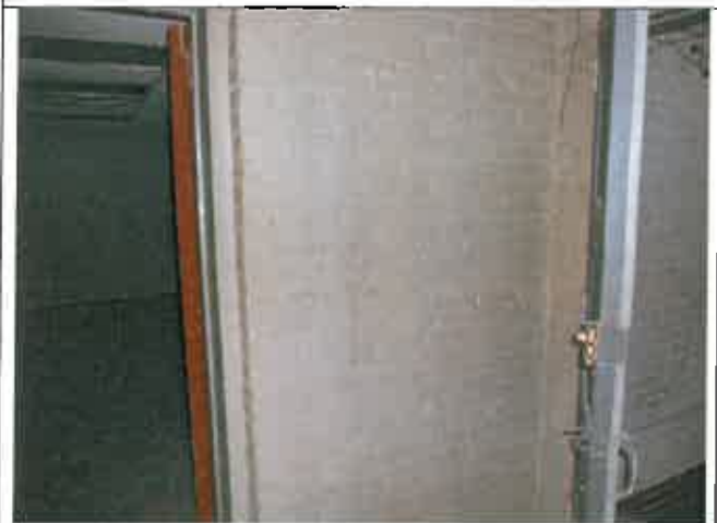
Rd. 34-36, Room 03 Walls
