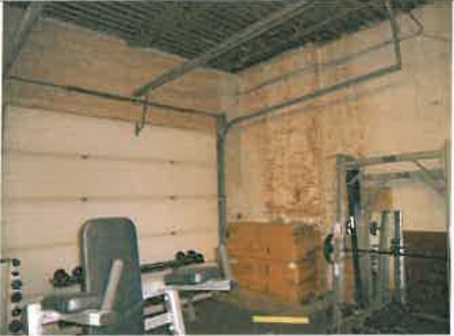
Rd. 125, 127, Room 15, Walls
