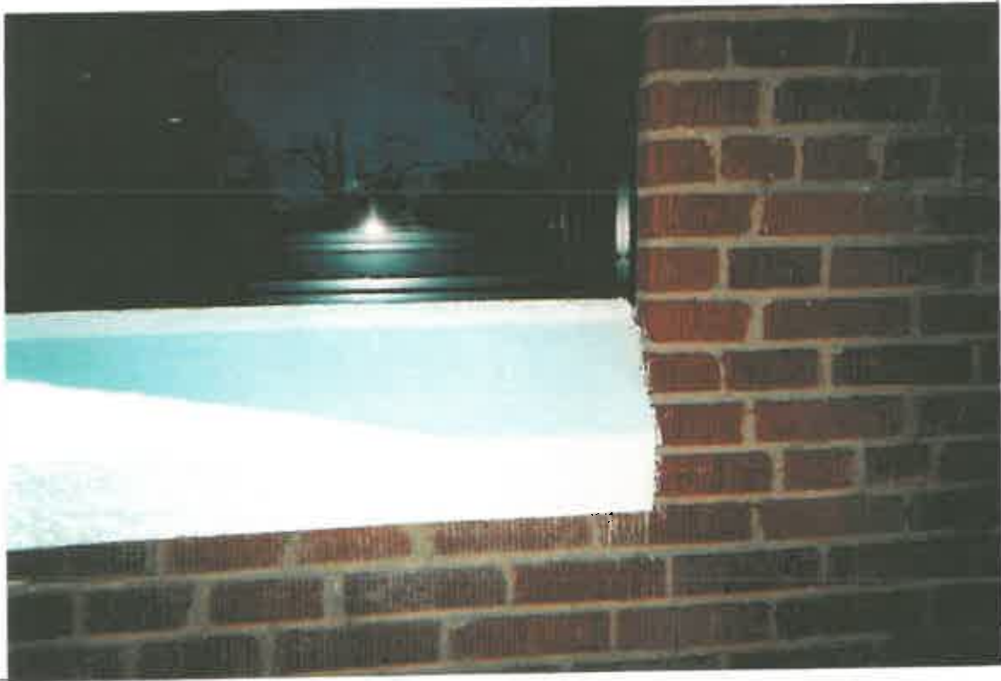
SEALED WINDOW SILL
