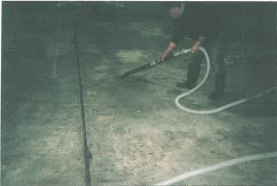
DRILL FLOOR CLEANING
