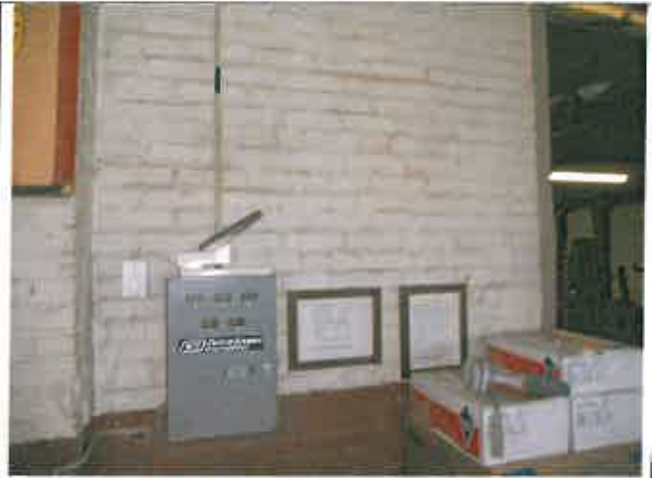
Rd. 5-9, Room 01, Walls
