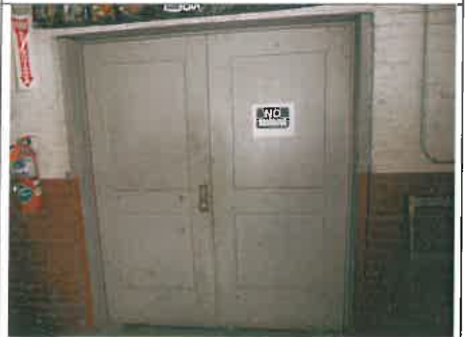
Rd. 19-20, Room 01 Doors and Frame, 2 Doors 83" x 37"
