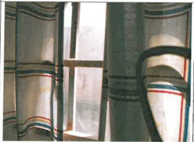
Rd. 71, Room 05, Bars on Window
