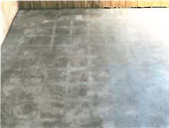
Photo #3: Following Re-cleaning
