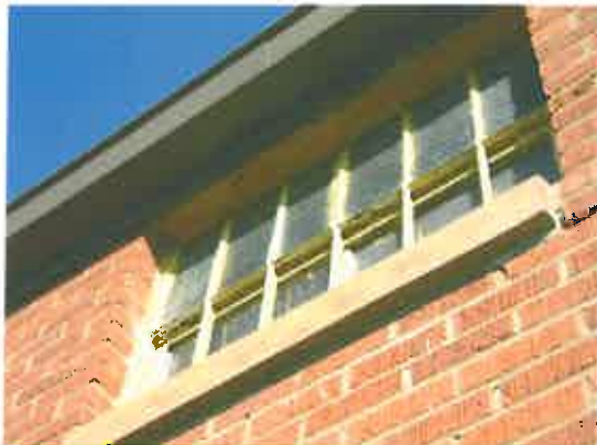
Photo #17: Grey-painted window lintel on Side D - LBP.
