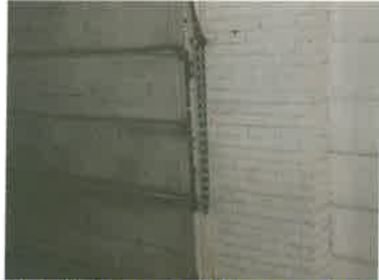
Photo #2: Beige-painted rollup door and metal frame - LBP.
