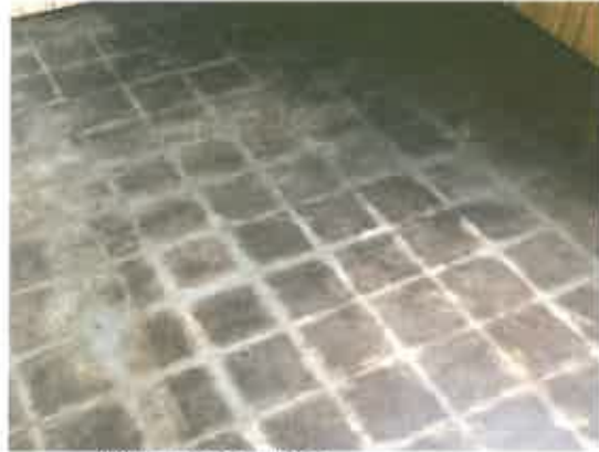
Photo #4: Following Re-cleaning
