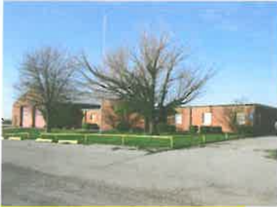
Photo #1: Walters National Guard Armory.
