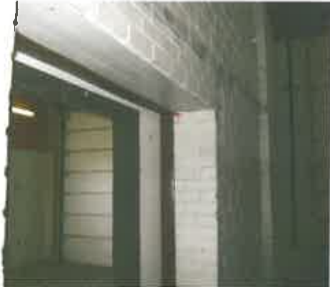
Photo #7: View of white painted lintel, Room 16, Side B - LBP.
