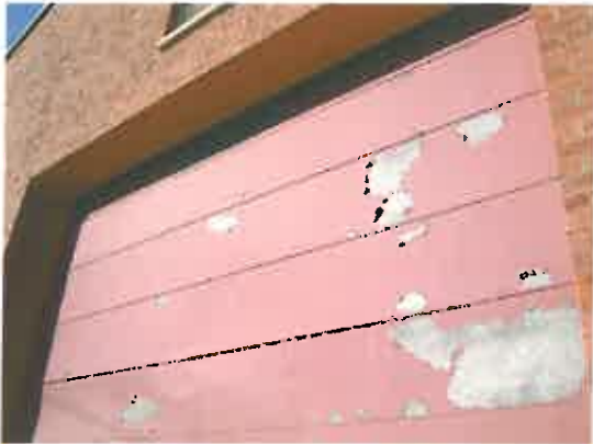
Photo #13: Yellow-painted rollup door lintels, on Sides A & D - LBP.
