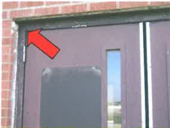
Photo #3: Brown-painted metal door frame, Room 23 - LBP.
