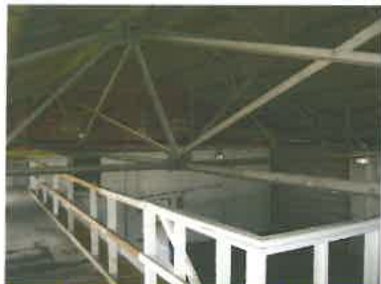
Photo #6: Gray-painted metal bar joist/trusses, Room 16 - LBP.
