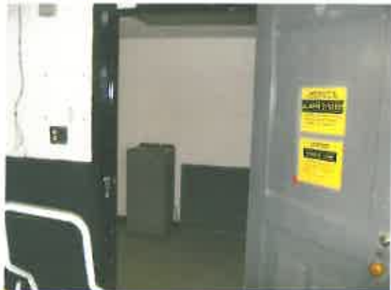
Photo #5: Gray-painted metal door, Room 16 - LBP.
