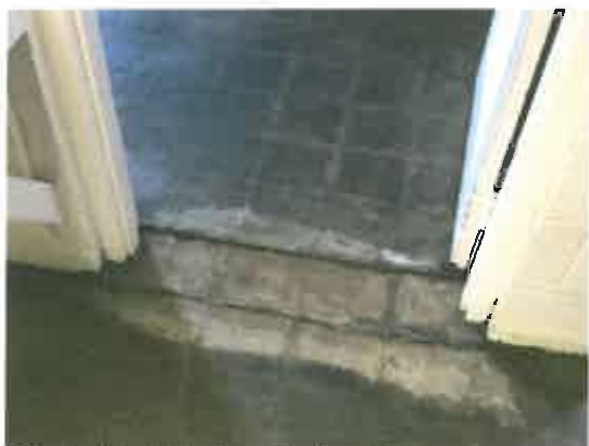
Photo #6: Following Re-cleaning
