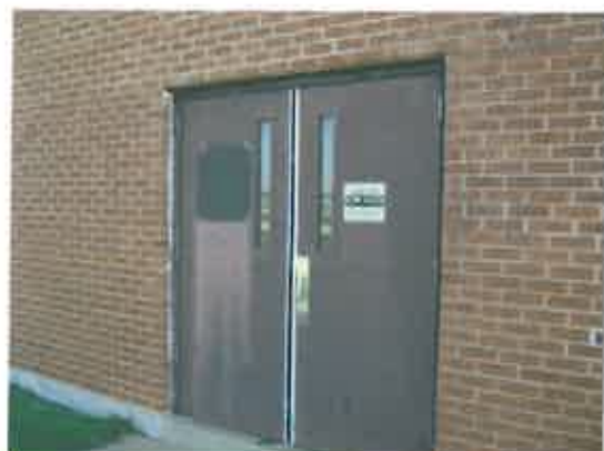
Photo #12: Brown painted metal door lintel, as found on Sides A & C - LBP.
