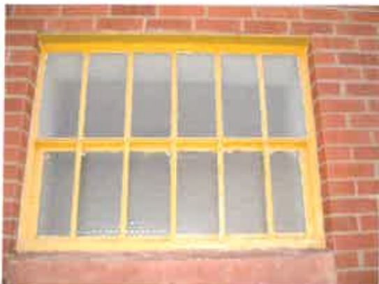
Photo #11: Yellow-painted window frame and lintel - LBP.
