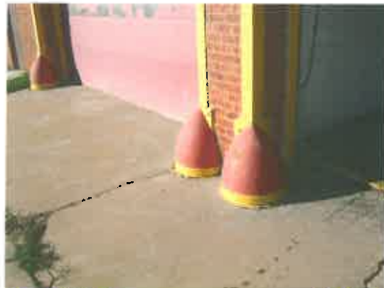
Photo #14: Red-painted metal modified bollards on Sides A and D- LBP.
