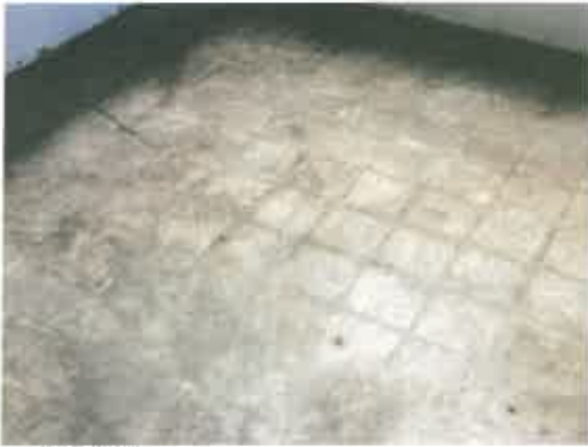
Photo #1: Following Re-cleaning
