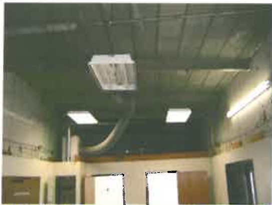
Photo #9: I-beams and kaylo ceiling, Room 23 - LBP.
