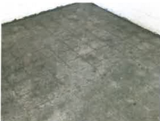
Photo #5: Following Re-cleaning
