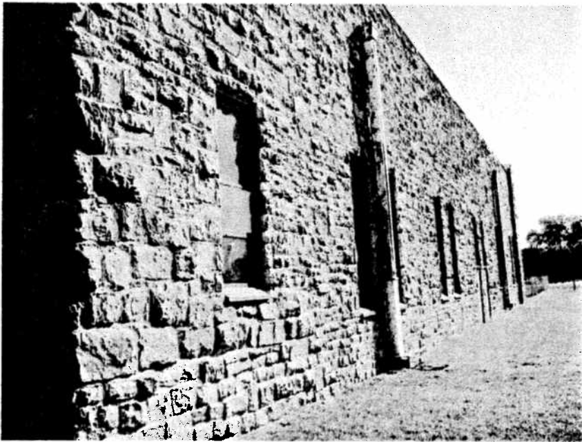
Figure 6: South side of armory facing east.
