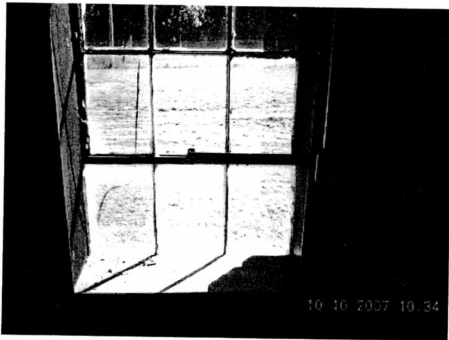
Figure 29. Window looking east from the office south of the kitchen area. Note the cracking and peeling paint typical of most of the Sulphur Armory windows.
