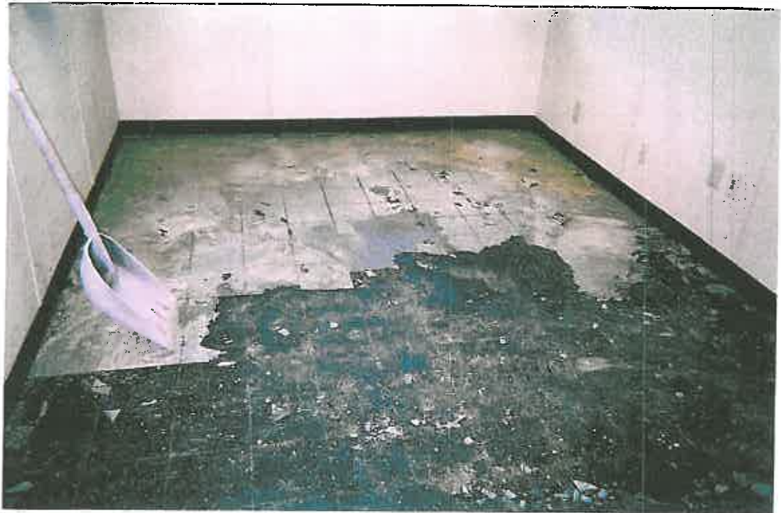
Abatement of floor tile and mastic
