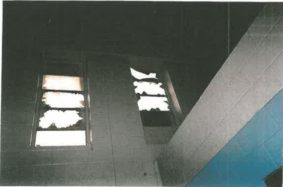
Inside window lintels - post abatement
