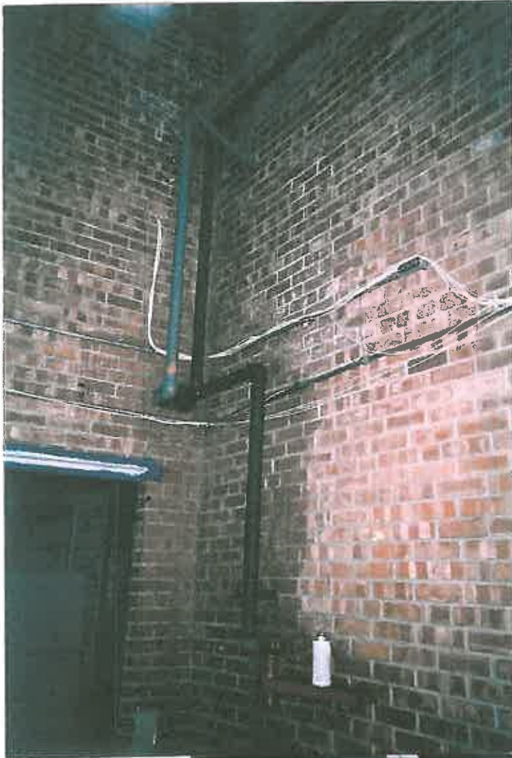
Post abatement of piping
