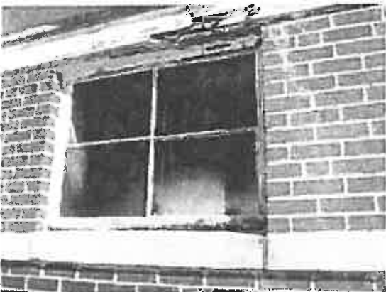
Photo #11: White painted highbay metal window frame and lintel and white painted wood fascia - LBP.
