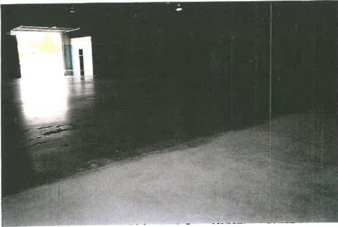
Floors after cleaning
