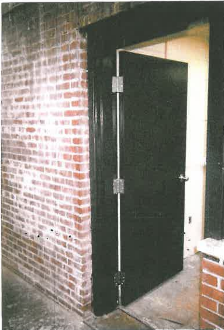
New door with butt hinges
