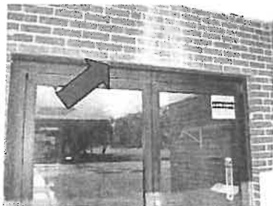
Photo #6: Red painted metal lintel - LBP.
