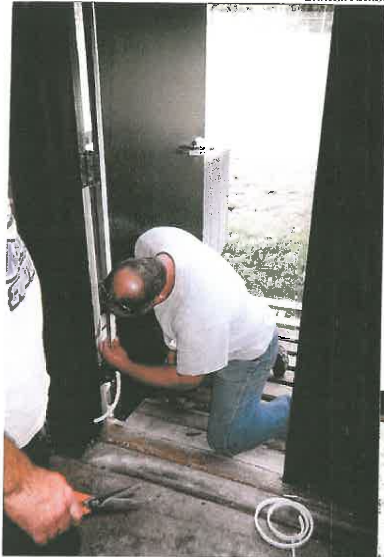
Install weather-strip on new doors
