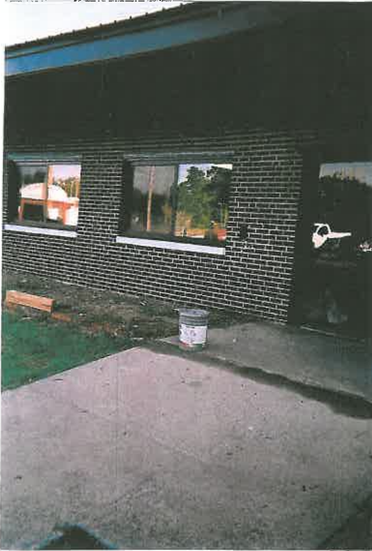
Exterior window lintels - post abatement
