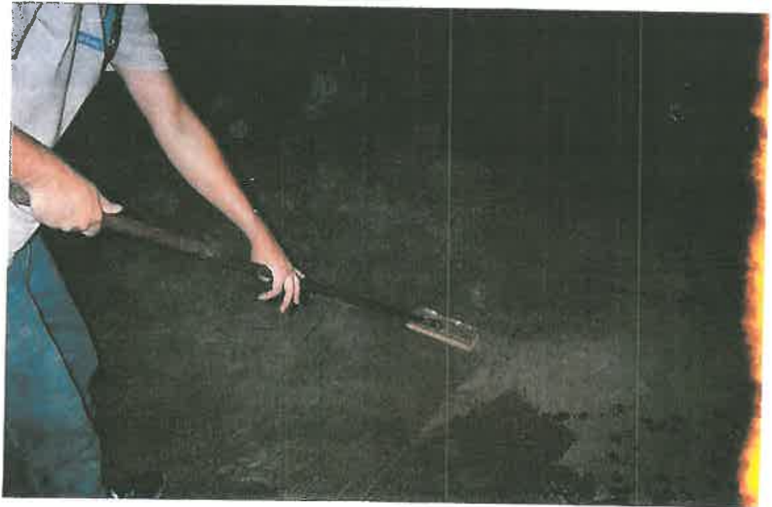
Post abatement of floor tile and mastic
