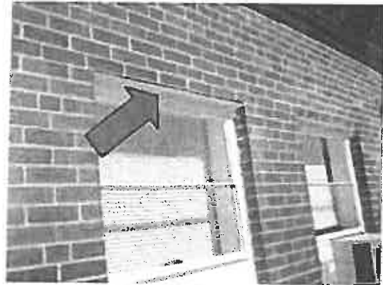
Photo #4: White painted metal window lintel - LBP.
