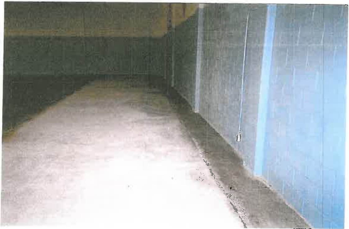
Floors after cleaning
