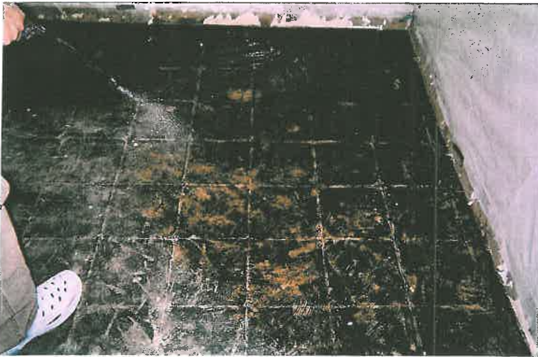
Abatement of floor tile and mastic
