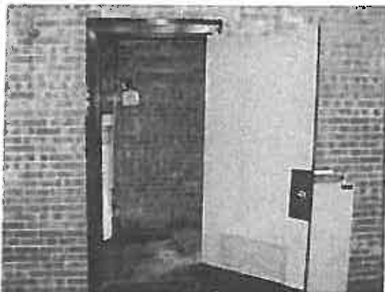
Photo #17: Yellow painted wood door Room 15 - LBP.
