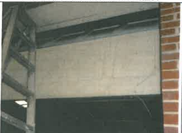
Photo #5: A roll-up door opening from Room 19 to Room 17 – LBP.
