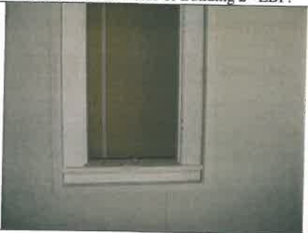
Photo #10: White pass through window in Room 10 –LBP.
