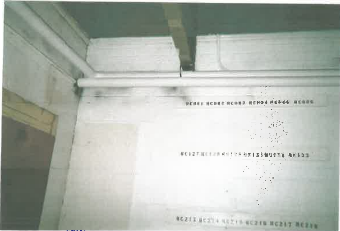
NEW INSULATION ON PIPING
