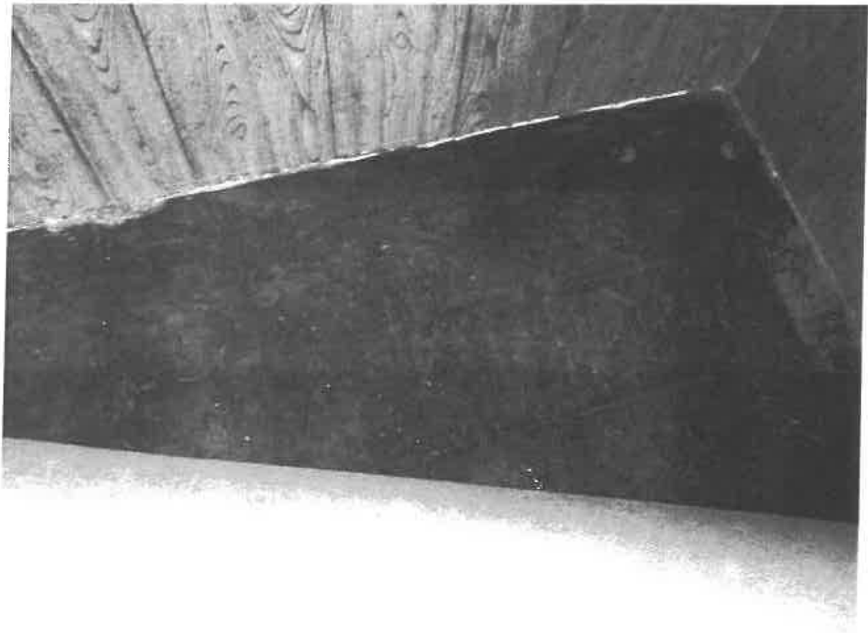
Black Mastic (Under Carpet) in Room 16 (Sample # SA-14A)
