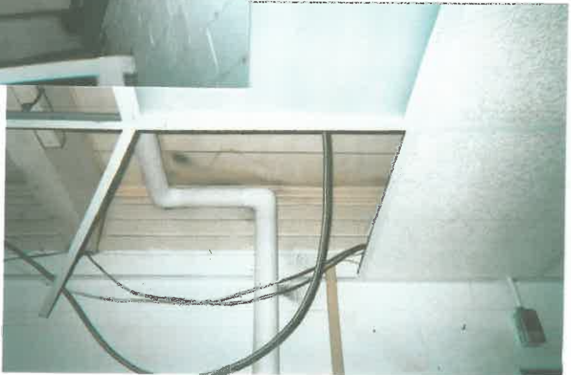
NEW INSULATION ON PIPING
