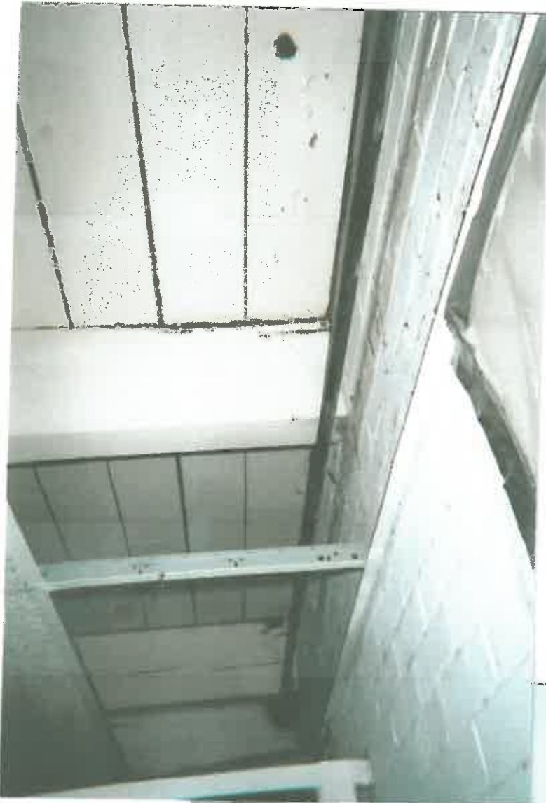
ABATED PIPE INSULATION
