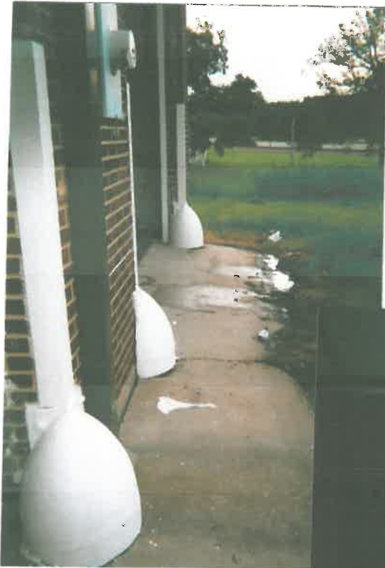
BOLLARDS - LOOSE AND PEELING PAINT REMOVED AND SEALED
