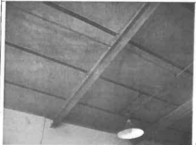
Reading 582, Room 2, Metal Ceiling Beams
