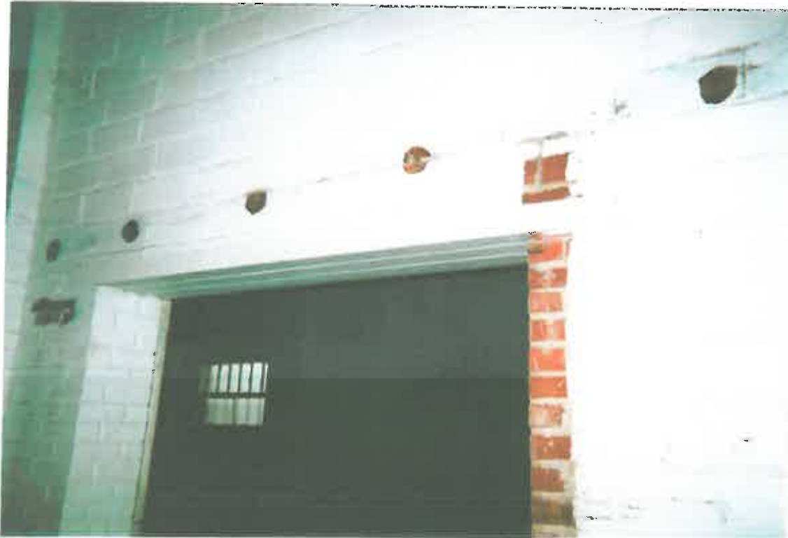
DOOR FRAME - LOOSE AND PEELING PAINT REMOVED AND RE-SEALED
