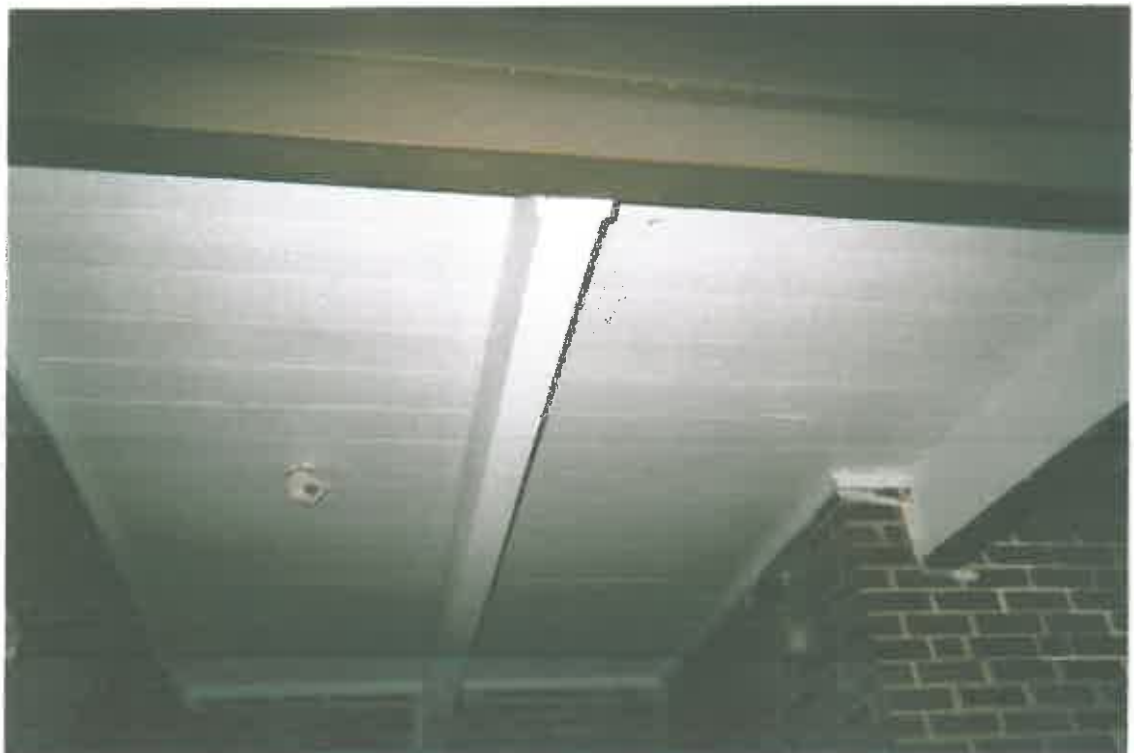
MAIN ENTRANCE - LOOSE AND PEELING PAINT REMOVED AND RE-SEALED
