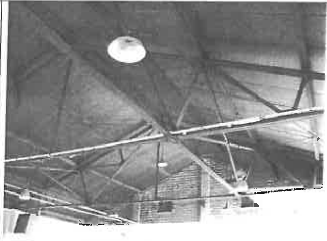
Reading 552, Room 1, Metal Ceiling Beams & Cross Members
