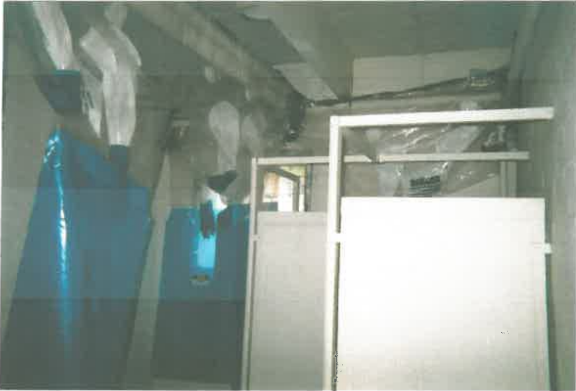
GLOVEBAGS ON ASBESTOS INSULATION
