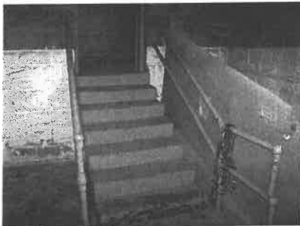
Photo: 3) Pre Lead Abatement
