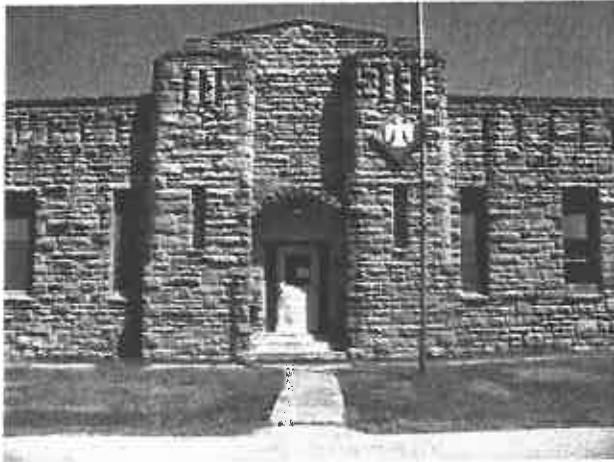
Photo: 1) Pre Lead Abatement
