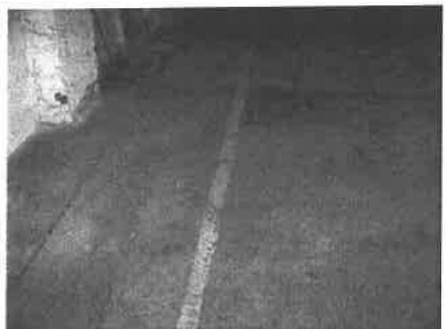
Photo: 6) Pre Lead Abatement
