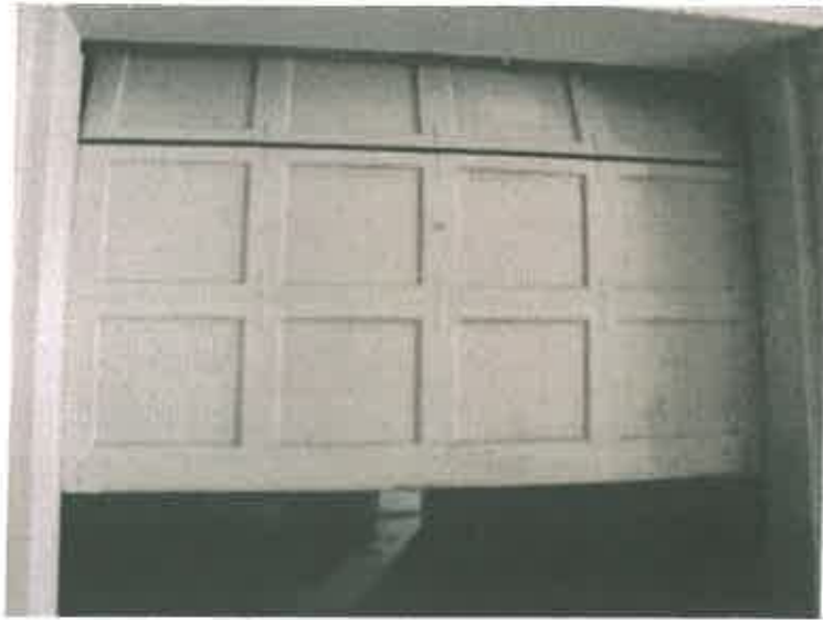
Figure 7. Overhead Door (# 41) (Opposite Side)
