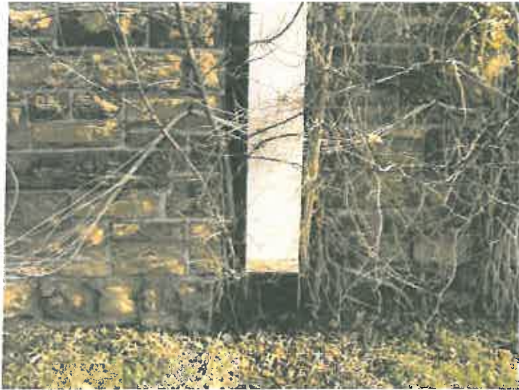
Figure 29. Roof Drain (Side C-2)
