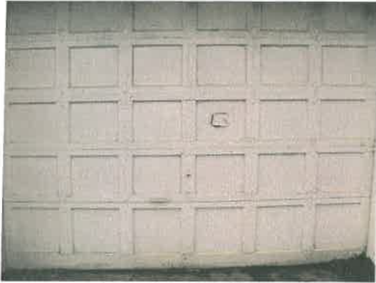
Figure 17. Garage Door (Side A-1, #1)
