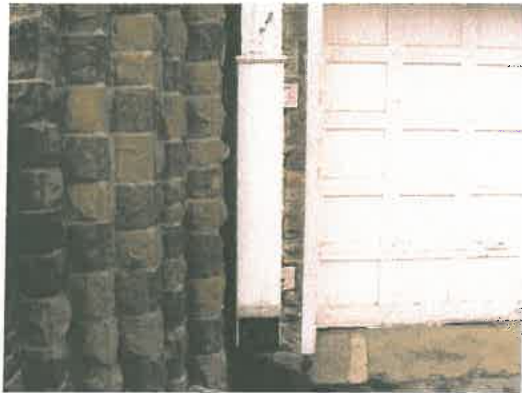
Figure 24. Roof Drain (Side A-1, #2)
