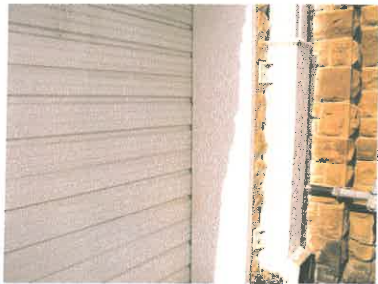
Figure 20. Garage Frame (Side A-3, #1)
