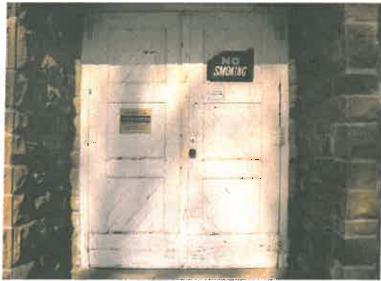
Figure 14. Exterior Door (Side B-2)
