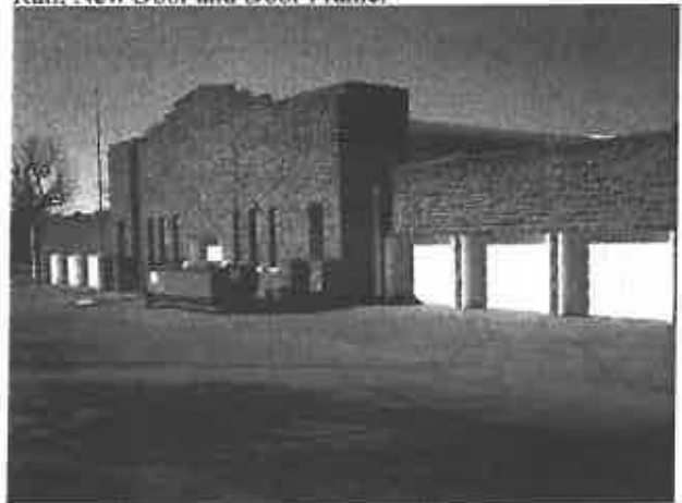
Photo: 18) Post Lead-Based Paint Exterior Abatement;
