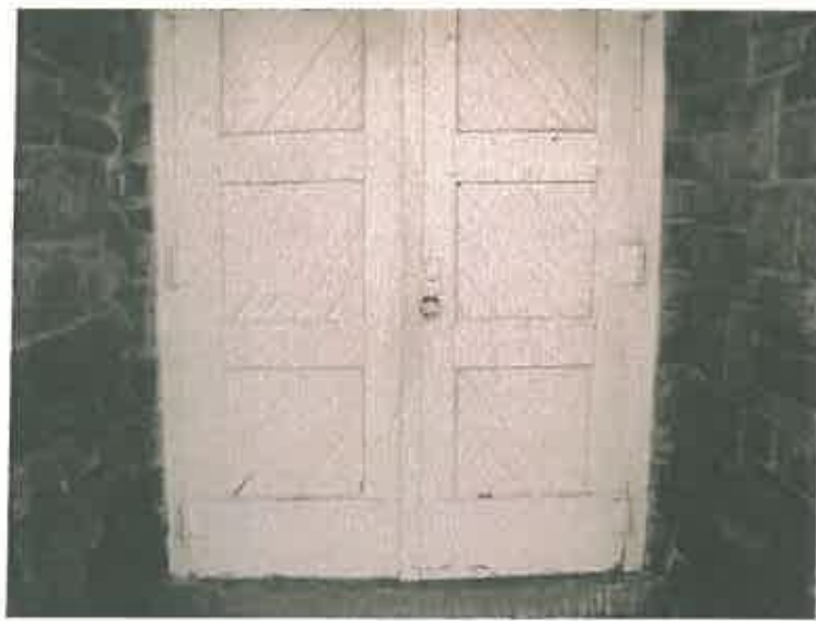
Figure 8. Exterior Door (Side D-2)
