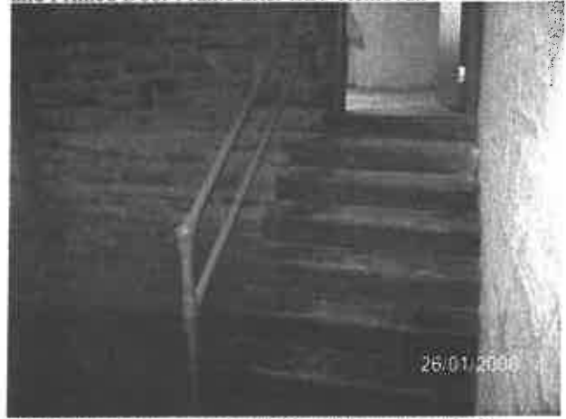
Photo: 16) Post Lead-Based Paint Abatement of Stair Rail, New Door and Door Frame.
