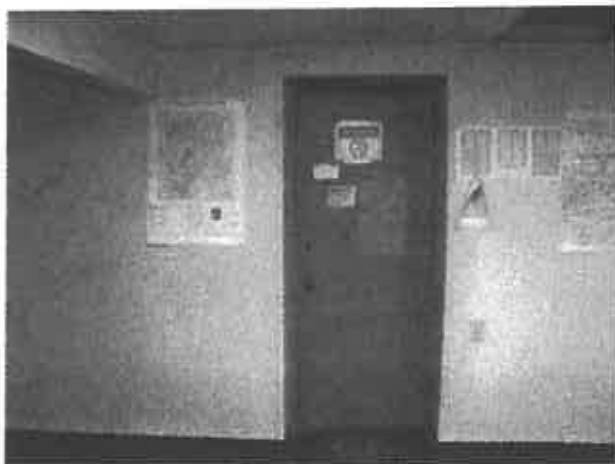
Photo: 5) Pre Lead Abatement
