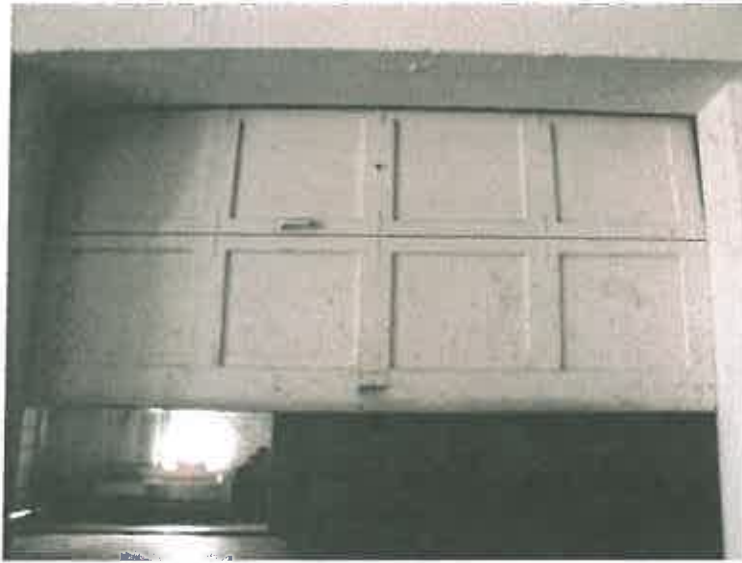
Figure 5. Overhead Door (# 12) (Opposite Side)
