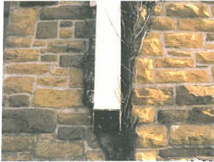
Figure 28. Roof Drain (Side C-1)
