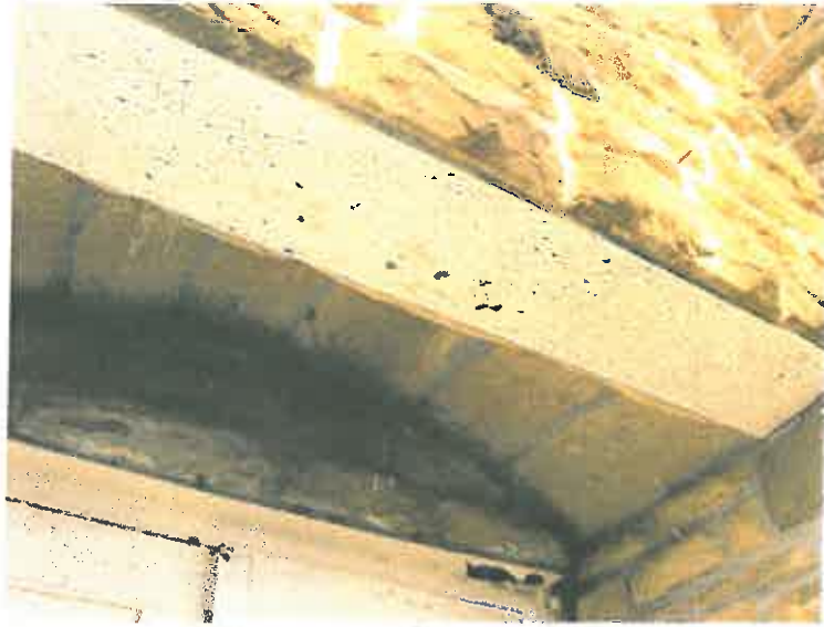
Figure 13. Doorway Overhang (Side B-2)
