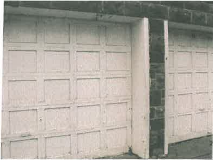
Figure 23. Garage Frame (Side A-1 #3)
