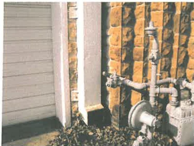
Figure 26. Roof Drain (Side A-3, #1)
