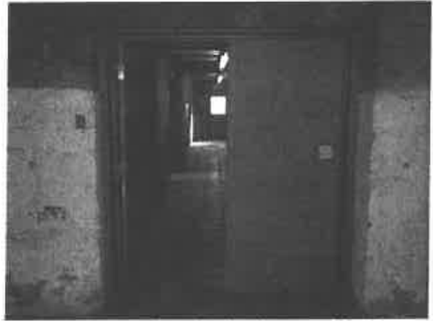
Photo: 14) Post Lead-Based Paint Abatement; New Door and Primed Door Frame after LBP Removal.
