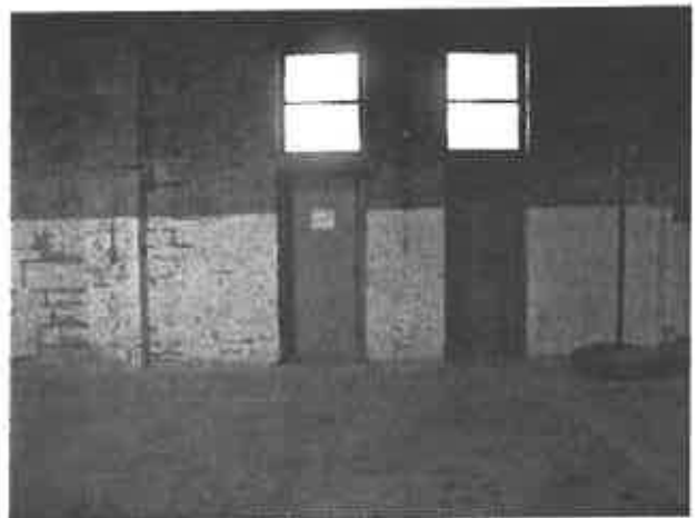
Photo: 4) Pre Lead Abatement
