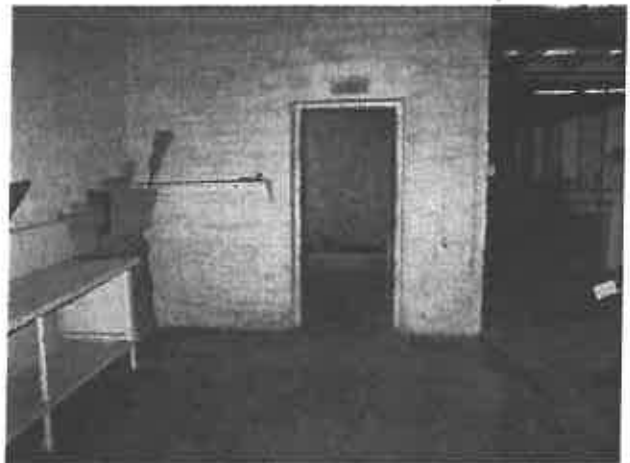
Photo: 6) Pre Lead Abatement
