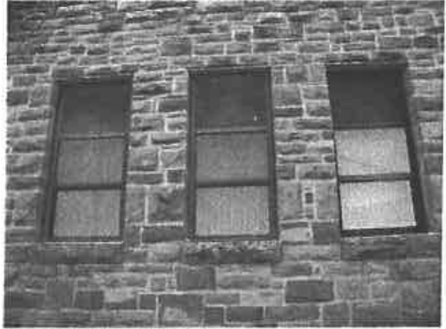
Photo: 2) Pre Lead Abatement
