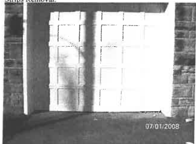
Photo: 12) Post Lead Abatement; Overhead Door and Jamb after LBP Encapsulated.
