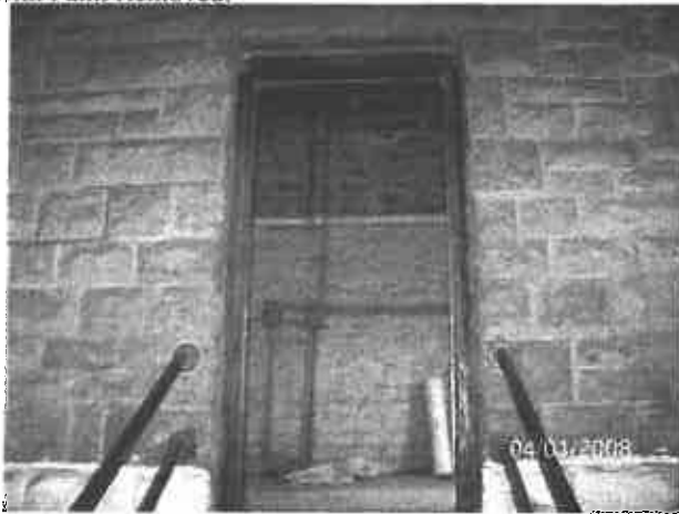
Photo: 9) Post Lead Abatement; Primed Door and Frame after LBP removal.
