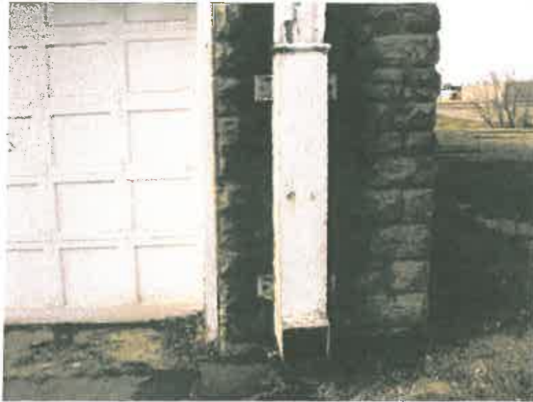
Figure 25. Roof Drain (Side A-1, #1)
