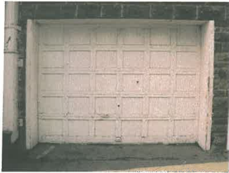
Figure 16. Garage Door (Side A-1, #3)
