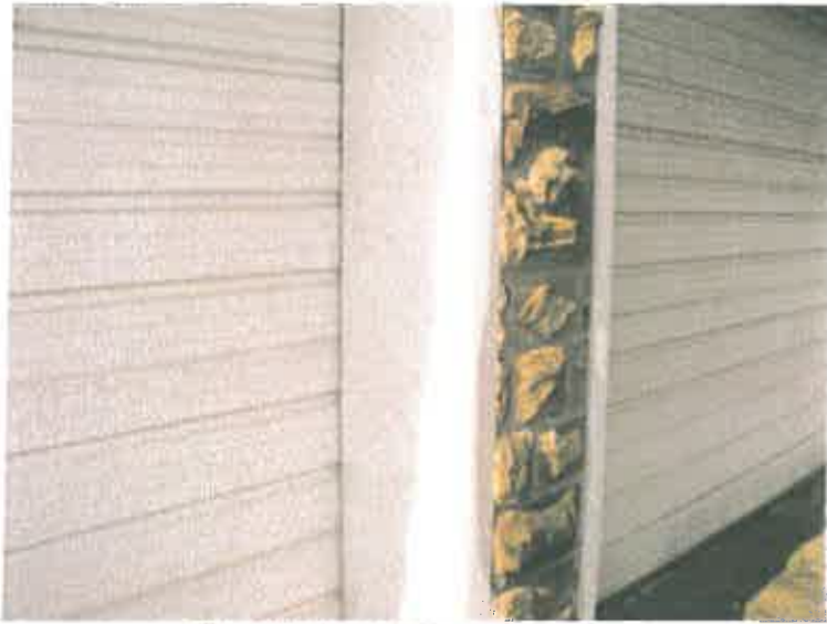
Figure 21. Garage Frame (Side A-3, #3)
