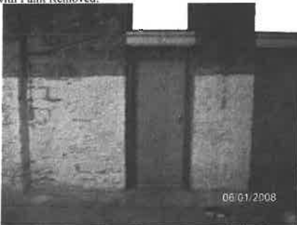
Photo: 9) Post Lead Abatement; New Door and Primed Frame after LBP removal.
