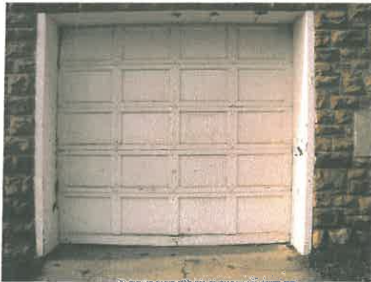
Figure 16. Garage Door (Side A2)
