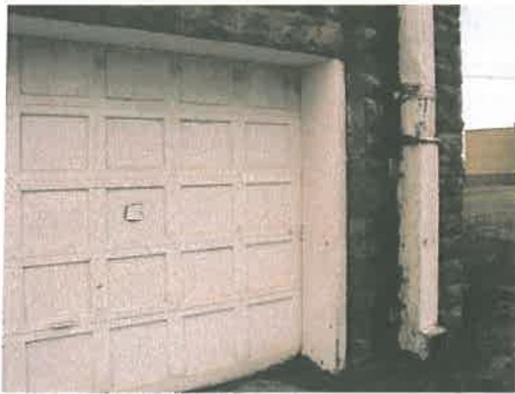
Figure 22. Garage Frame (Side A-1, #1)
