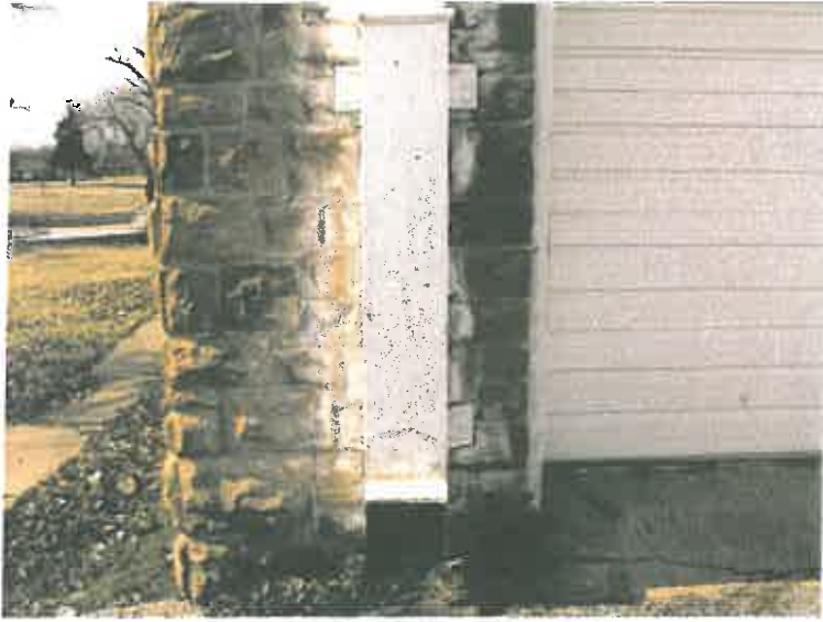
Figure 27. Roof Drain (Side A-3, #2)
