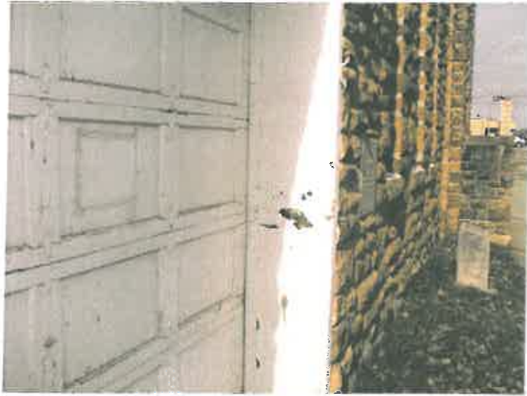
Figure 19. Garage Frame (Side A2)
