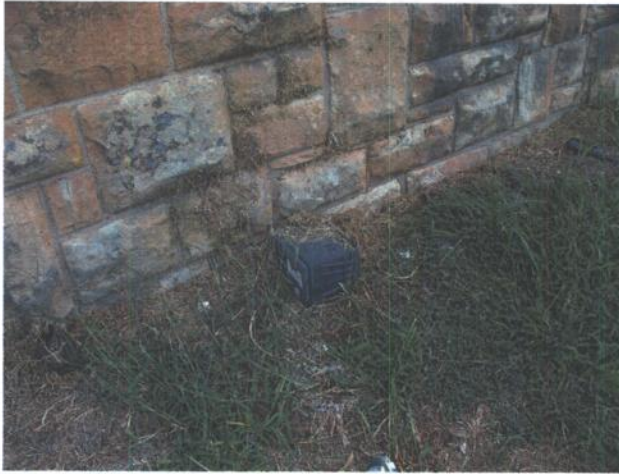
Photo #13: Car battery located on the west end of the armory building.
