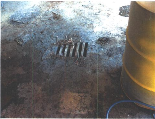
Photo #15: Drain in Drill Hall
