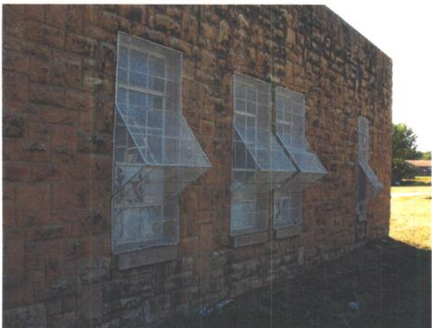
Photo #5: Outside wall of the west wing.
