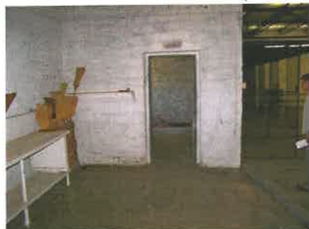
Photo: 6) Pre Lead Abatement
