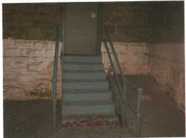
Photo: 14) Post Lead-Based Paint Abatement of Stair Rail, New Door and Door Frame.
