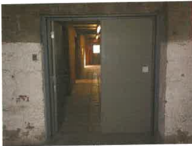
Photo: 13) Post Lead-Based Paint Abatement. New Door and Primed Door Frame after LBP Removal.
