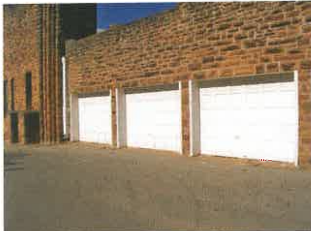
Photo: 3) Pre Lead Abatement
