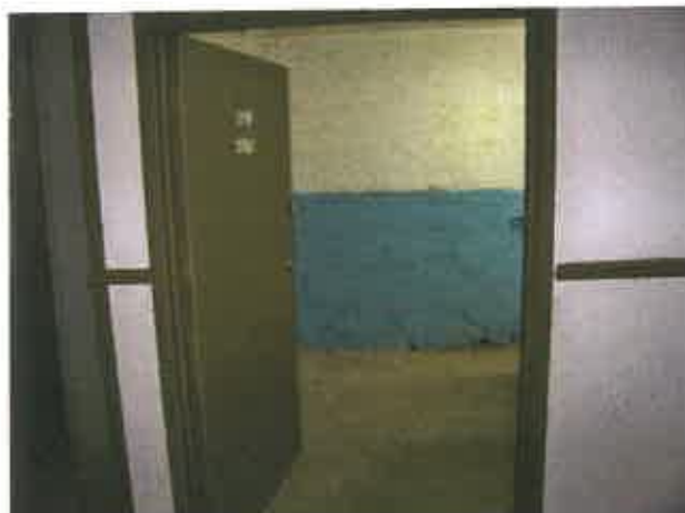
Photo: 5) Pre Lead Abatement
