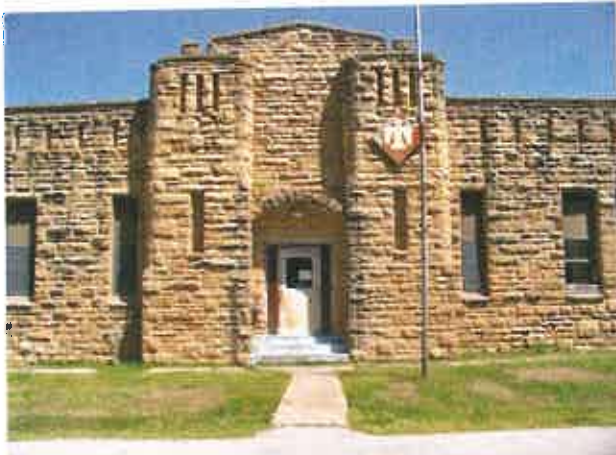
Photo: 1) Pre Lead Abatement
