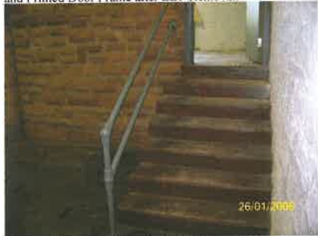
Photo: 16) Post Lead-Based Paint Abatement of Stair Rail, New Door and Door Frame.
