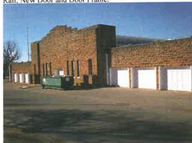
Photo: 18) Post Lead-Based Paint Exterior Abatement;
