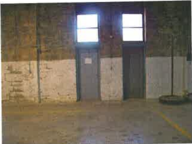
Photo: 4) Pre Lead Abatement
