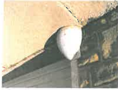
White Metal Roof Drain - Side C #1
