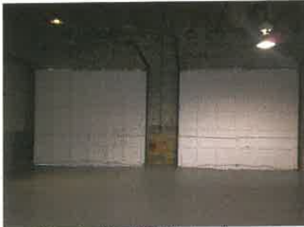
Photo: 13) Post Lead-Based Paint Abatement.
