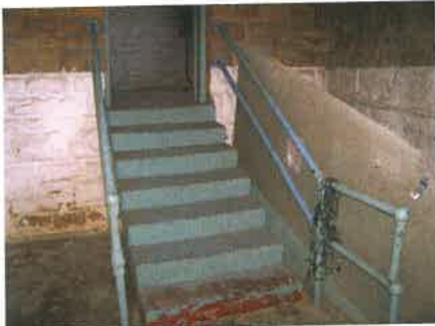
Photo: 3) Pre Lead Abatement
