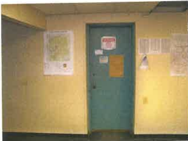
Photo: 5) Pre Lead Abatement
