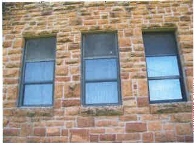
Photo: 2) Pre Lead Abatement
