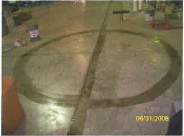
Photo: 10) Post Lead Abatement; Floor Sealed after LBP Strips Removal.
