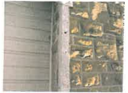
White Metal Roof Drain - Side C #2
