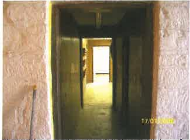
Photo: 8) Post Lead Abatement; Lead-Based Paint Door Frame with Paint Removed.
