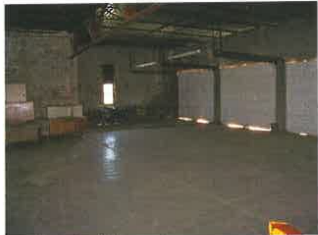
Photo: 4) Pre Lead Abatement
