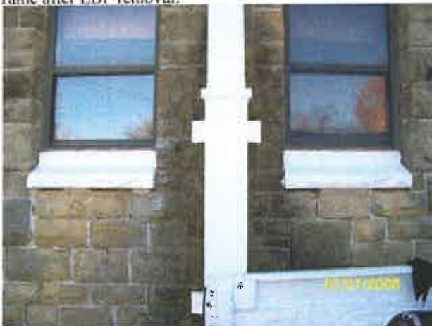
Photo: 11) Post Lead Abatement; Downspout and Window Sill Sealed with Approved Encapsulant.
