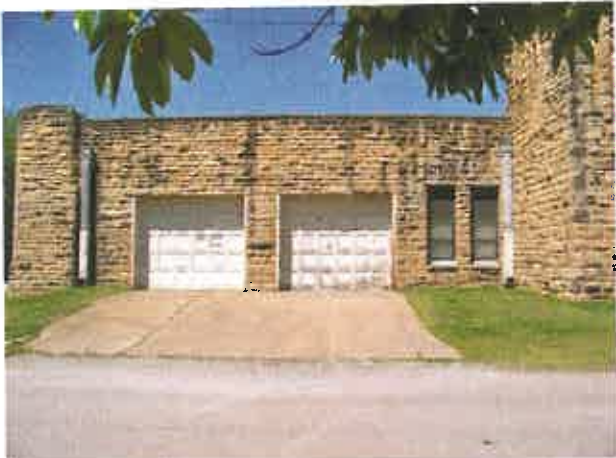
Photo: 2) Pre Lead Abatement
