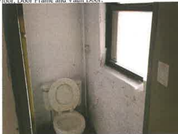
Photo: 17) Post Lead Abatement; Primed Door Frame after LBP Removal and Encapsulated Walls.
