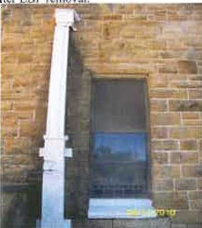
Photo: 11) Post Lead Abatement; Downspout and Window Sill Sealed with Approved Encapsulant.
