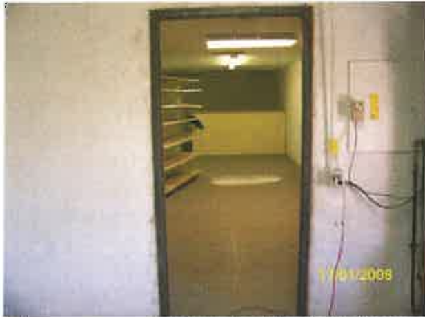
Photo: 7) Post Lead Abatement; Lead-Based Paint Frame with Paint Removed.
