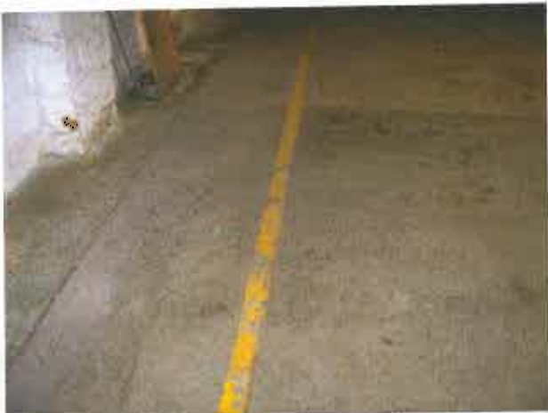
Photo: 6) Pre Lead Abatement
