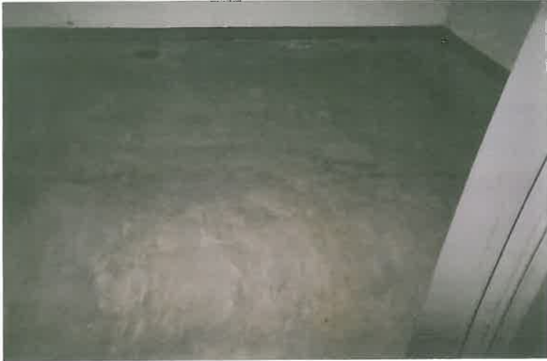
CLASSROOM AFTER FLOOR TILE AND MASTIC REMOVAL
