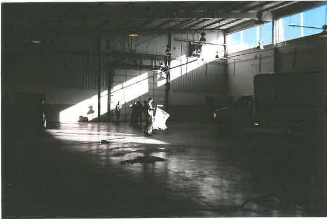
DRILL FLOOR CLEANING
