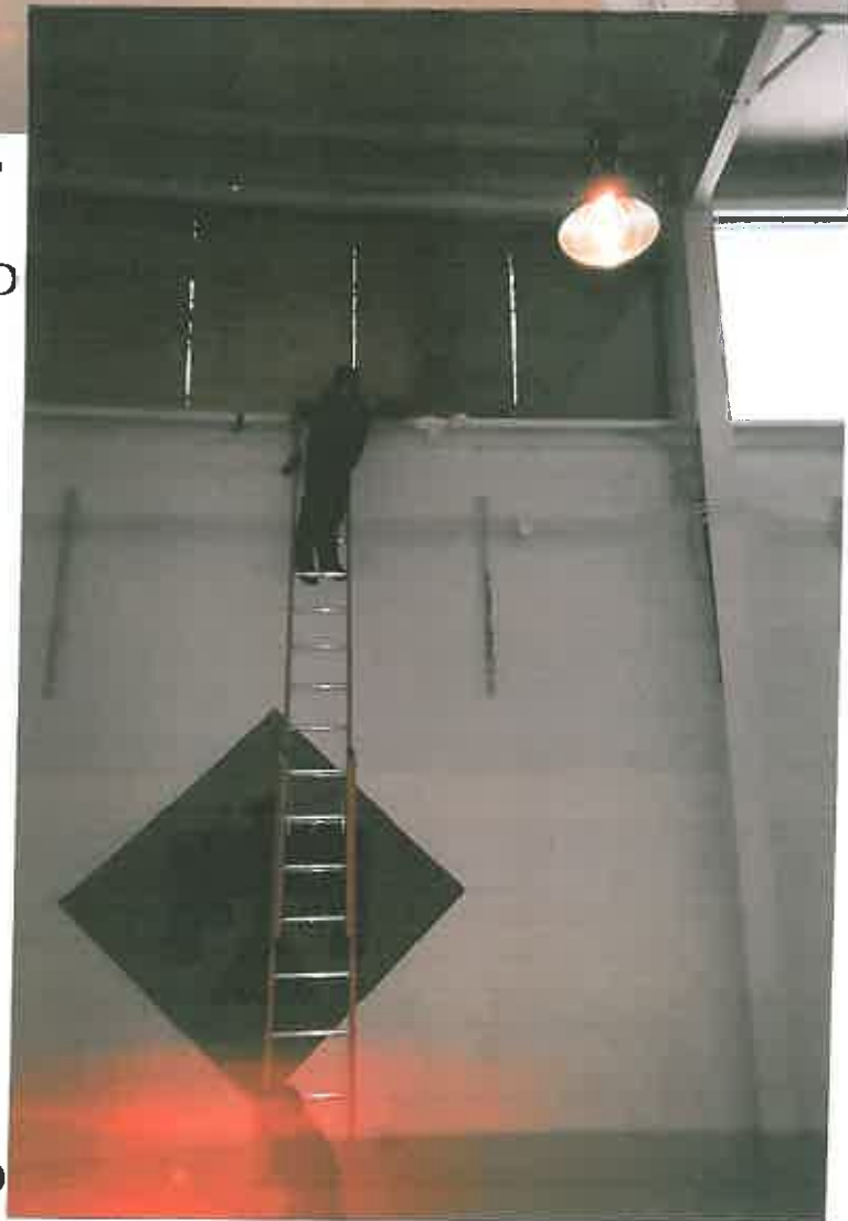
DRILL FLOOR WINDOW SEATS WIPED AND VACUUMED
