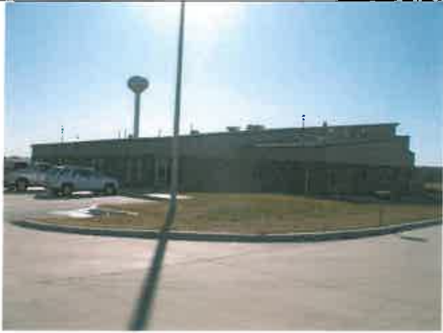
Former Okemah Armory
