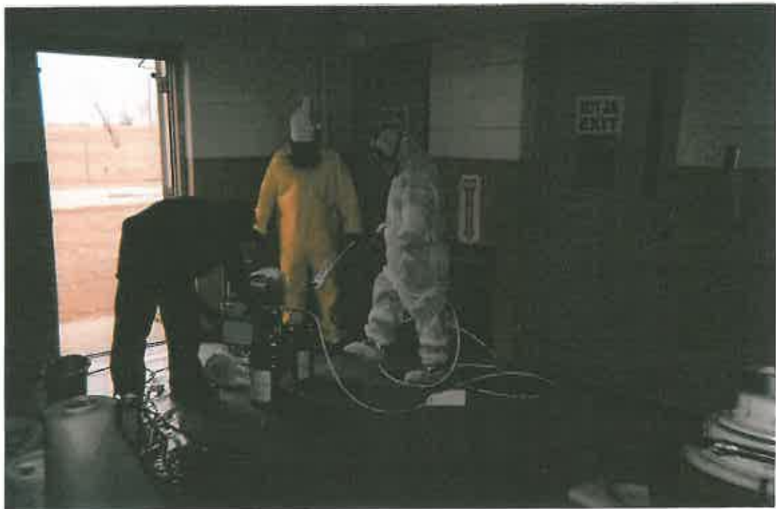
STAGING AREA FOR FIRING RANGE CLEANING
