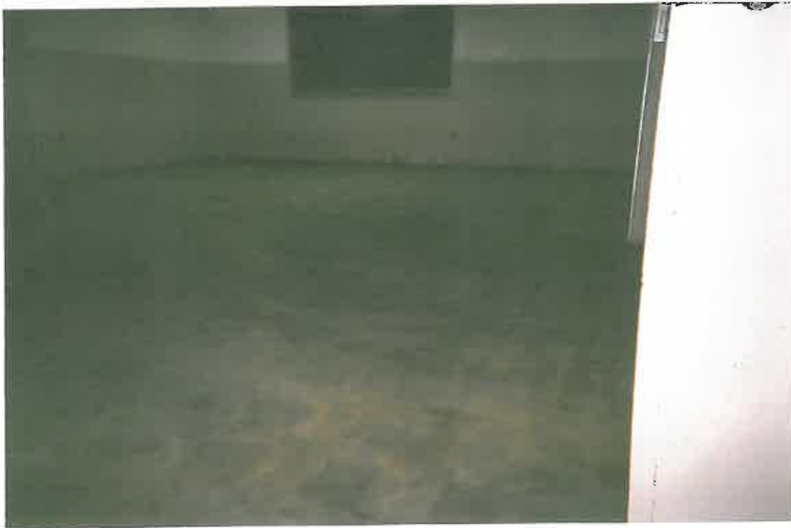
CLASSROOM AFTER FLOOR TILE AND MASTIC REMOVAL
