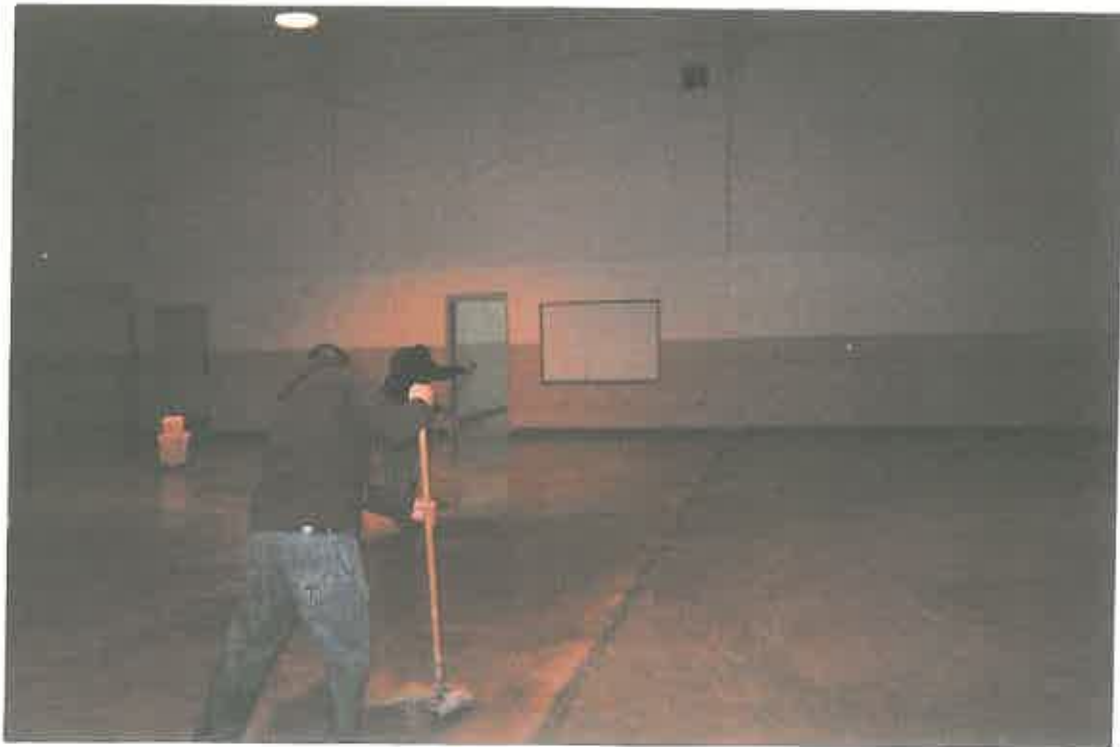
DRILL FLOOR FINAL CLEAN
