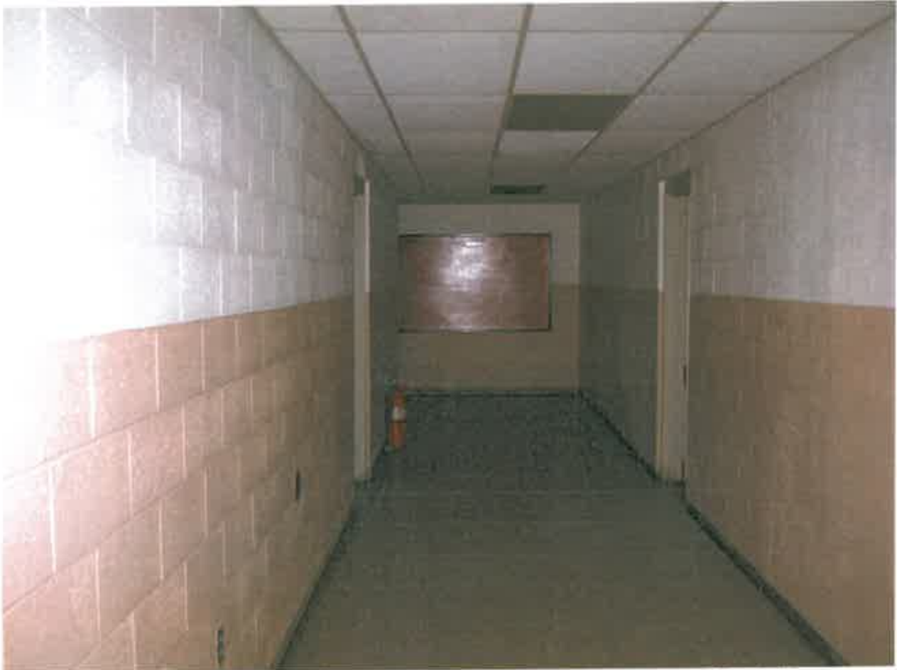
Non-Friable Asbestos Containing Mastic on Non-Asbestos Brown Floor Tile (Sample # OK-04A)
