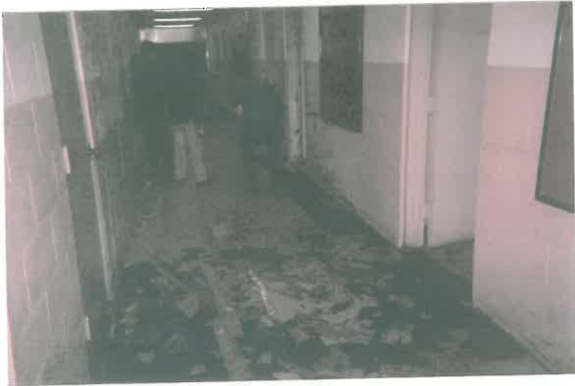
FLOOR TILE REMOVAL
