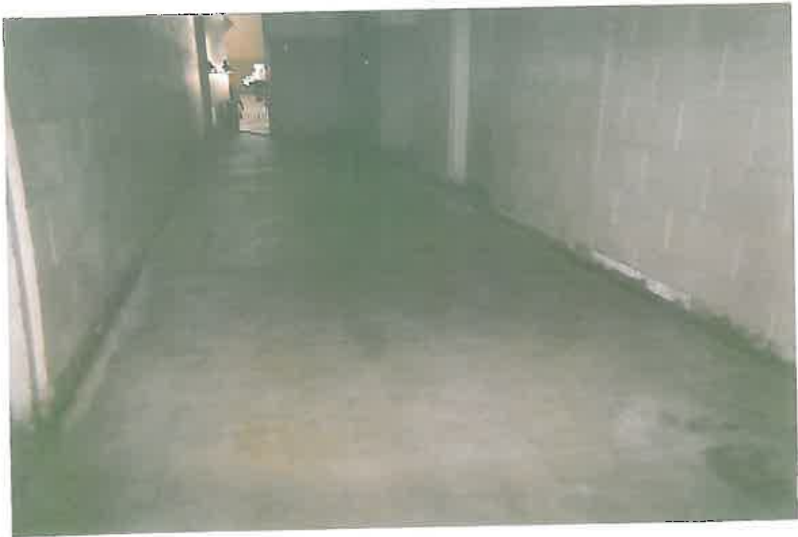
HALLWAY AFTER REMOVAL
