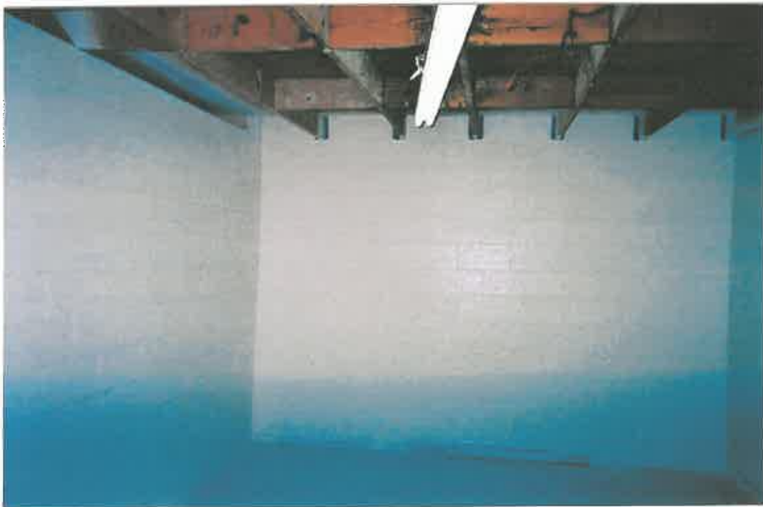
Removal of loose and peeling paint - wall
