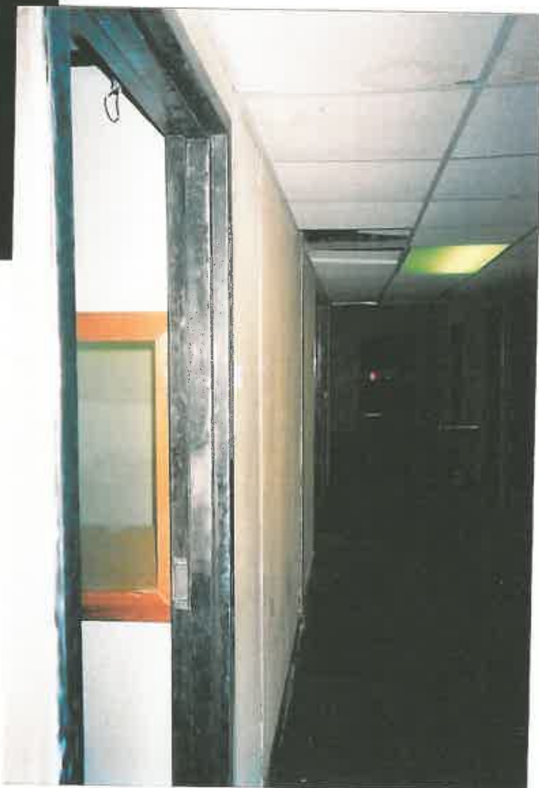
Door frame after abatement and sealed
