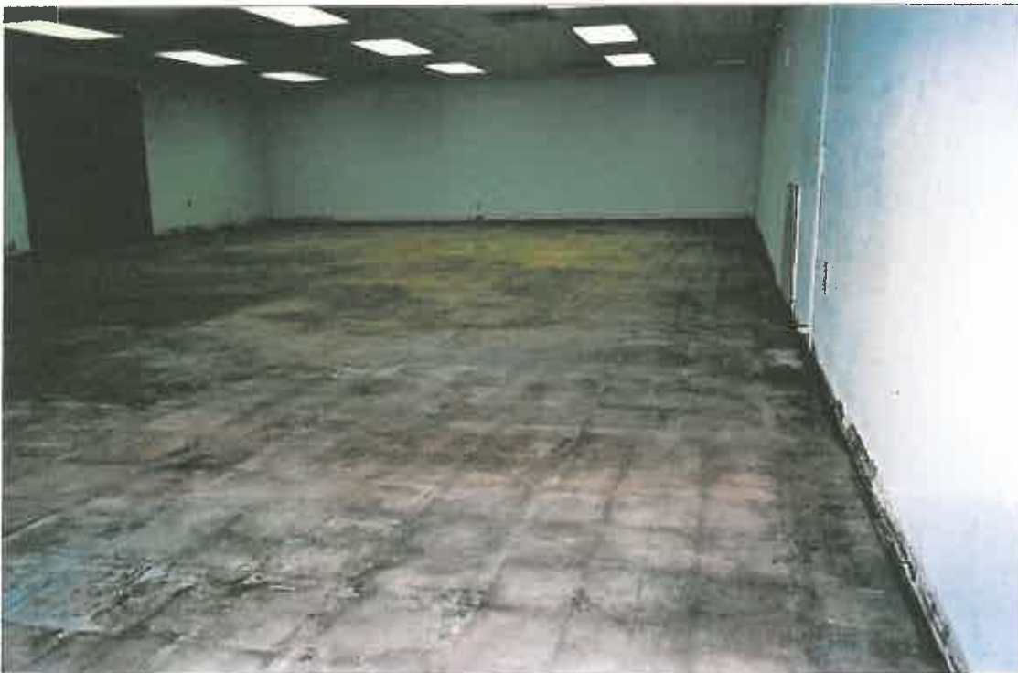
Floor tile removed
