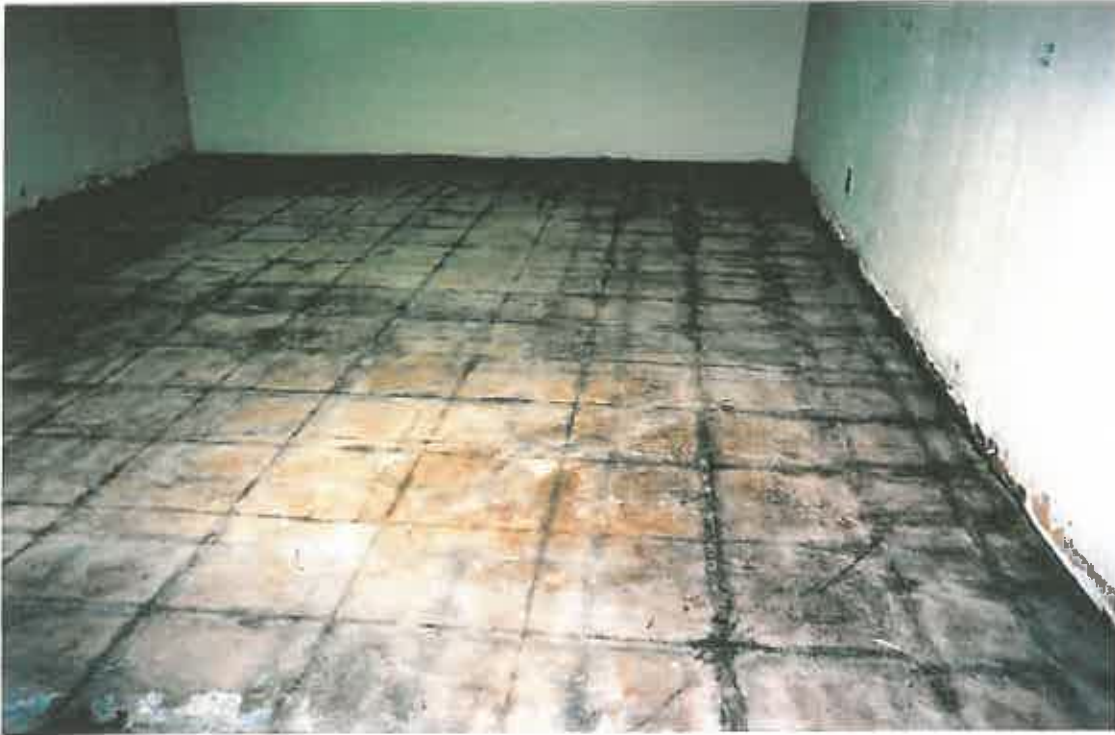
Floor tile and mastic removed
