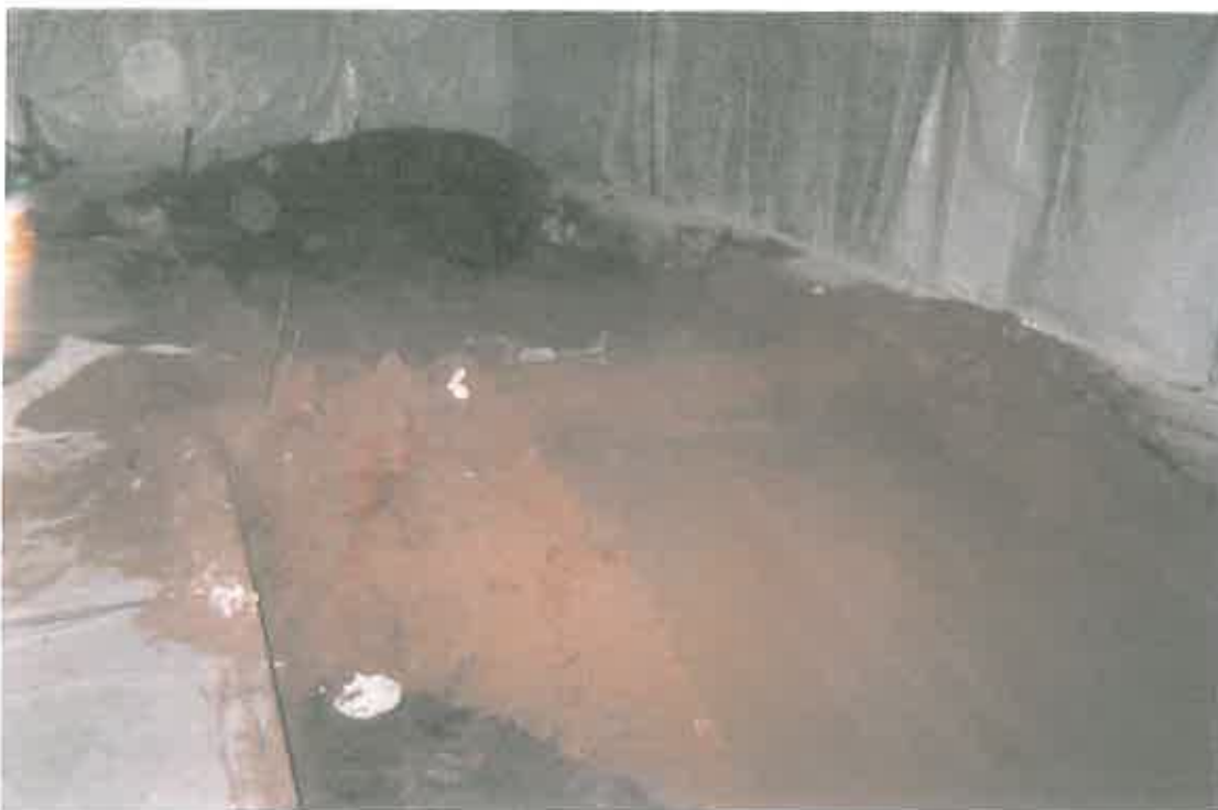
Sand pit removal
