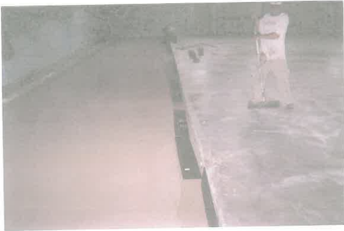
Clean sand and expansion joint
