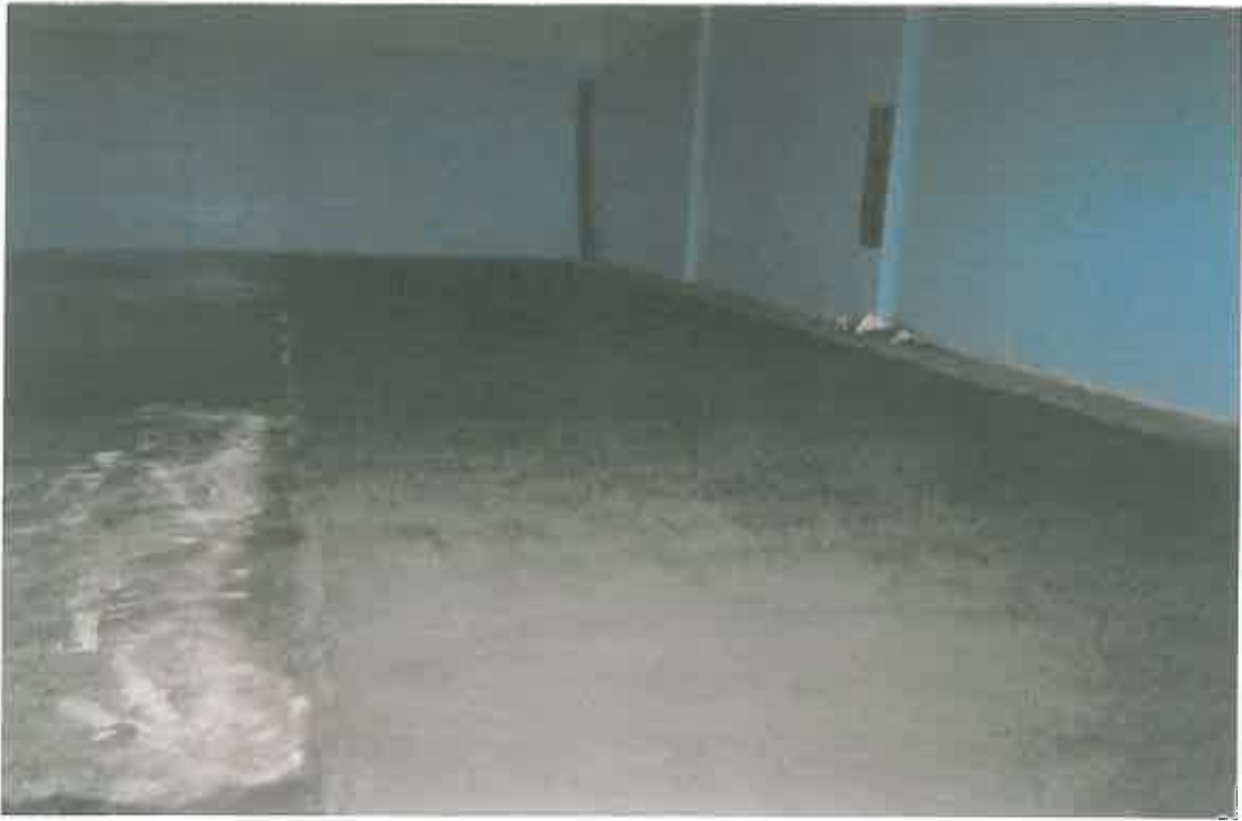
New concrete cap - final
