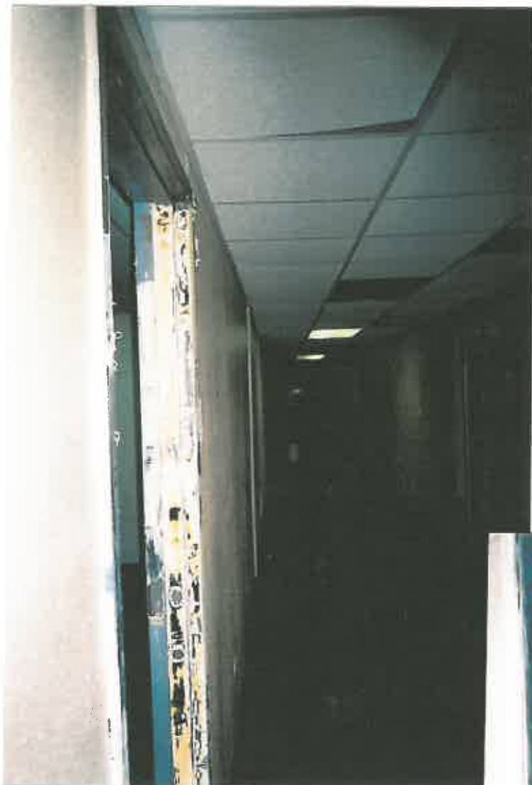
Door frame LBP removed
