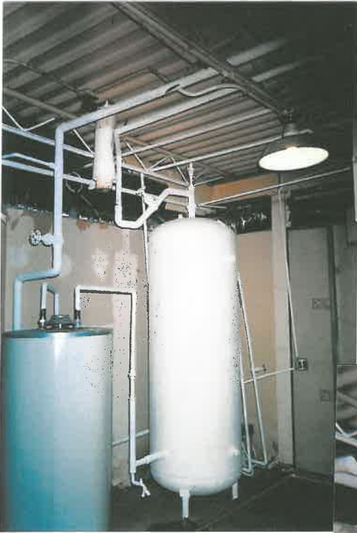
Water tank - abated
