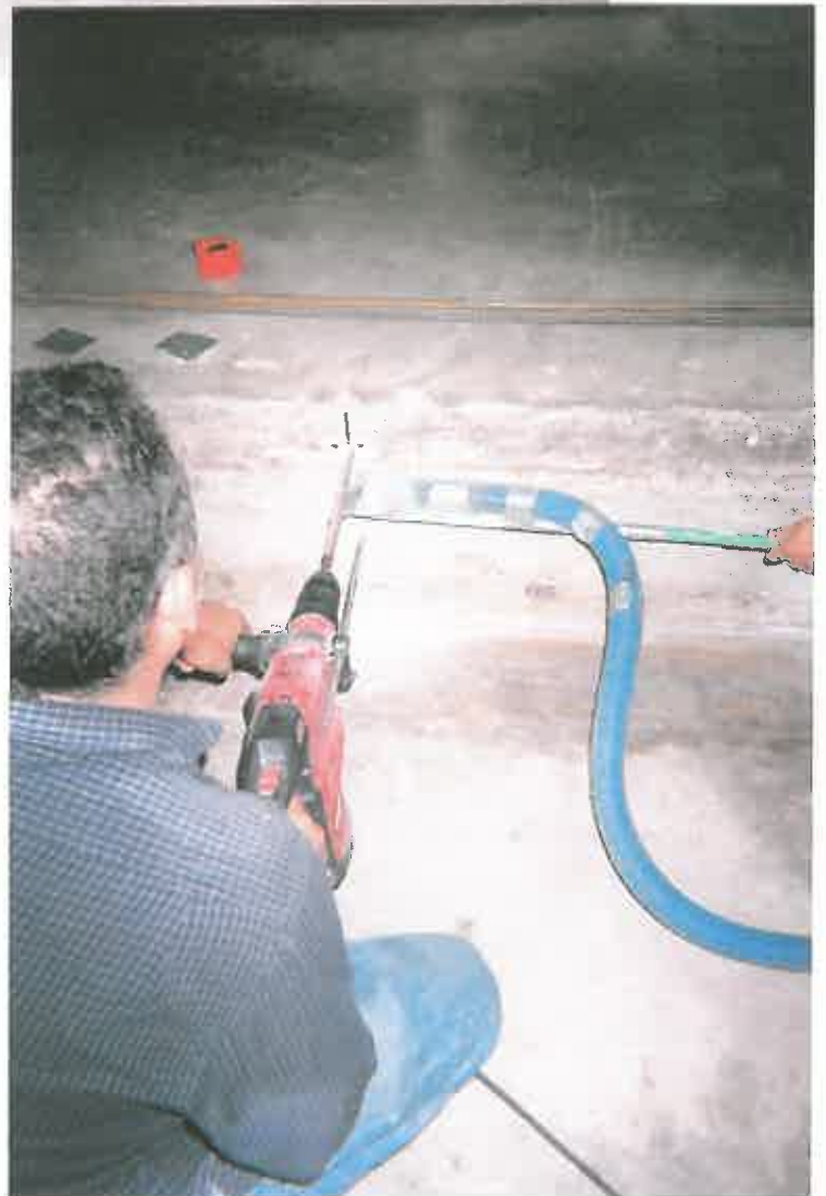
New concrete prep work
