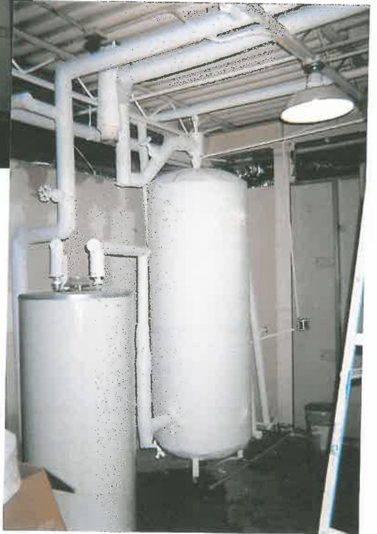
Water tank - reinsulated
