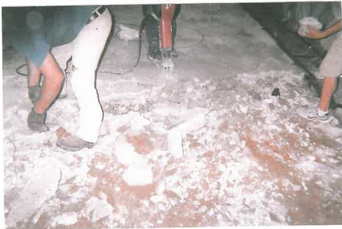
Concrete layer of sand pit
