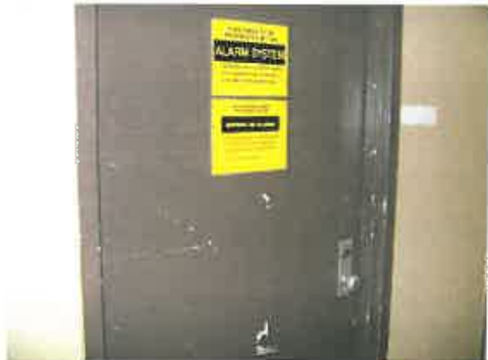
Photo # 4: Typical brown door and door frame - LBP.
