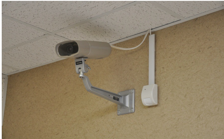
Figure 4-9 Example of a VMD camera
