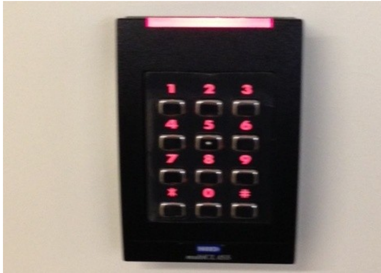
Figure 4-3 Card reader with associated PIN pad
