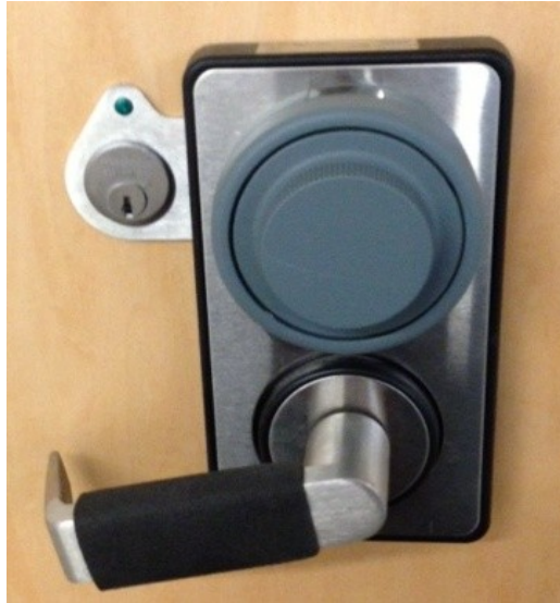
Figure 4-1 Combination door lock with bypass key lock
