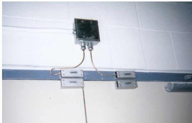
Figure 4-5 Triple-biased BMS sensor on double doors
