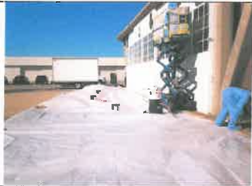
Hanger door during LBP abatement.
