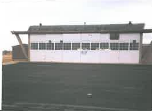
North hanger door pre-abatement.
