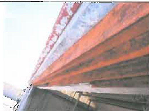
Hanger door tracks after paint is removed.
