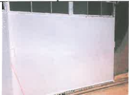
Exterior hanger door with LBP paint encapsulated.
