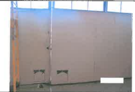
Interior hanger door with new insulation and wood panels.
