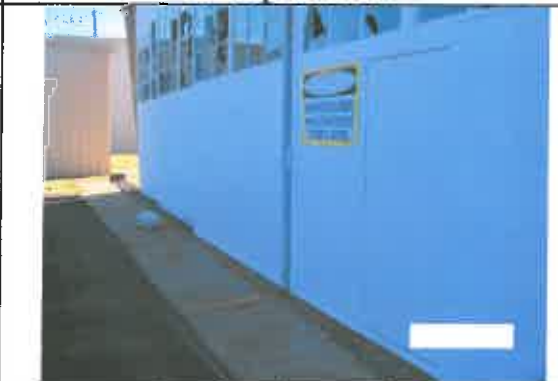
Exterior hanger door with LBP paint encapsulated.
