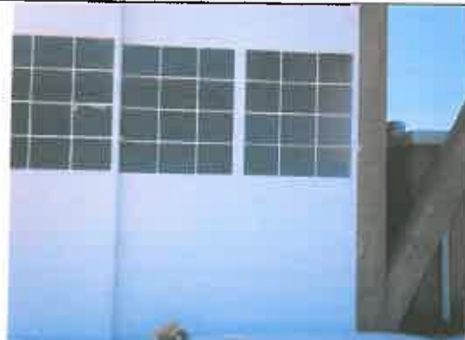
North hanger door post abatement.
