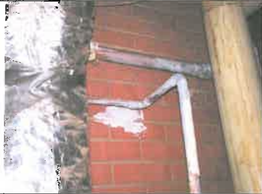
Asbestos removal complete and inspected by ODOL.
