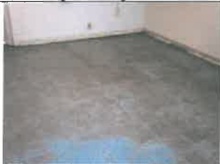
Concrete floor after asbestos mastic removed.
