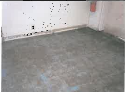
Concrete floor after asbestos mastic removed.
