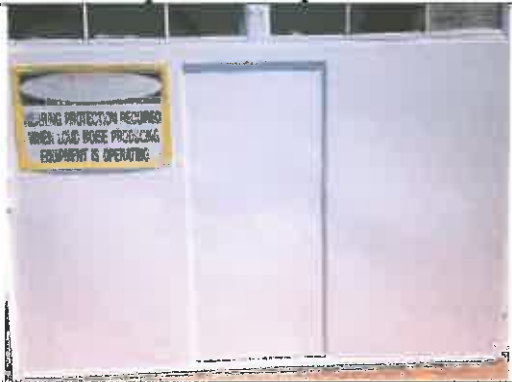
Exterior hanger door with LBP paint encapsulated.
