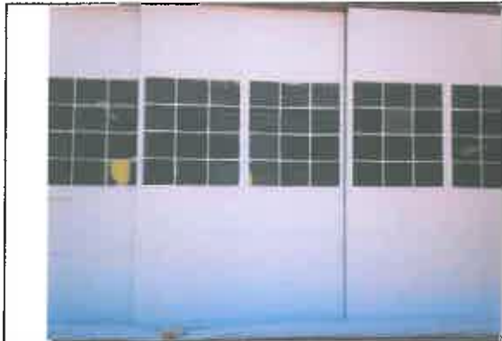
Exterior hanger door with LBP paint encapsulated.
