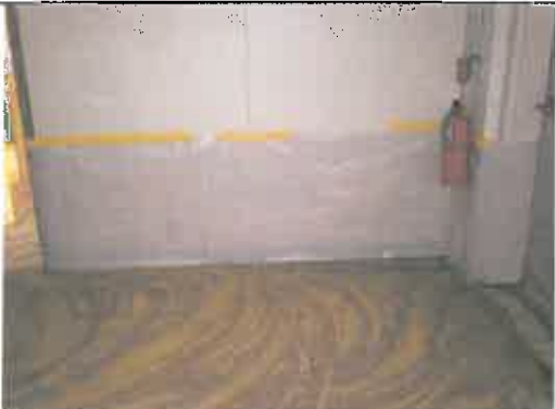
Asbestos mastic prepped for removal.
