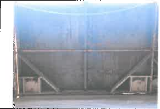
Interior hanger door during LBP abatement
