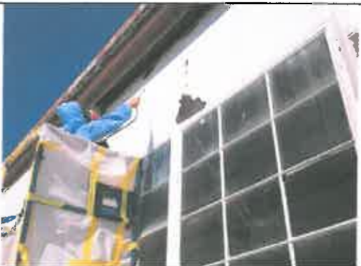
Hanger door during LBP abatement.
