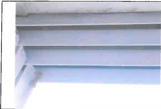
Hanger door tracks after LBP abatement.
