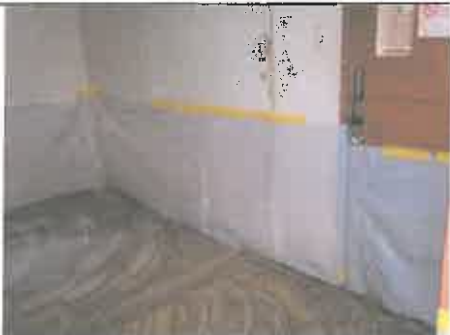
Asbestos mastic prepped for removal.
