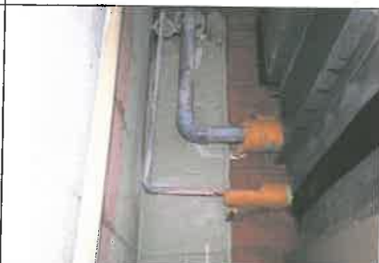
Asbestos removal complete and inspected by ODOL.
