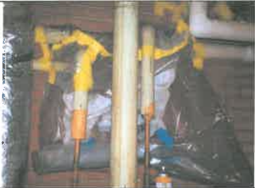
. Asbestos pipe fittings prepared for removal
