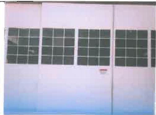
Hanger door after LBP abatement.
