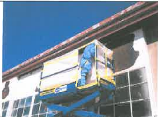
Hanger door during LBP abatement.
