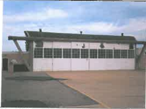
South hanger door pre-abatement.
