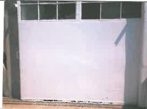
South hanger door post abatement.
