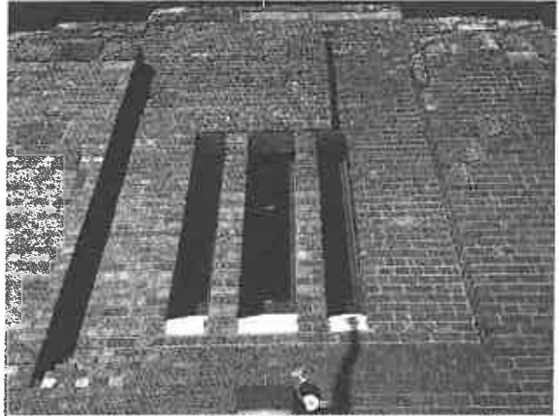
Photo: 14) Post Lead-Based Paint Abatement; Exterior Window Sills and Lintels.
