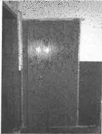
Photo: 9) Post Lead Abatement; Primed Door and Frame after LBP removal.
