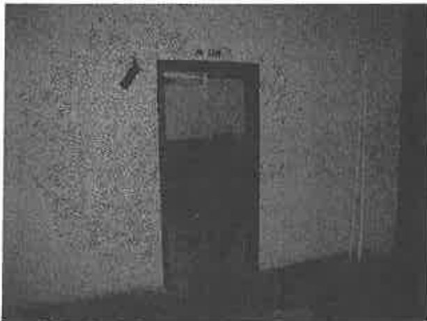
Photo: 3) Pre Lead Abatement
