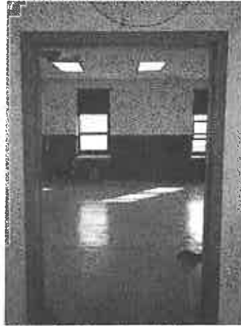
Photo: 10) Post Lead Abatement; Primed door Frame after LBP Removal.
