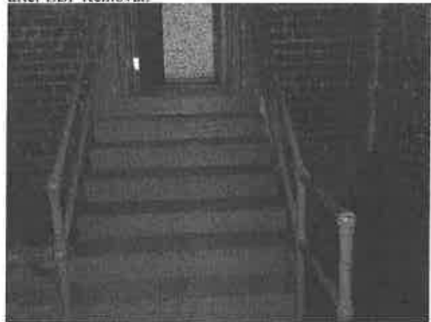
Photo: 12) Post Lead Abatement; Primed Stair Rails and Door Frame after LBP Removal.
