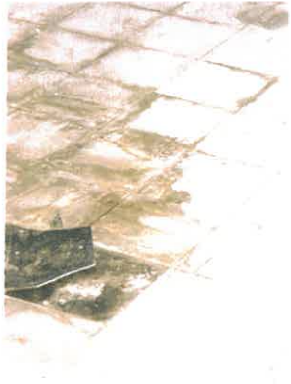
9x9 Floor Tile and Mastic in Room 4
