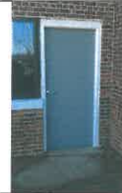
LBP door replaced.
