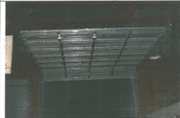
New OH door and track.
