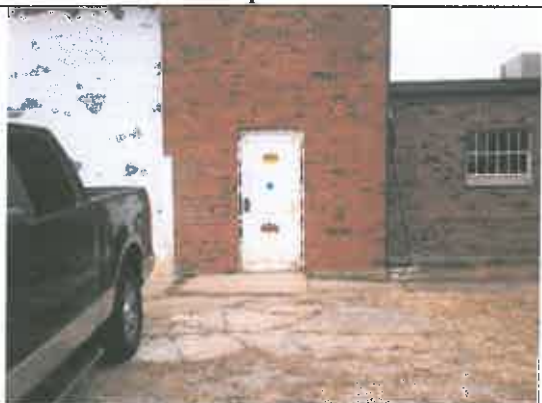
Replace LBP window, OH door, door and frame.
