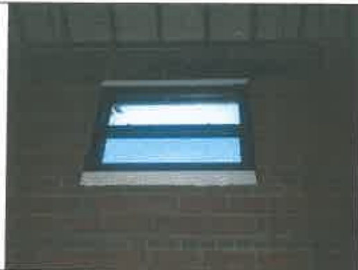
New window with encapsulated sill and lintel.
