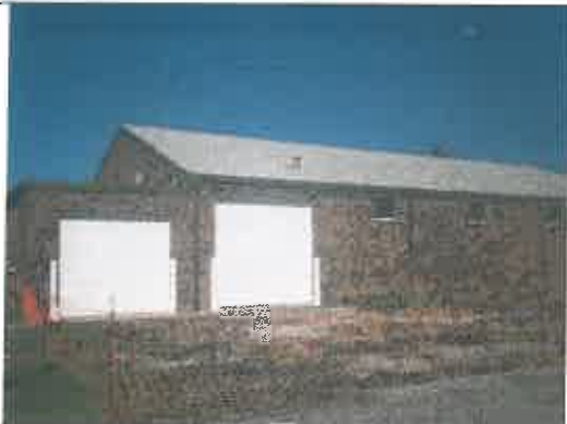
LBP OH doors, frames and guard post wet scraped and encapsulated.
