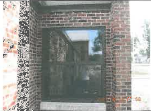
New window with encapsulated sill and lintel.
