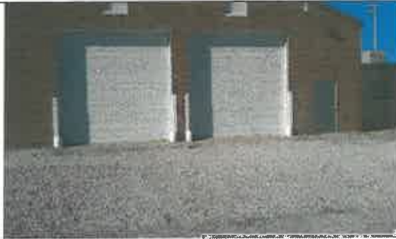
Wet scrape and encapsulate black LBP on brick.
