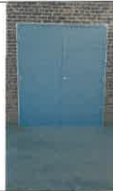
New door and frame.
