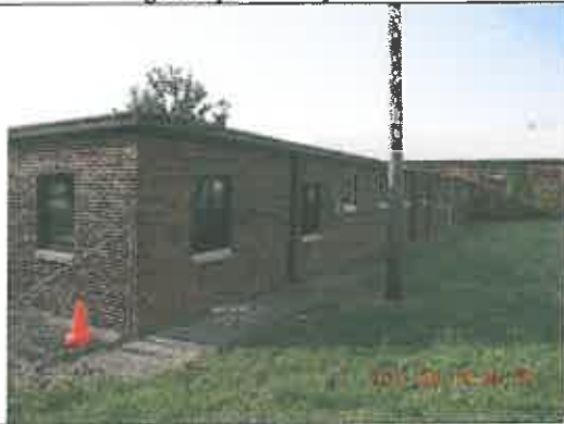
New windows with encapsulated window sills and lintels.
