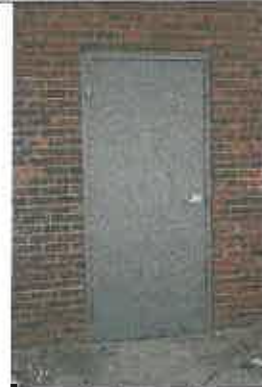
New walk door and frame.
