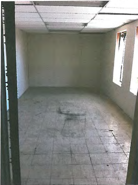
Asbestos-Containing Floor Tile
