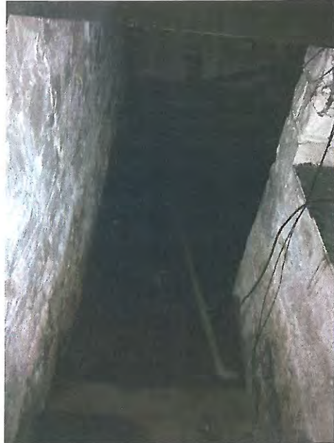
Flooded Indoor Firing Range
