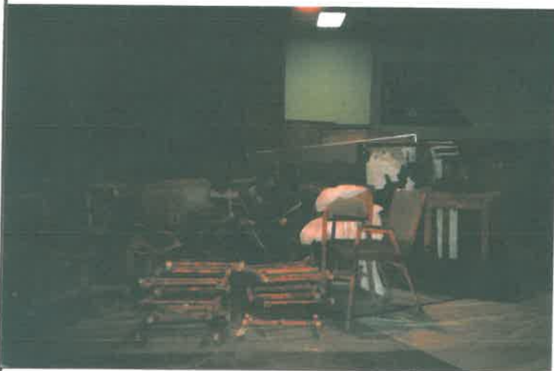
Bldg 1 - Non-lead contaminated trash on drill floor.
