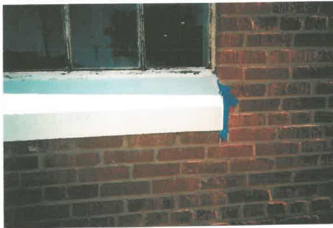
Window sill after abatement and encapsulation.
