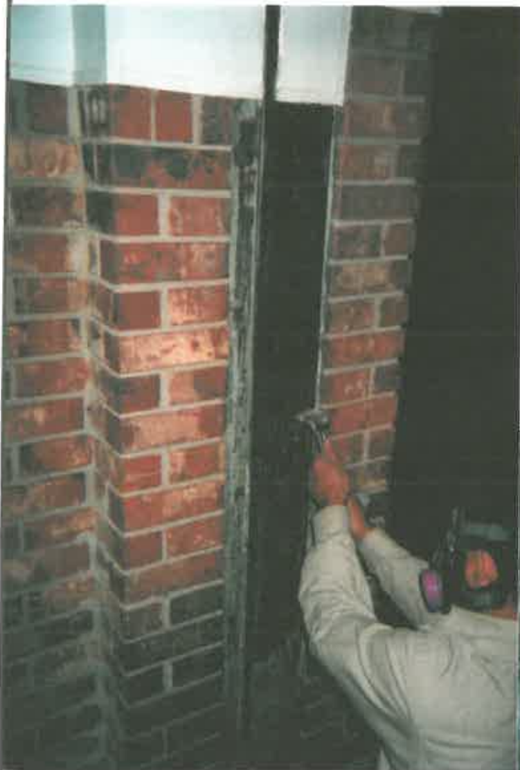
Door frame during abatement process.
