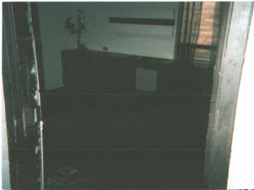
BLDG 7 - Door frame and room.
