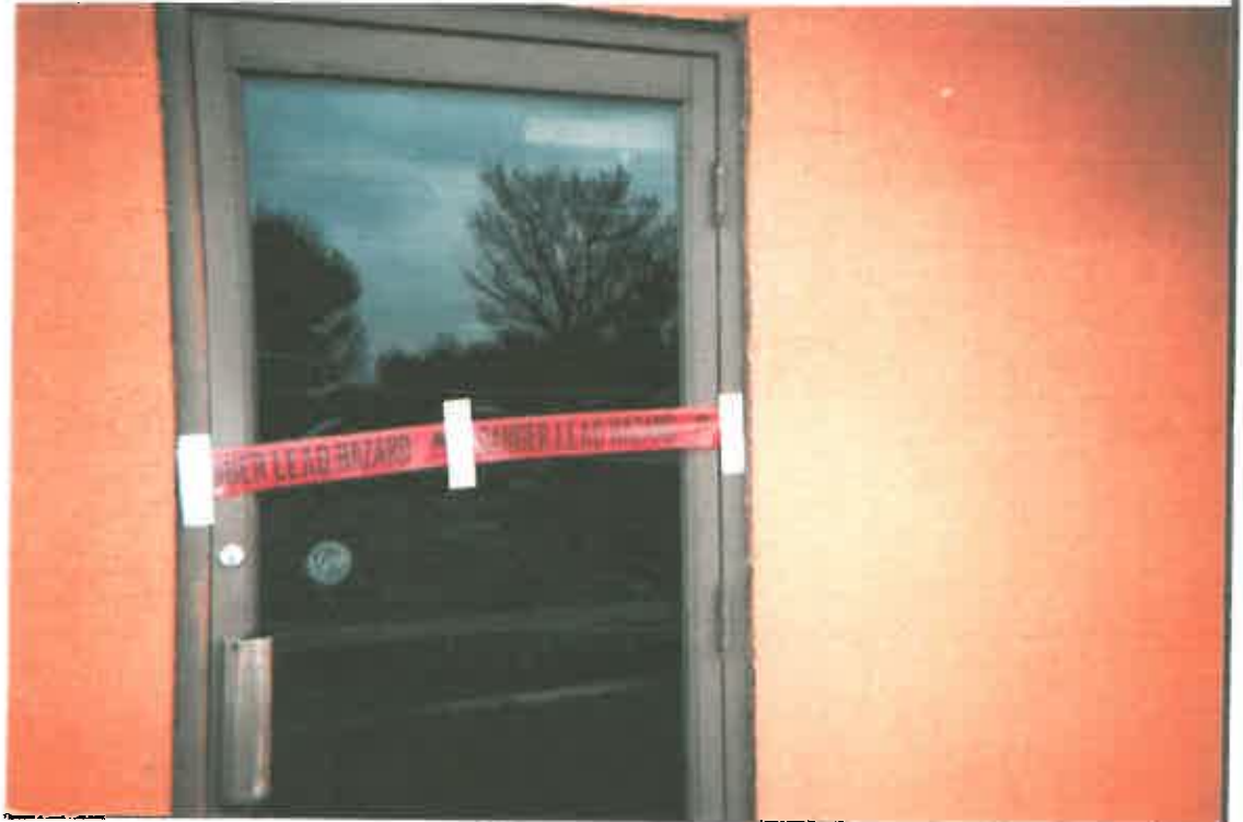
Bldg 7 - Entry door secured.
