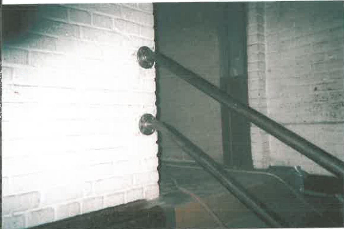
Stairway railing after abatement and before encapsulation.
