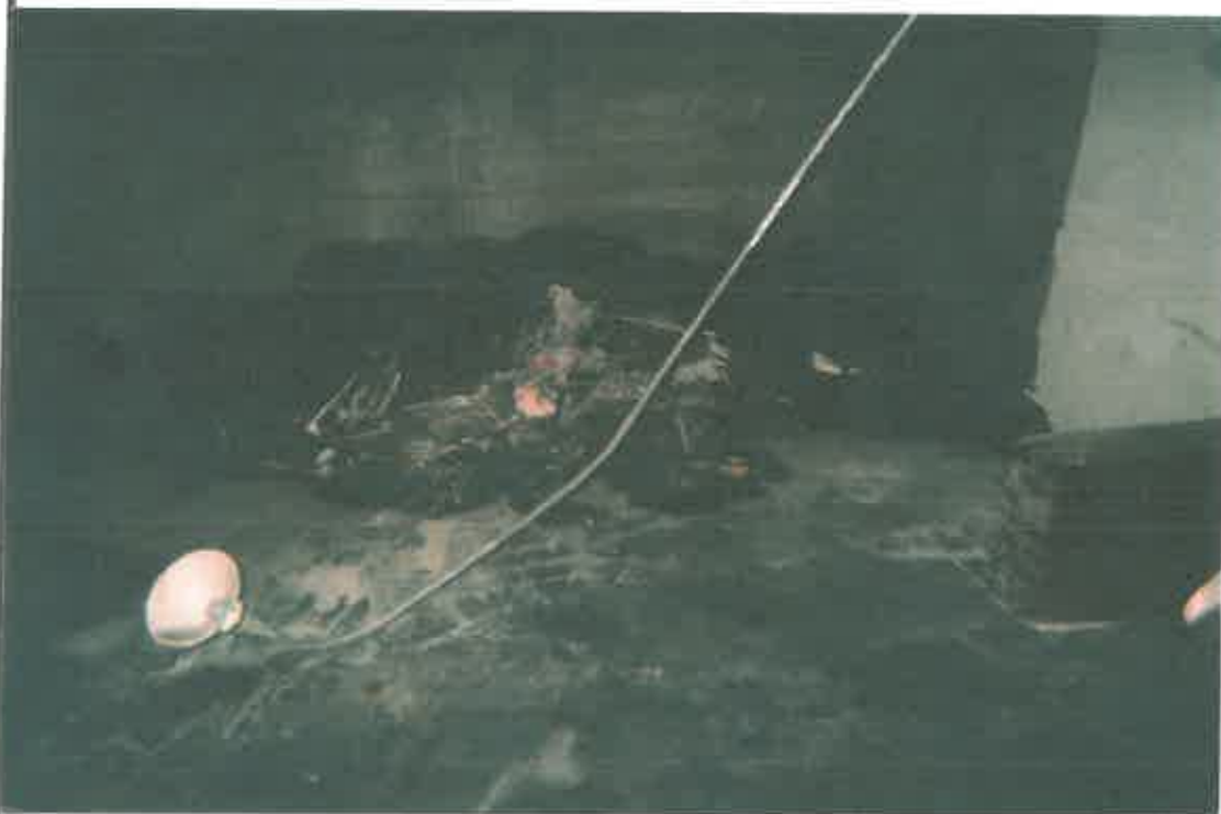
IFR - Trash before removal.
