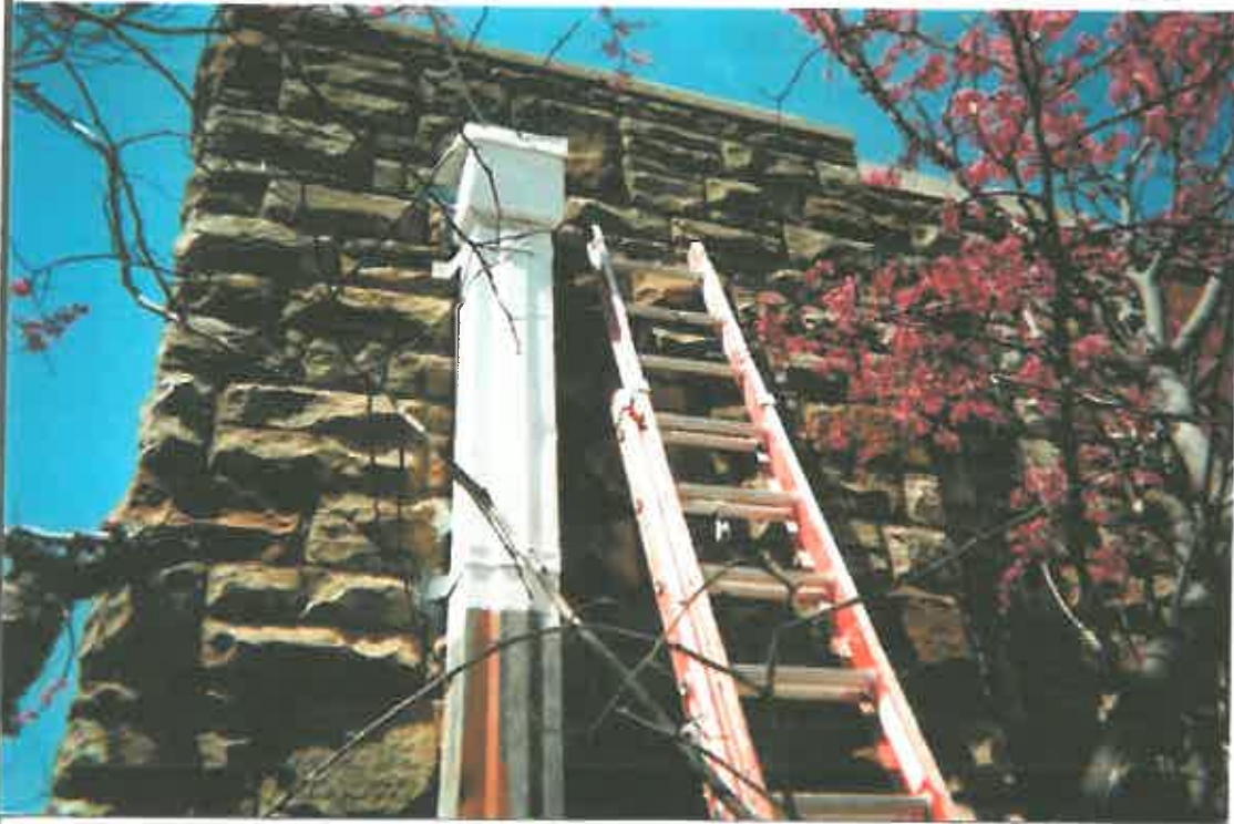
Downspout being encapsulated after abatement of loose and peeling paint.
