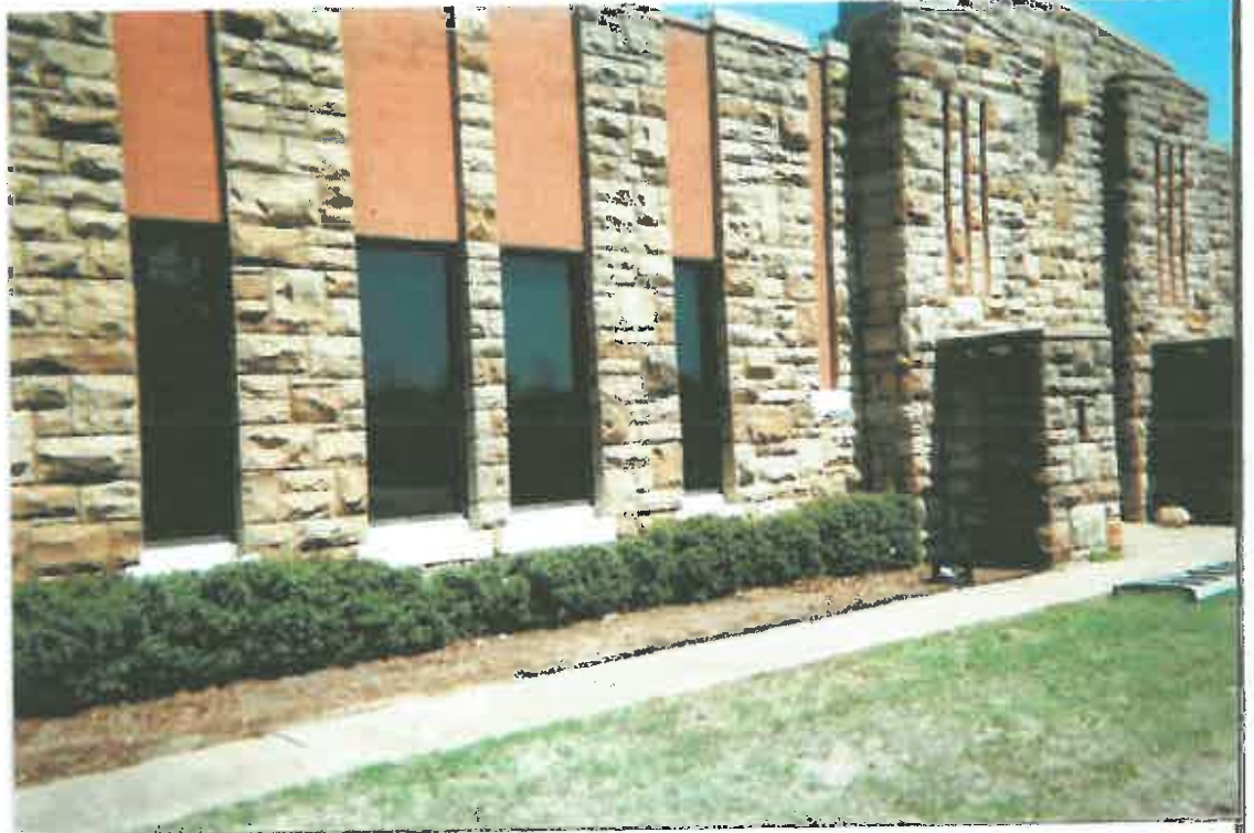
Exterior window lintels/sills after abatement and encapsulation.
