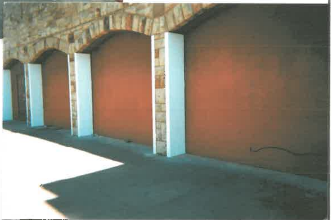
Bldg 1 - Door frame/guards after abatement and encapsulation.
