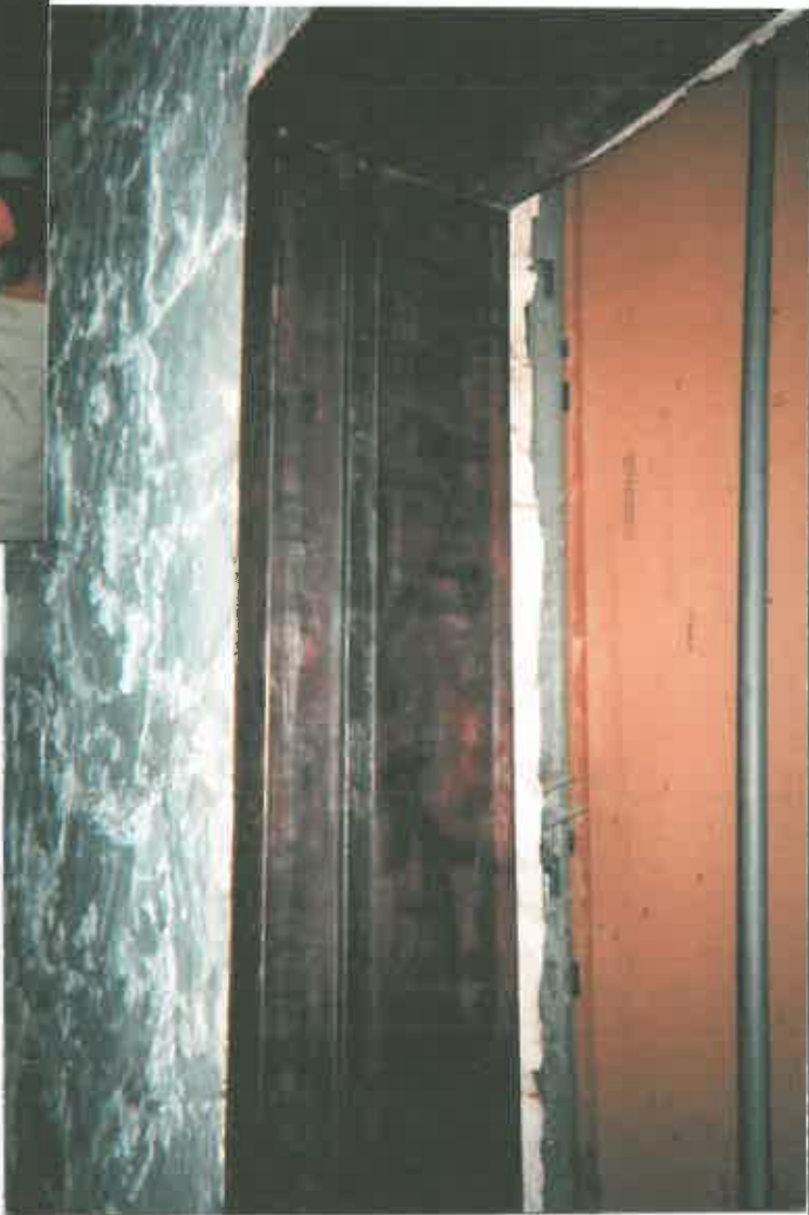
Door frame after abatement and before encapsulation.
