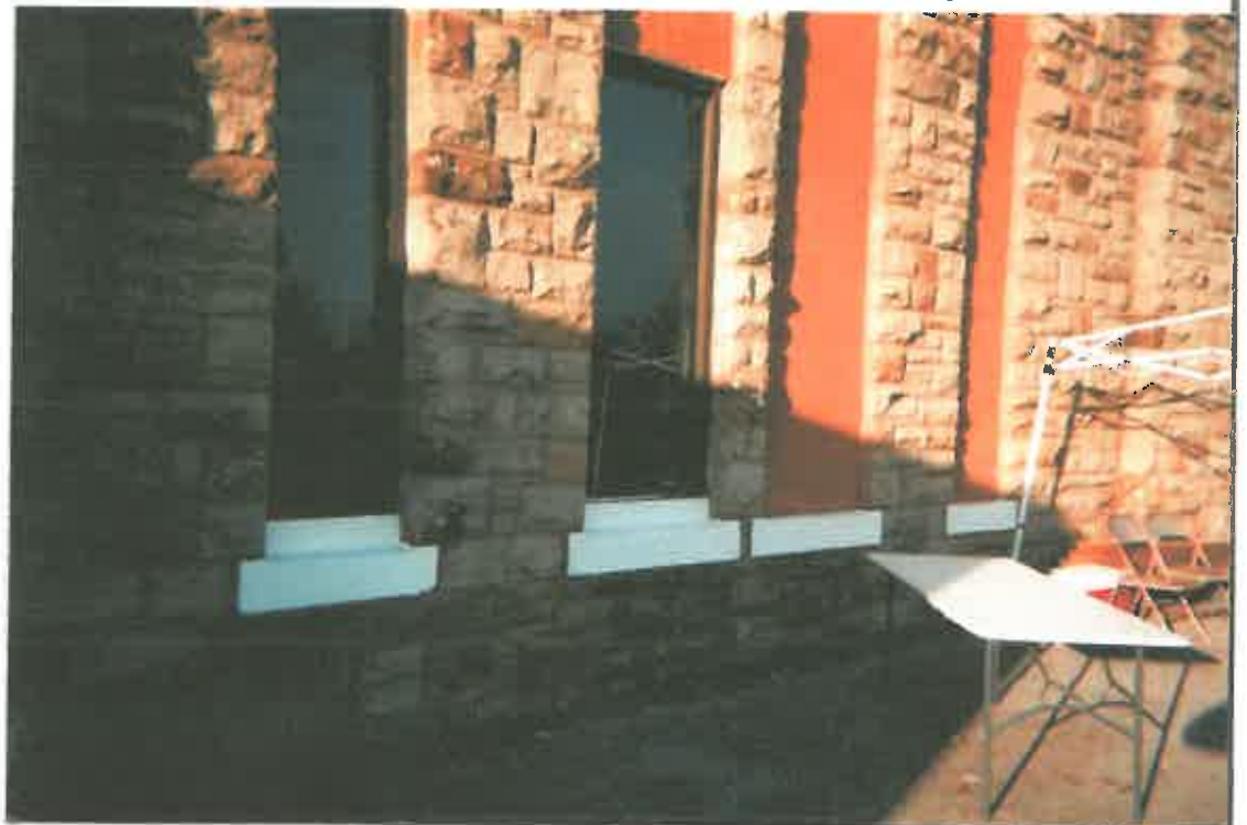
Window lintels and sills after abatement and encapsulation.
