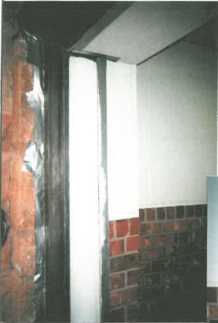
Door frame after abatement and during encapsulation.
