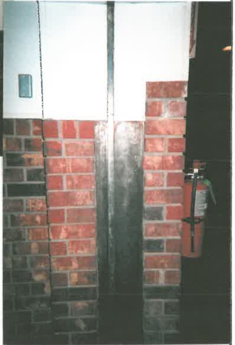
Door frame after abatement and before encapsulation.
