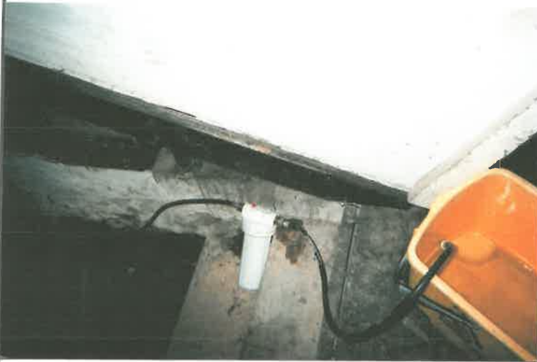
IFR - Pumping water out.
