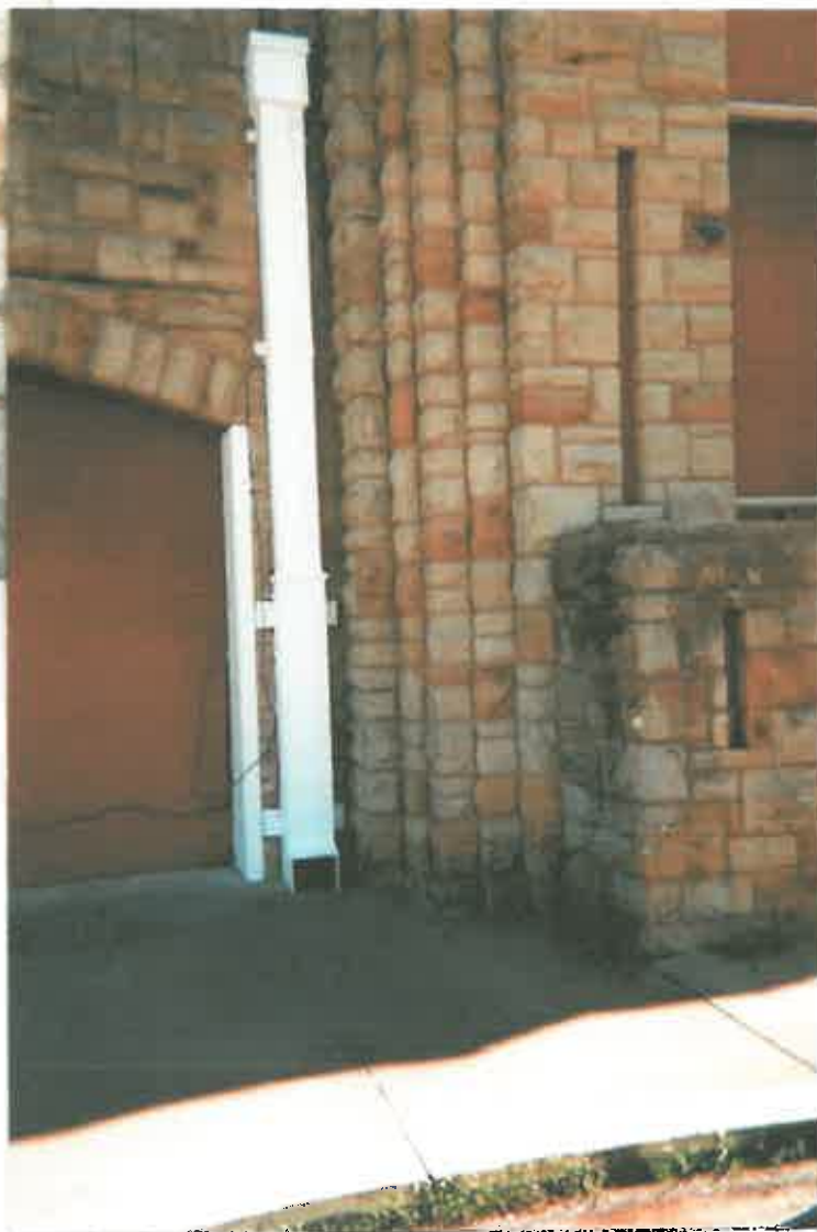
Bldg 1 - Downspout and door frame after abatement and encapsulation.
