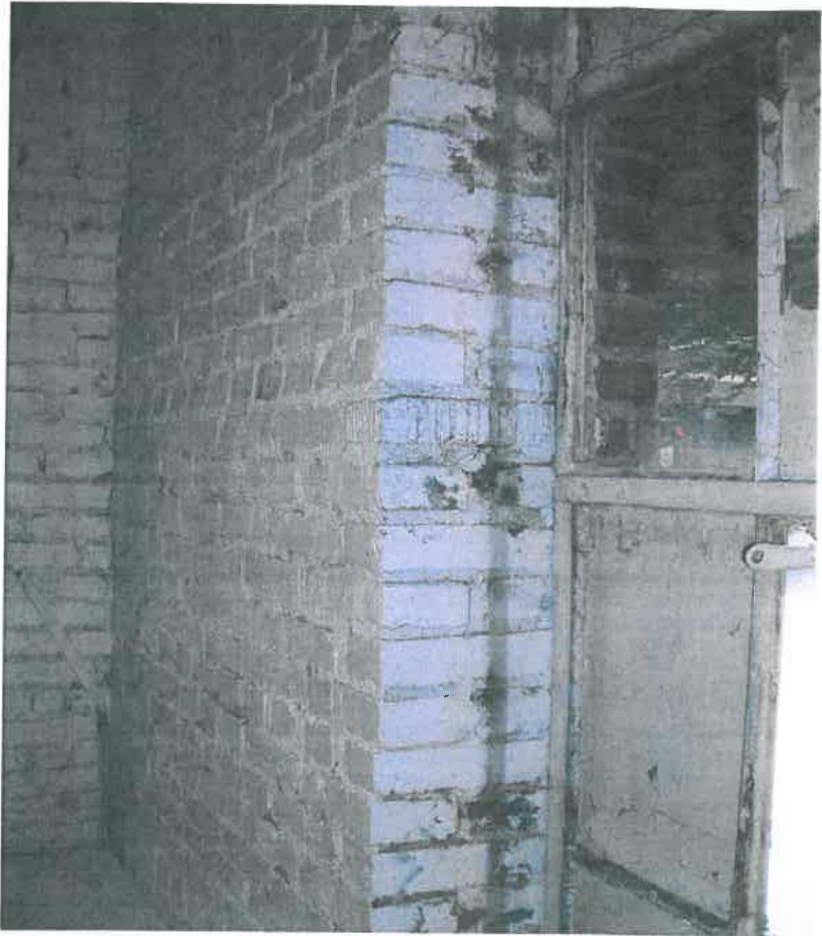
Room # 4 prior to window replacement.
