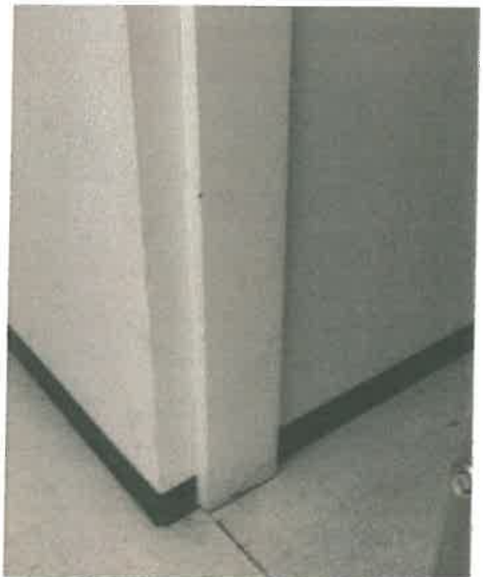
Room 14 entrance Concrete Door Jam
