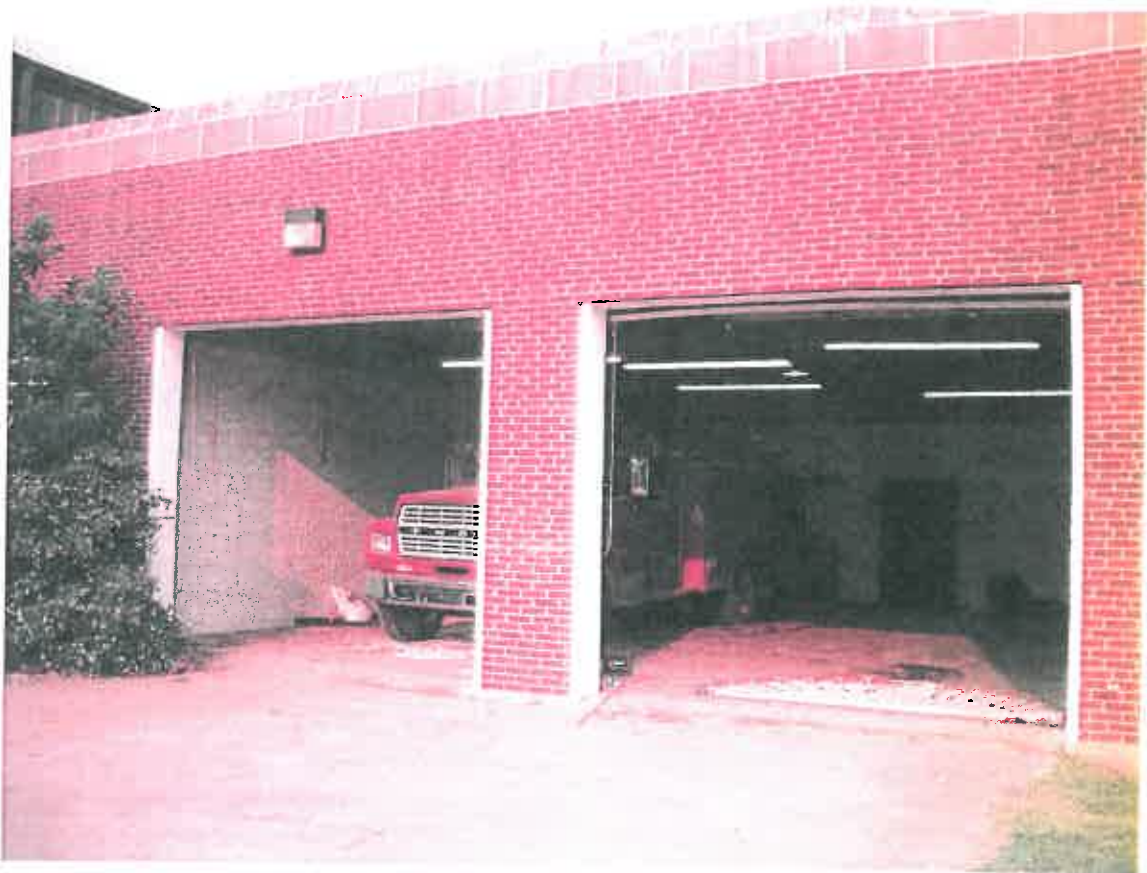
East Bay Doors post wet scrap and encapsulation
