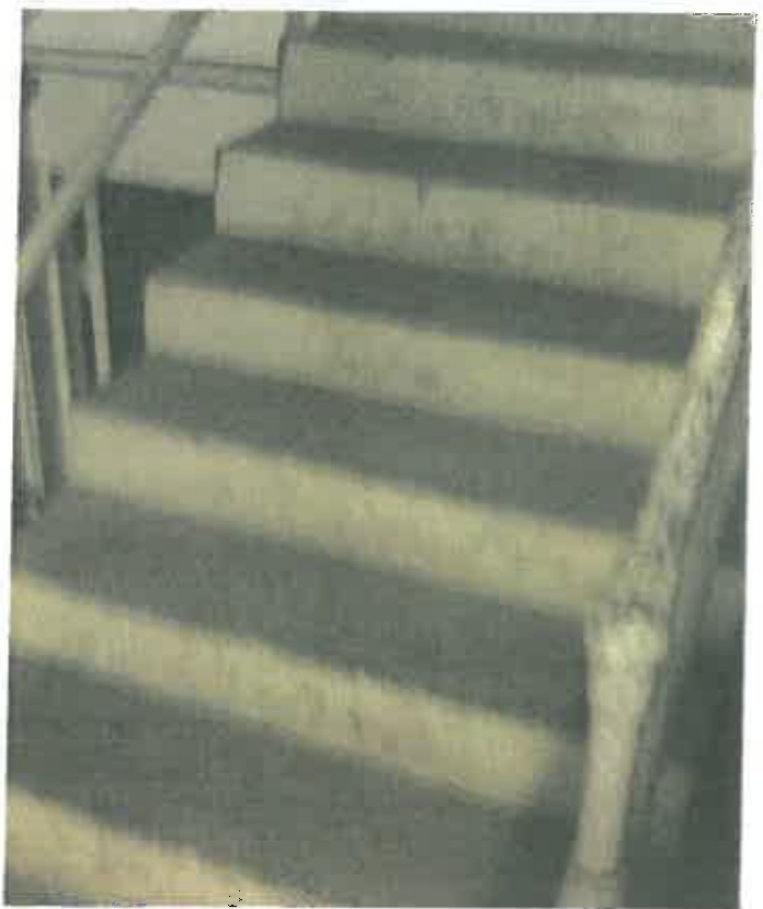
Room 19 concrete Staircase
