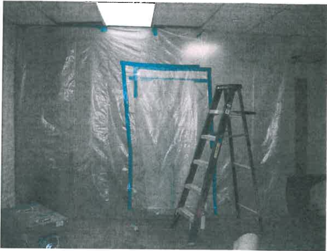
Critical Barrier Room # 10 Adjacent to Room # 12 (vault)
