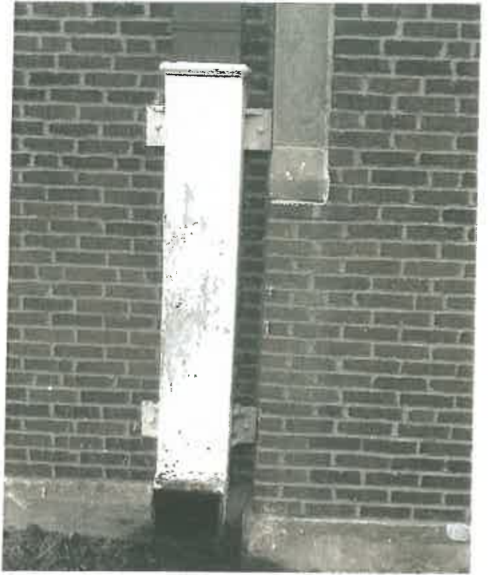
Drain B# 1 side B1
