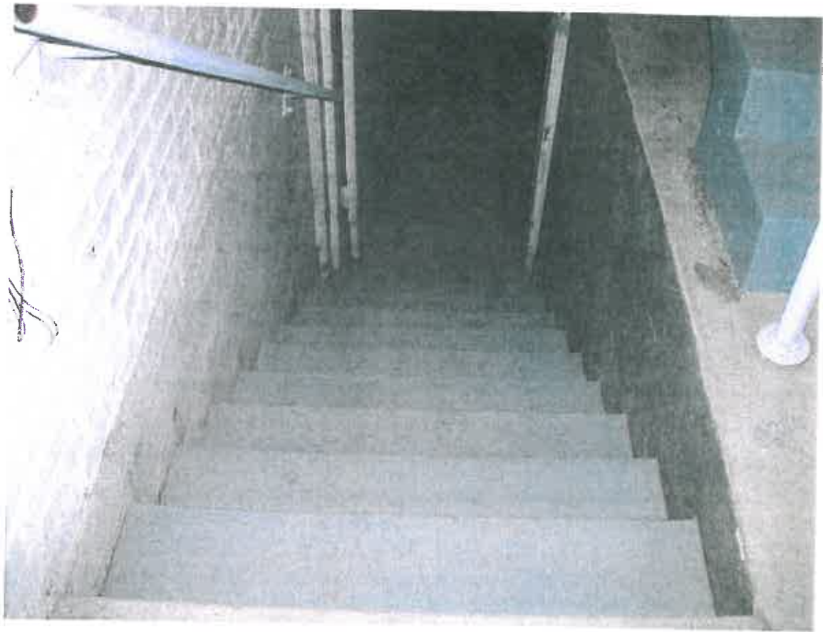
Stairs leading to IFR post encapsulation.
