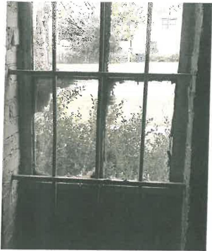
Room 22 window guard (side A)
