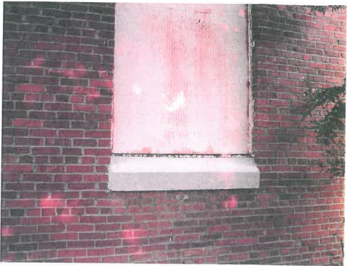
View showing a window sill prior to window installation
