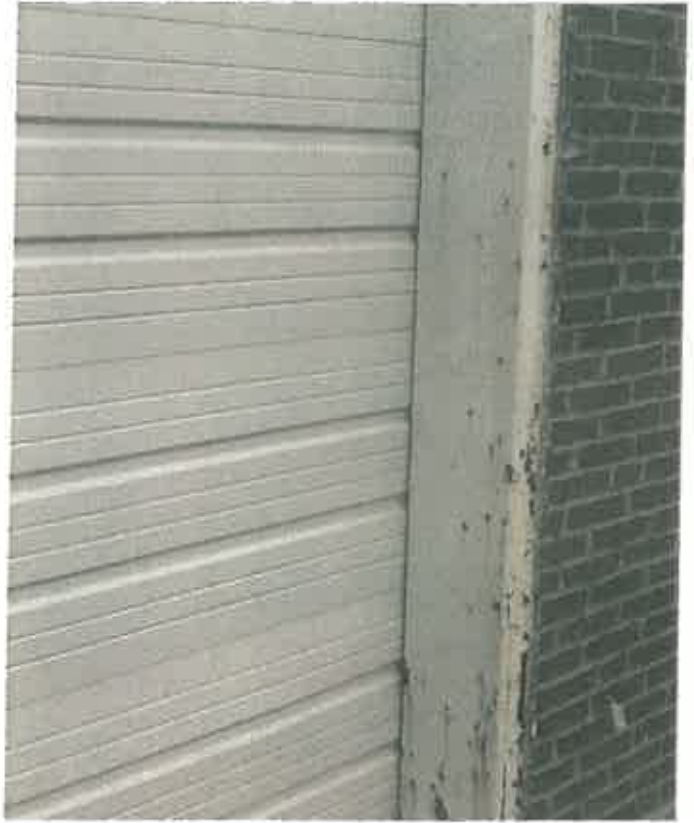
Garage Frame side B1
