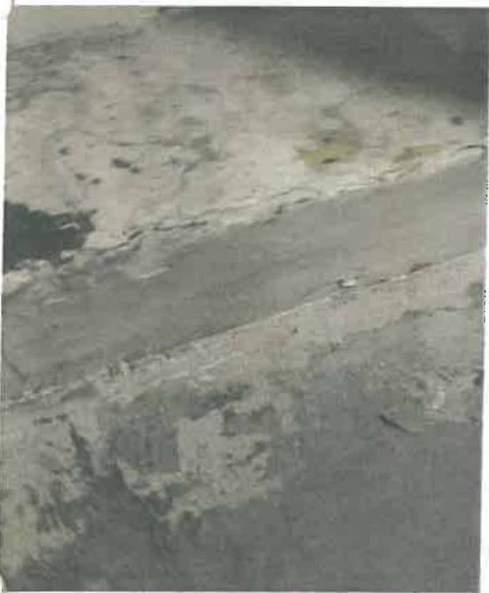
Room 10 stair side D
