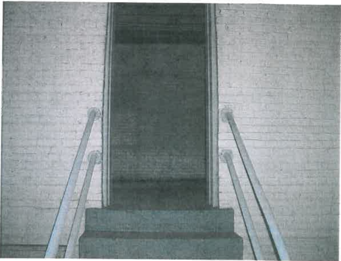
View of stairs leading into room # 17 post encapsulation.
