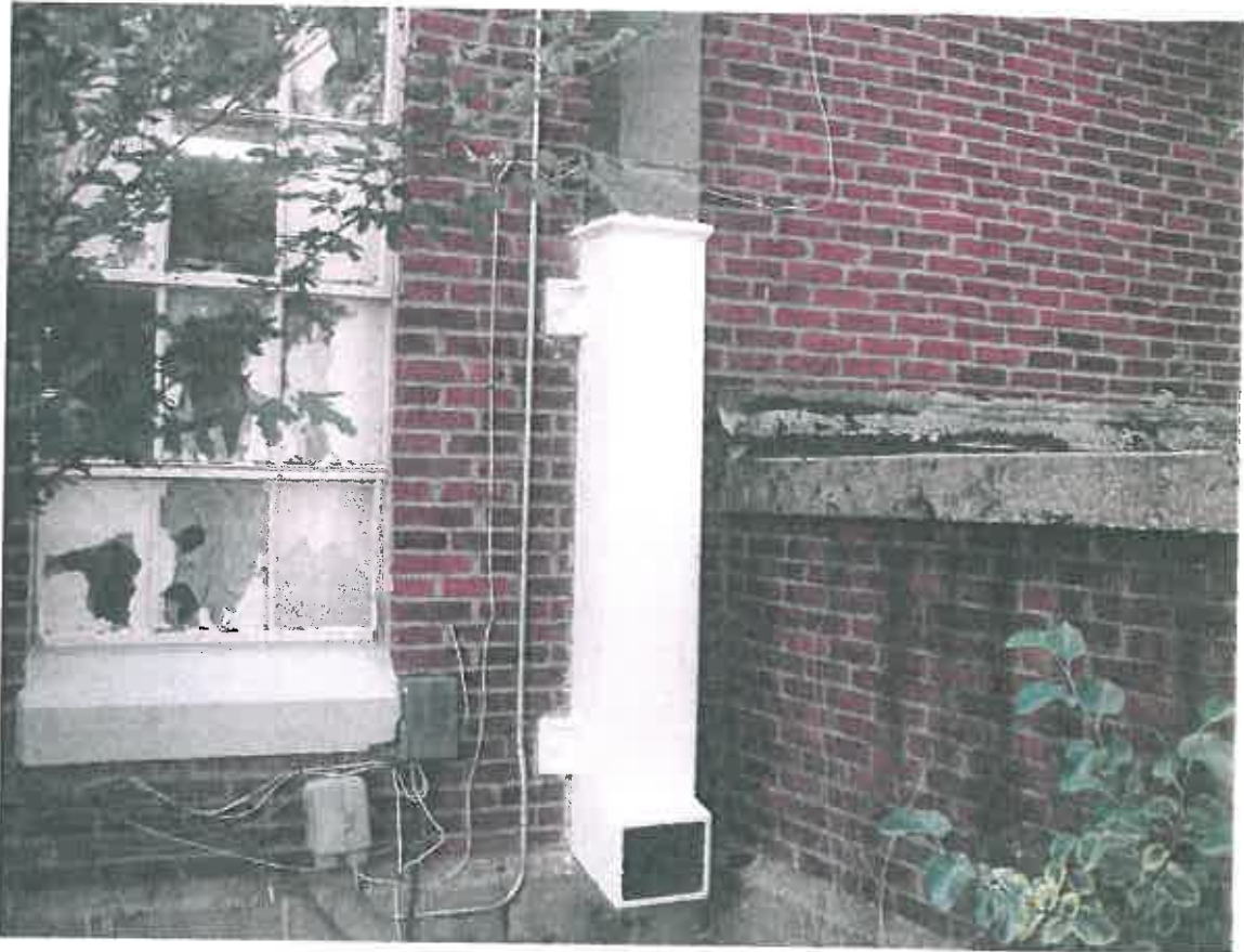
Down spout, East side of armory post wet scrape and encapsulation.
