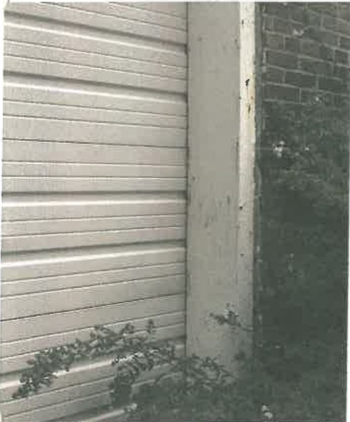
Garage Frame Side B2
