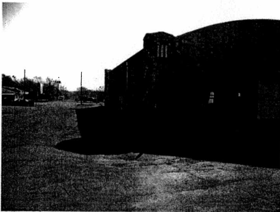
Photo 19. Corner of Janeway and Court Streets looking east down Court Street.
