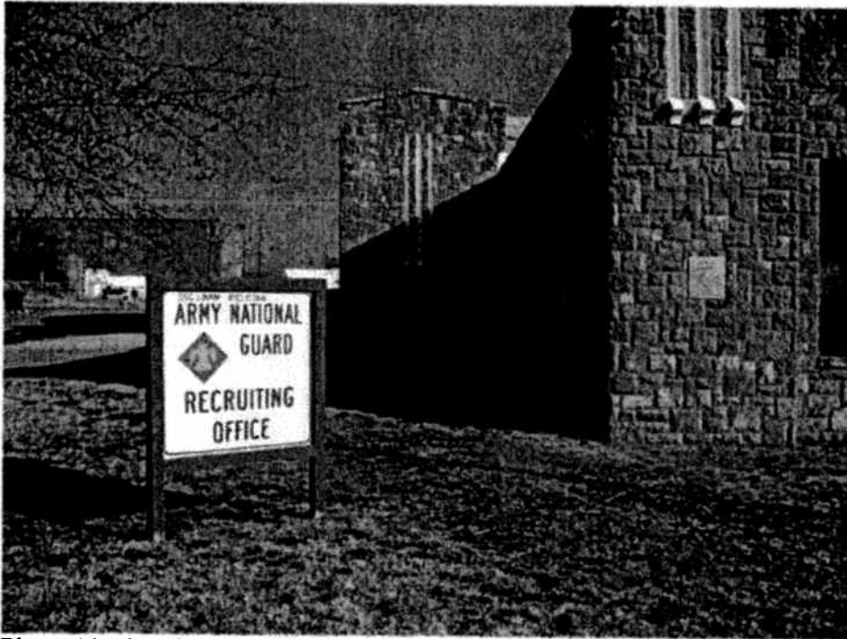
Photo 10. Southwest corner of the Armory noting active recruiting sign.
