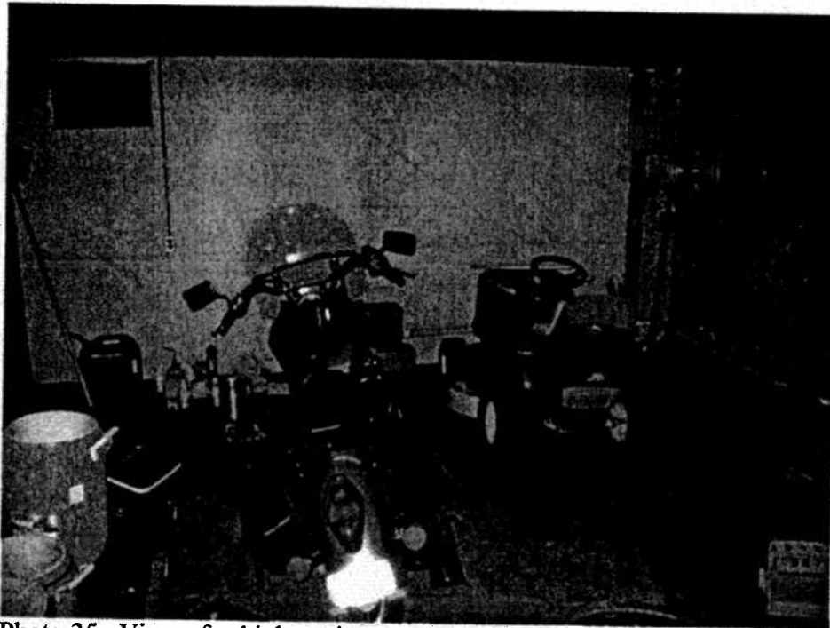
Photo 35. View of vehicle maintenance bay looking east from the bay door.
