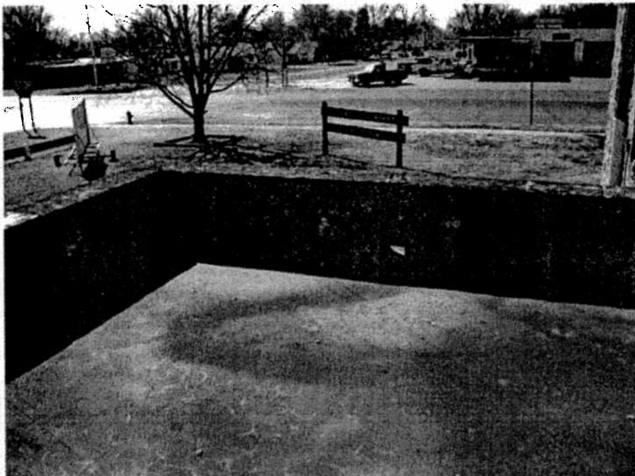
Photo 49. Mezzanine area located south of the room seen in photo 48.
