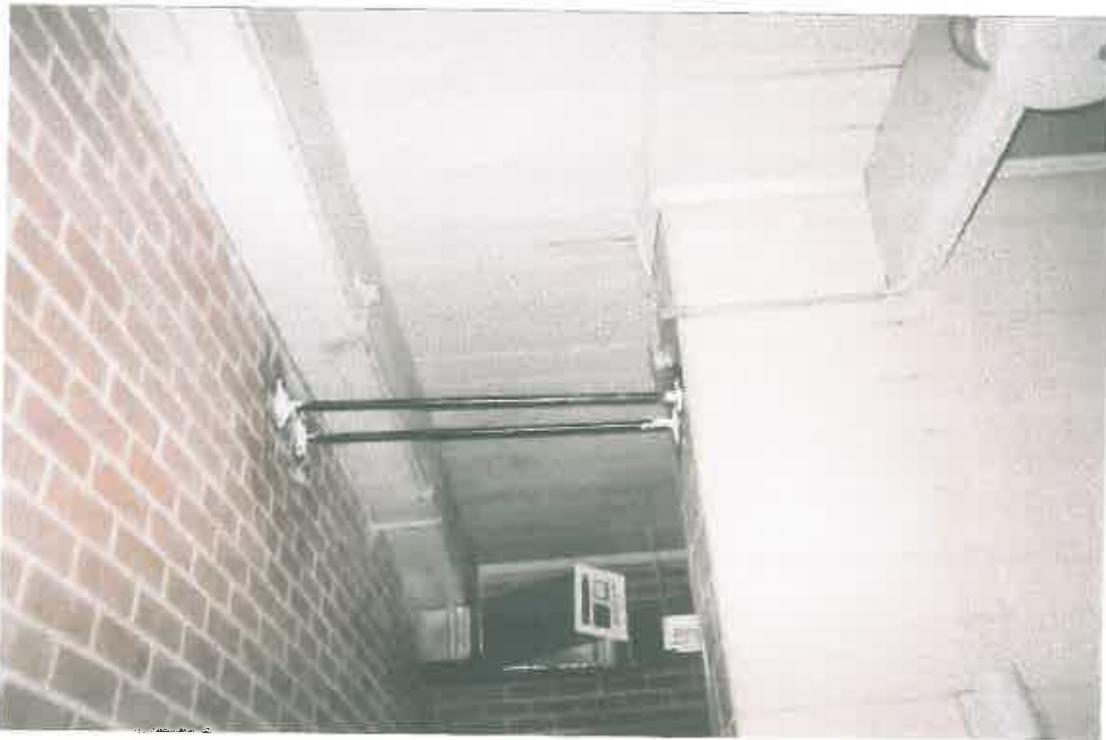
HA #8 & #9: PIPE INSULATION ABATED, PIPE "LOCKED DOWN" AND WALL PENETRATIONS SEALED
