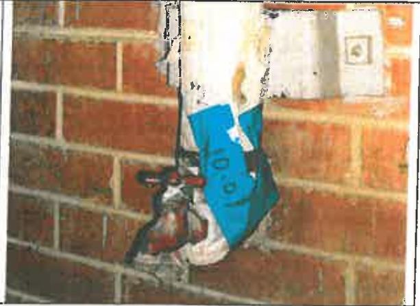
HA # 10: Pipe Fitting (Cold)
