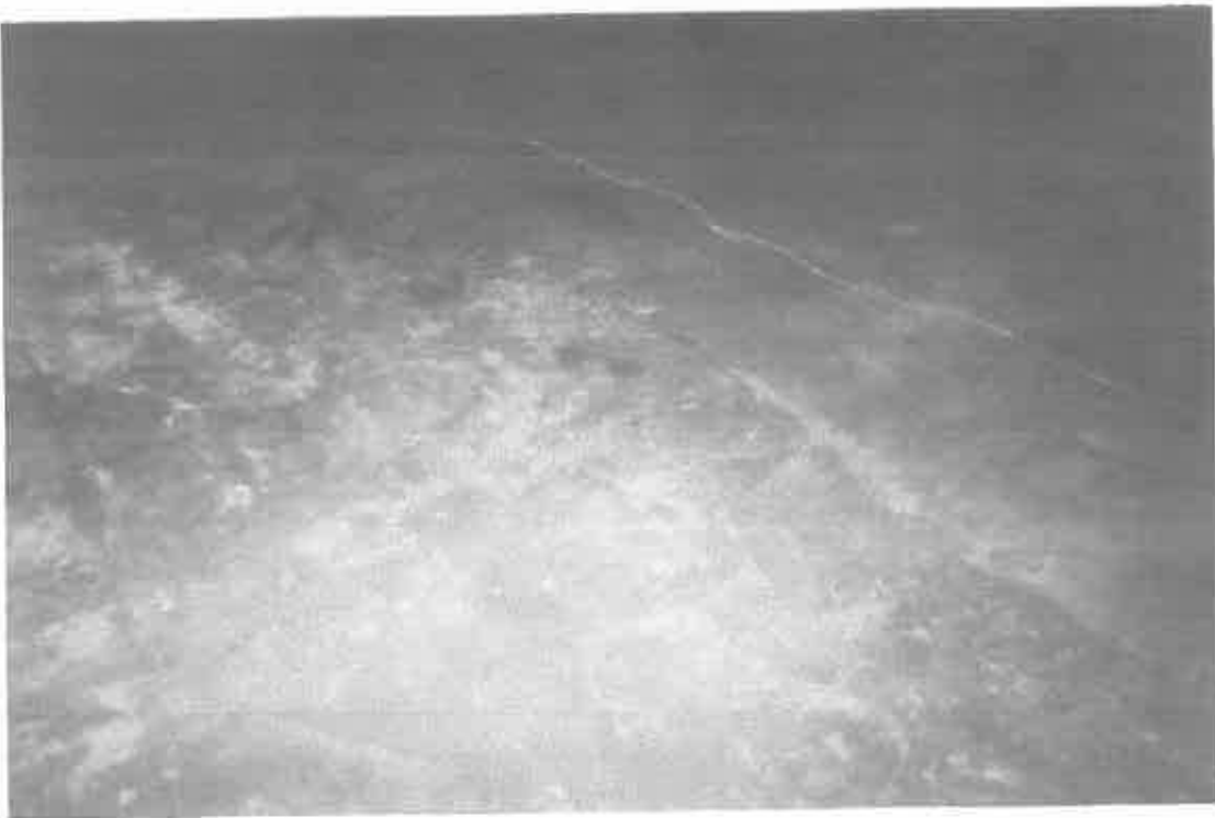
Room #1: FLOOR ABATED
