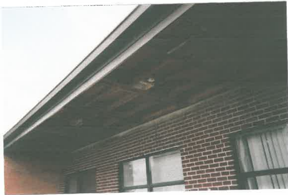
HA #1: TRANSITE PANELS ABATED
