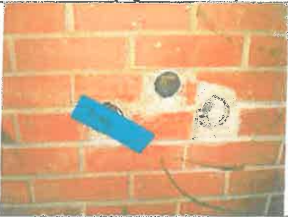
HA #11: Pipe Fitting (Hot)
