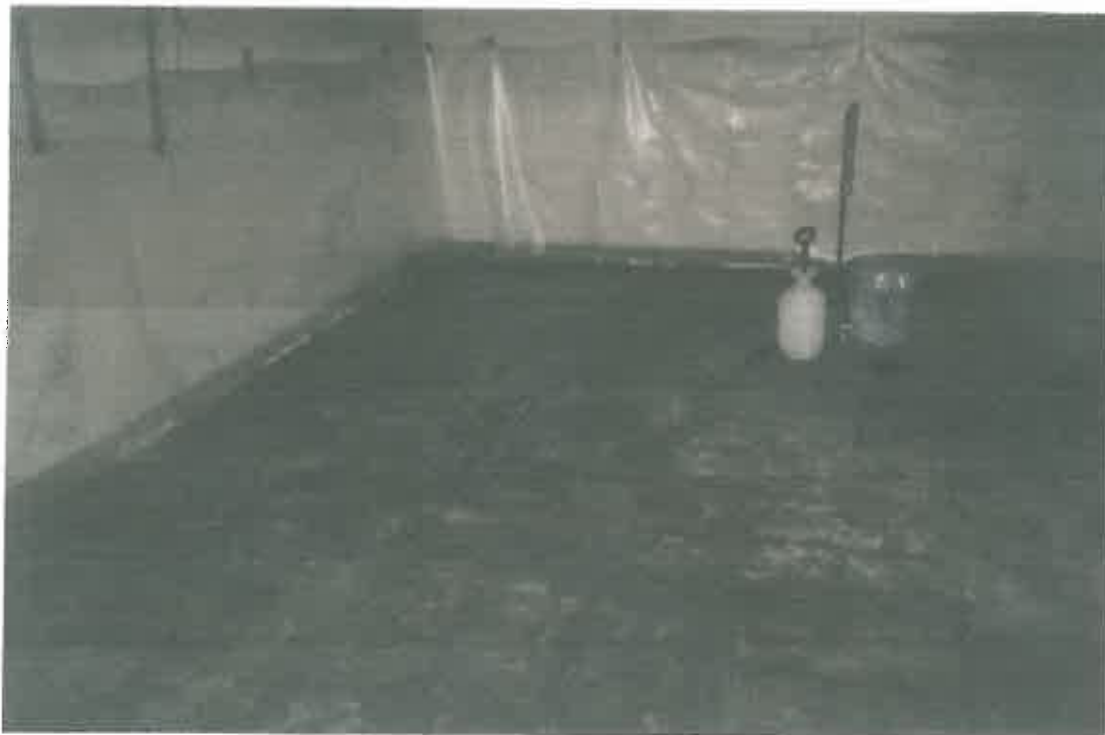
HA #3: FLOOR TILE AND MASTIC ABATED
