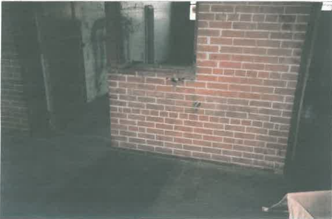
PHOTO #5 BLACK PAINTED PASS THROUGH WINDOW SILL IN ROOM 14 - LBP - ABATED
