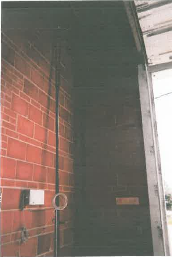
HA #8 & #9: PIPE INSULATION ABATED AND PIPE "LOCKED DOWN"
