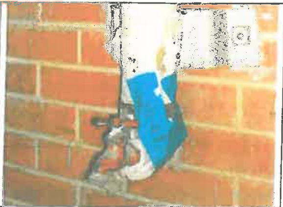
HA #10: Pipe Fitting (Cold)
