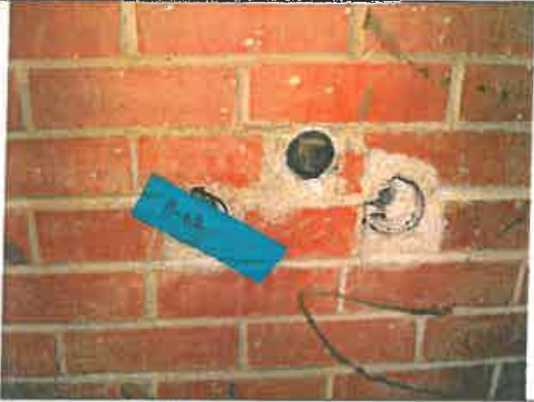
HA #11: Pipe Fitting (Hot)
