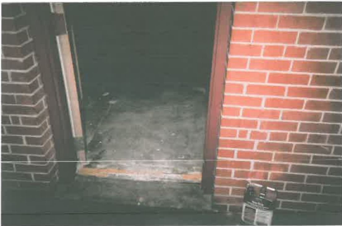
ROOM #6: FLOOR ABATED
