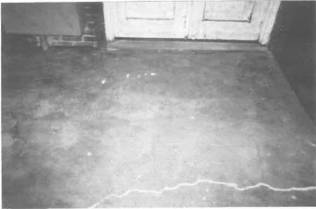
Room #1: FLOOR ABATED
