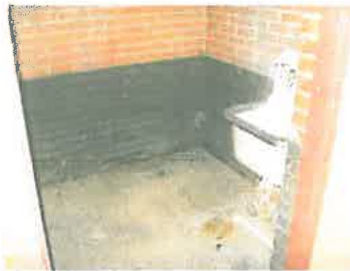
Photo # 6: Green painted brick wall in Room 18 - LBP.
