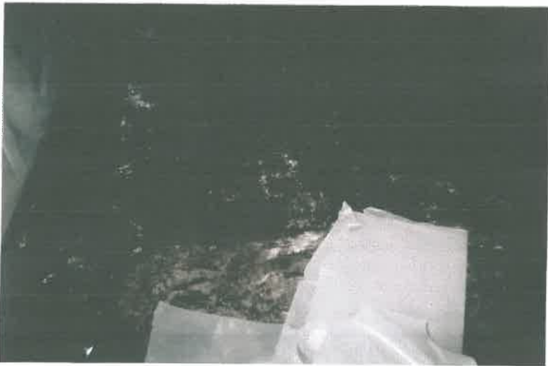
FLOOR BEING ABATED
