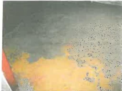
Photo # 4: Yellow, red, and gray painted concrete floor in Room 11 - LBP.
