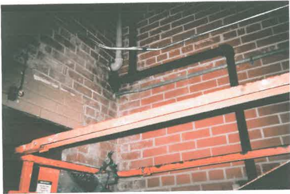
HA #8 & #9: PIPE INSULATION ABATED AND PIPE "LOCKED DOWN"
