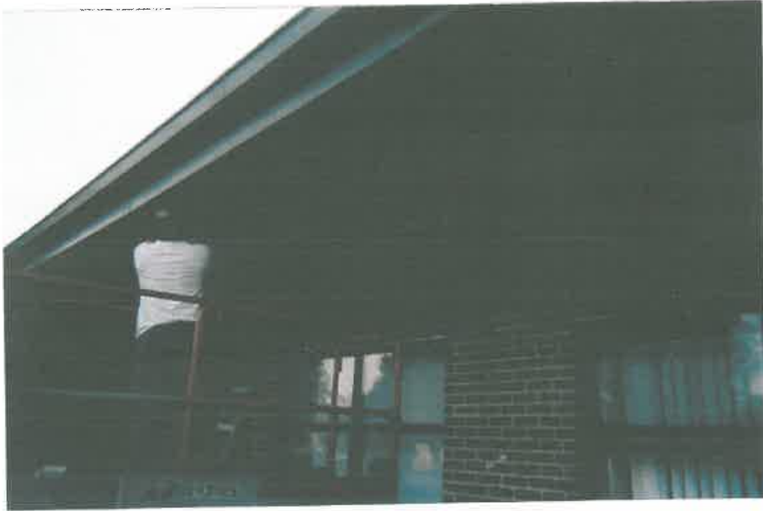
HA #1: ABATING TRANSITE PANELS
