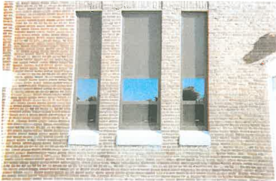
NEW WINDOWS AND SEALED SILLS
