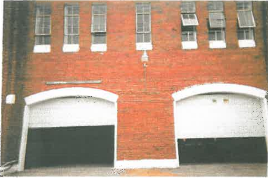
ORIGINAL WINDOWS AND SILLS
