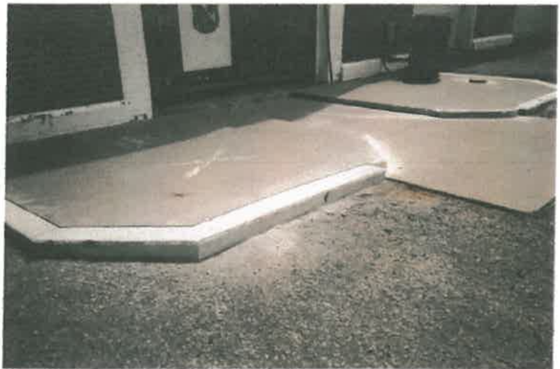
CONCRETE CURB – SEALED
