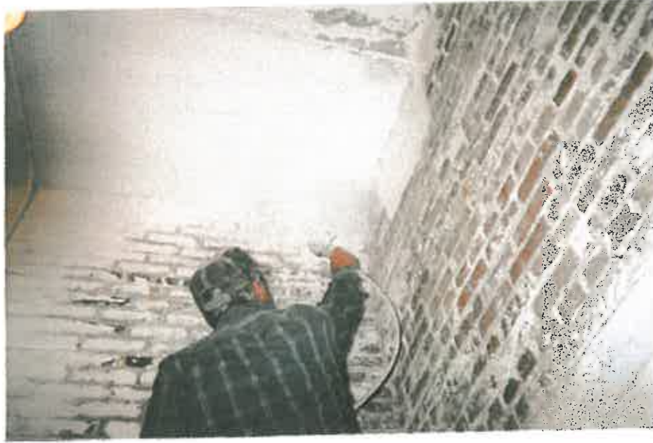
LOOSE AND PEELING LEAD BASED PAINT REMOVED – BEING SEALED
