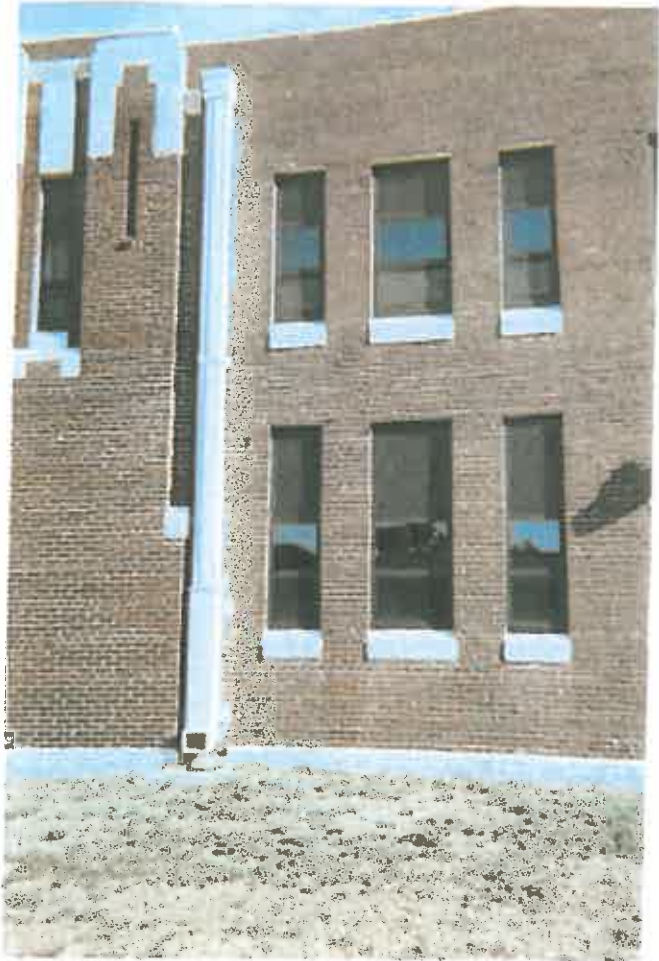
NEW WINDOWS, SILLS, DOWNSPOUT - SEALED
