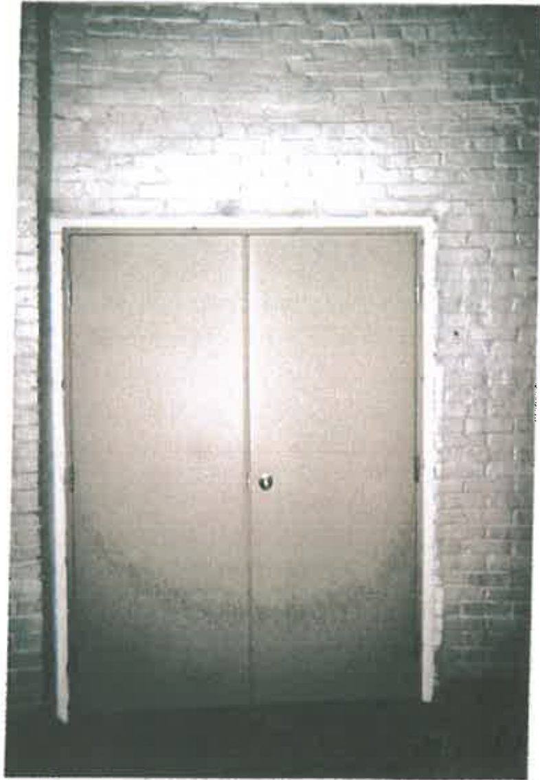
NEW DOOR – AND STAGE LEAD BASED PAINT TO BE REMOVED
