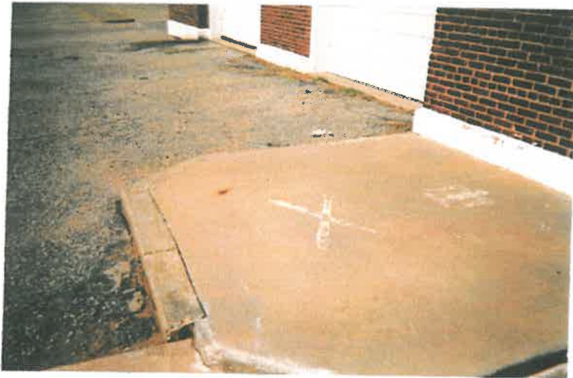
CONCRETE CURB – LEAD BASED PAINT REMOVED
