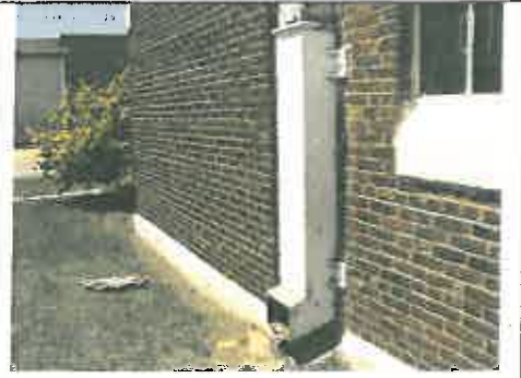
Roof Drain - Side D #2
