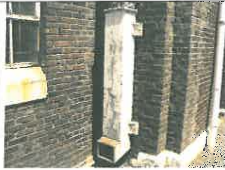
Roof Drain - Side D #1
