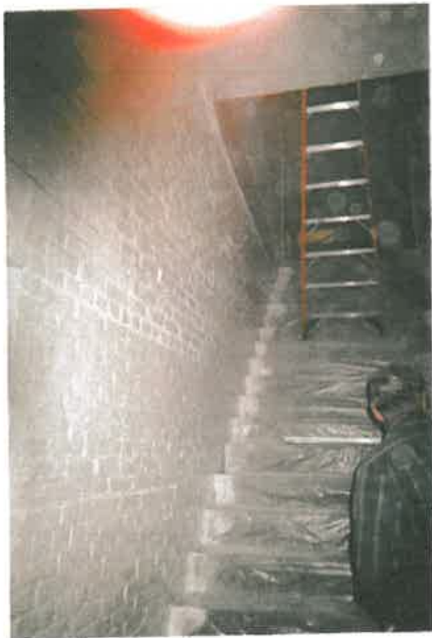
STAIRWELL AFTER REMOVAL – SEALED
