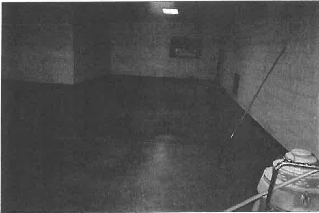
Floor - HEPA vacuumed and mopped, Room 9 (view to the South)
