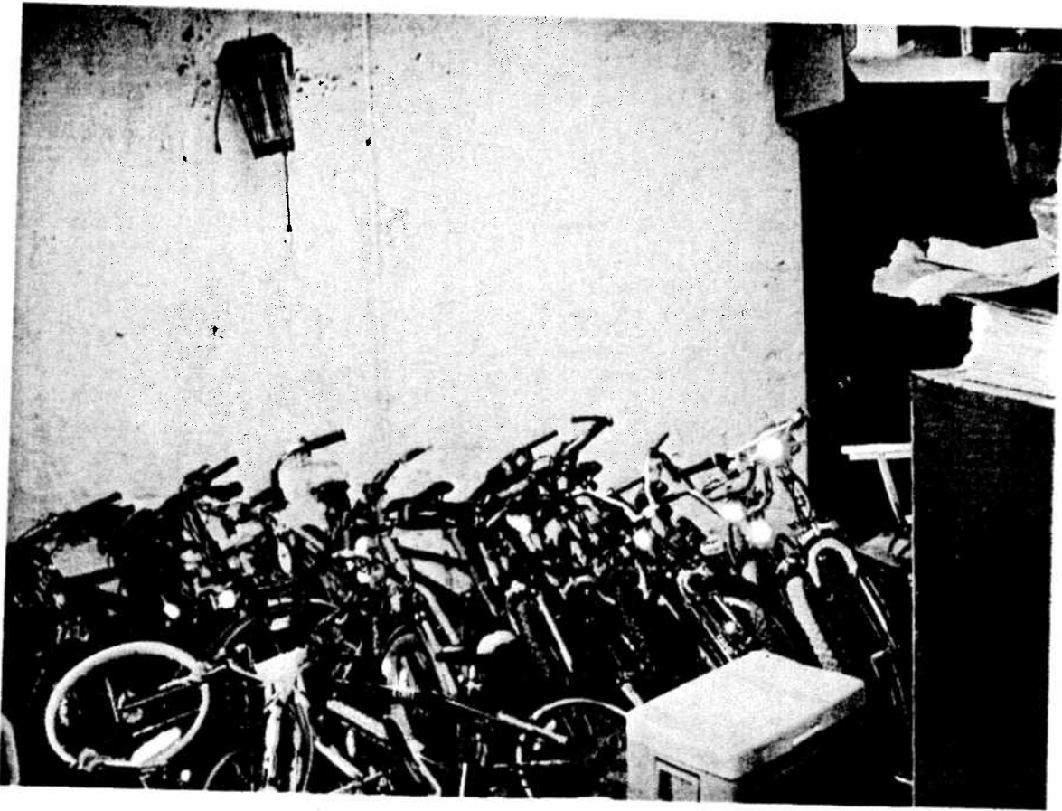
Figure 11. Hominy Armory – Hominy police impound storage room – note flaking original painted wall.
