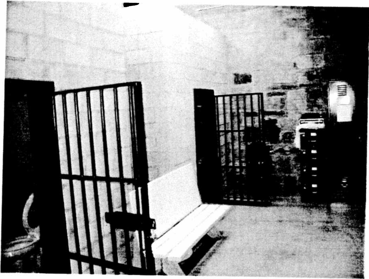
Figure 10. Hominy Armory – Hominy jail facility in the northeast side of the building – note the original walls were not painted
