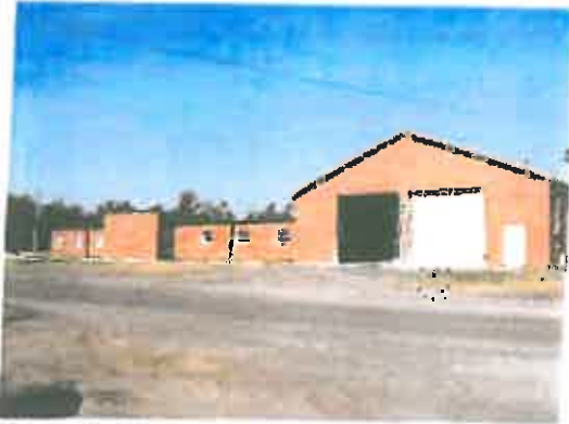
Photo #1: Hobart National Guard Armory.
