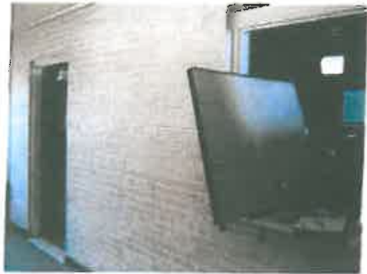
Photo #14: White painted brick wall in Room 3 - LBP
