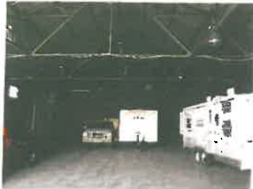
Photo #8: Roof trusses and supports in Room 1 - LBP.
