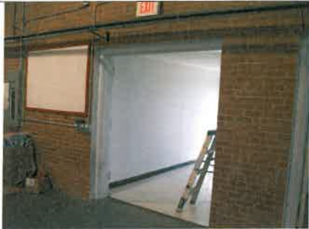
Reading 284, Room 7, Wood Door Frame
