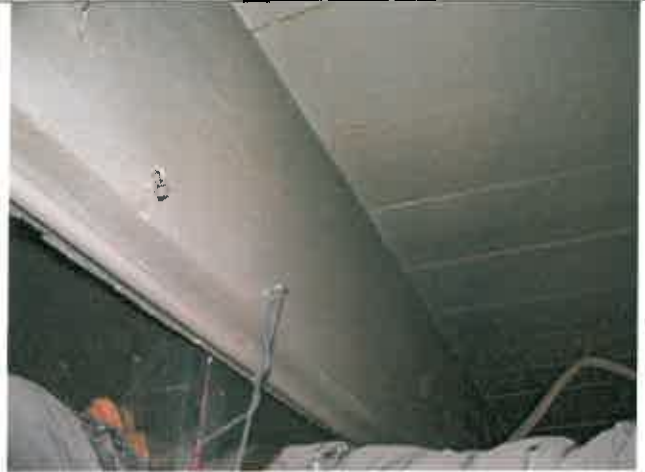
Rd. 285-286, Room 7, Ceiling Beams & Decking
