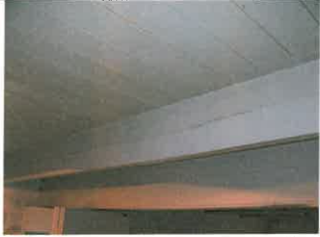
Rd. 321-323, Room 11, Ceiling Beam & Decking
