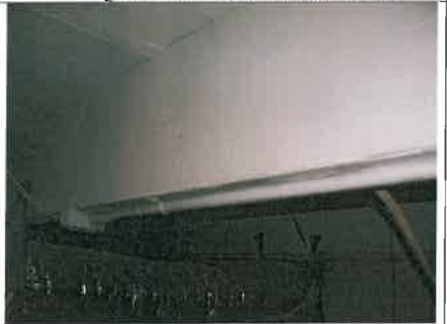
Rd. 305, Room 9, Ceiling Beam
