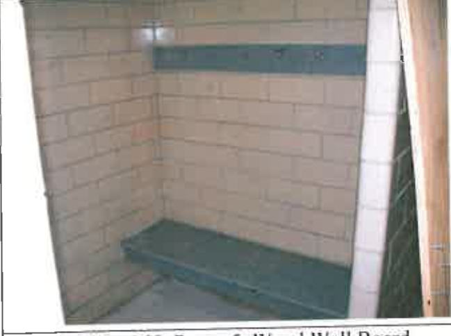
Reading 265, Room 5, Wood Wall Board Reading 266, Room 5, Wood Bench
