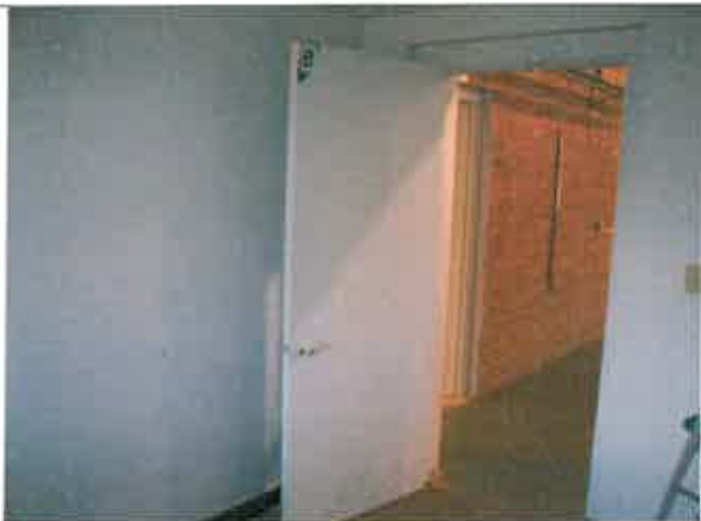
Reading 302, Room 9, Wood Door Frame Reading 303, Room 9, Wood Door
