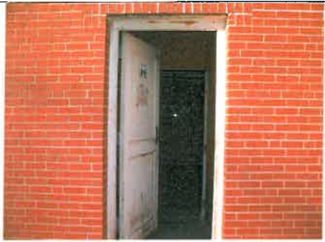
Reading 351, Annex 1, Metal Door Frame
