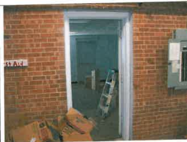
Reading 275, Room 6, Wood Door Frame
