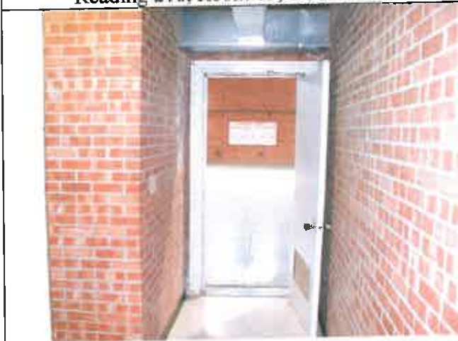
Reading 248, Room 4, Wood Door Frame
