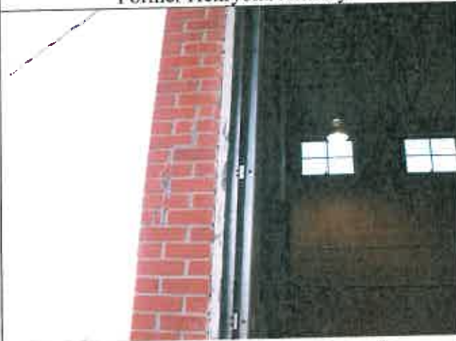
Reading 211, Room 13, Garage Door Frame
