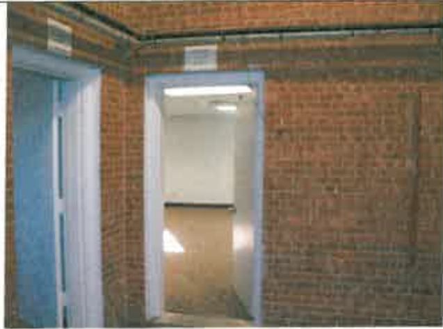
Reading 311, Room 10, Wood Door Frame
