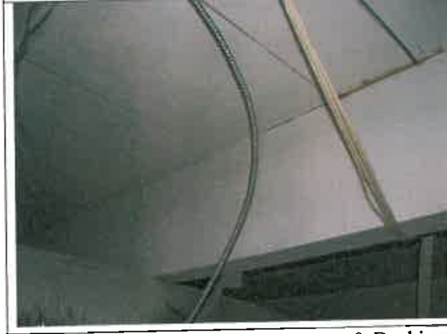
Rd. 276-277, Room 6, Ceiling Beams & Decking
