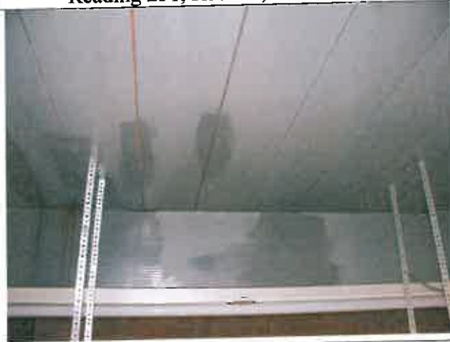
Rd. 263 - 264, Room 5, Ceiling Beam & Decking
