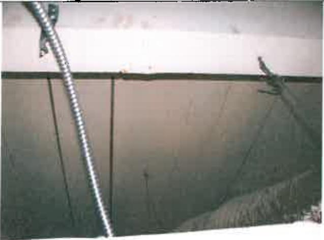
Rd. 287, Room 8, Ceiling Decking
