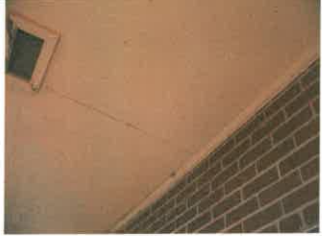
Reading 342, Exterior, Wood Porch Ceiling Reading 343, Exterior, Wood Porch Upper Trim
