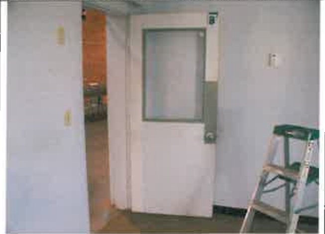
Reading 289, Room 8, Wood Door Reading 291, Room 8, Wood Door Frame
