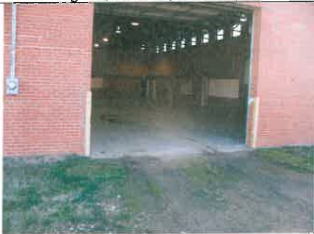
Reading 344, Exterior, Metal Garage Door Fascia
