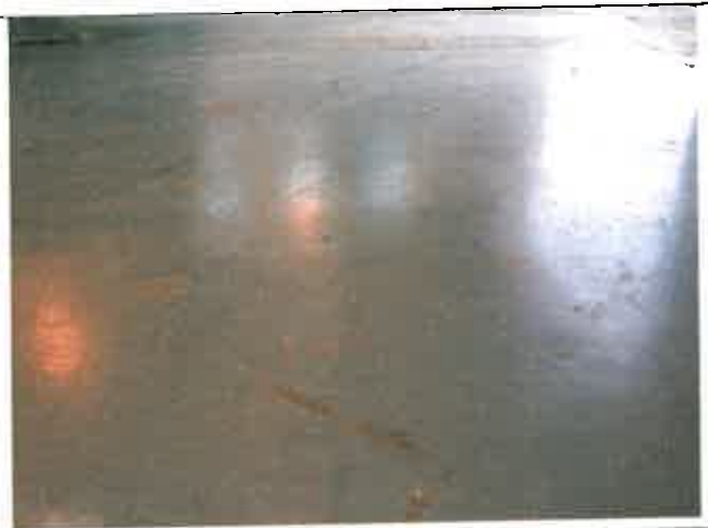
Reading 210, Room 13, Concrete Floor
