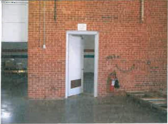
Reading 327, Room 12, Wood Door Reading 328, Room 12, Wood Door Frame
