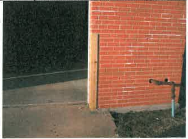
Reading 349, Annex 1, Metal Garage Door Fascia
