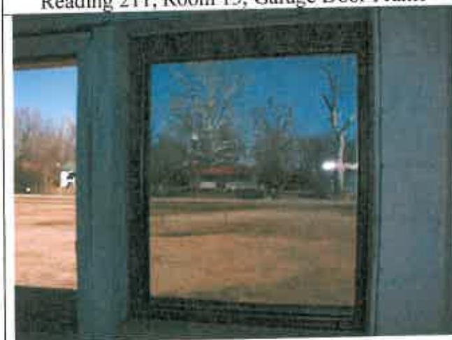
Reading 242, Room 3, Wood Window Frame
