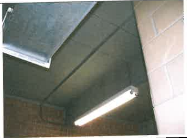
Rd. 253 - 254, Room 4, Ceiling Beams & Decking
