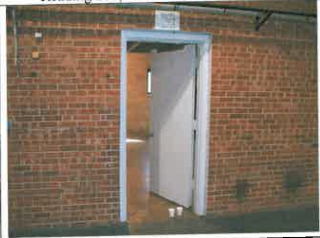
Reading 218, Room 13, Door Frame
