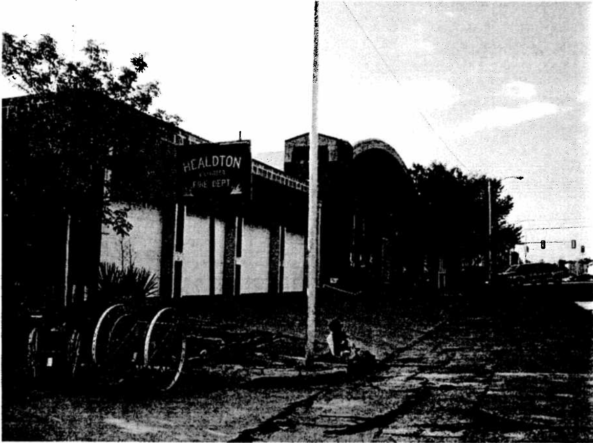
Figure 3: Healdton Armory - northwest corner, west entrance facing south.
