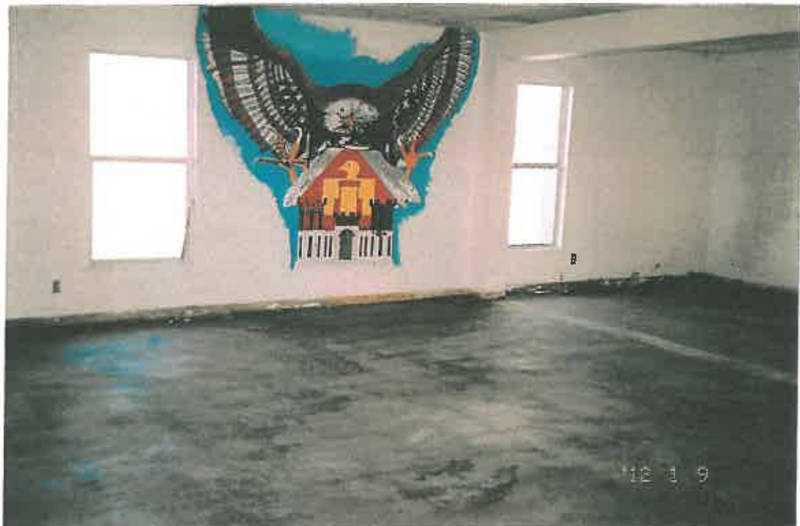
Floor tile and Mastic removed, Room 1
