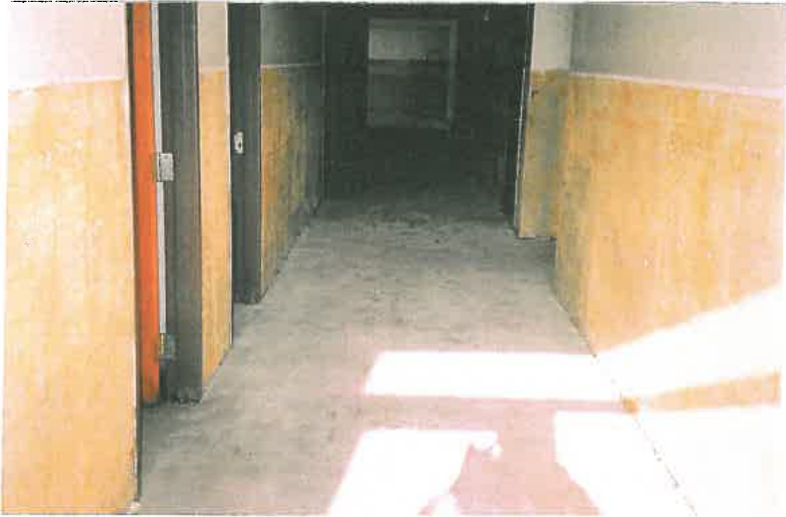
Floor tile and Mastic removed, N/S hallway
