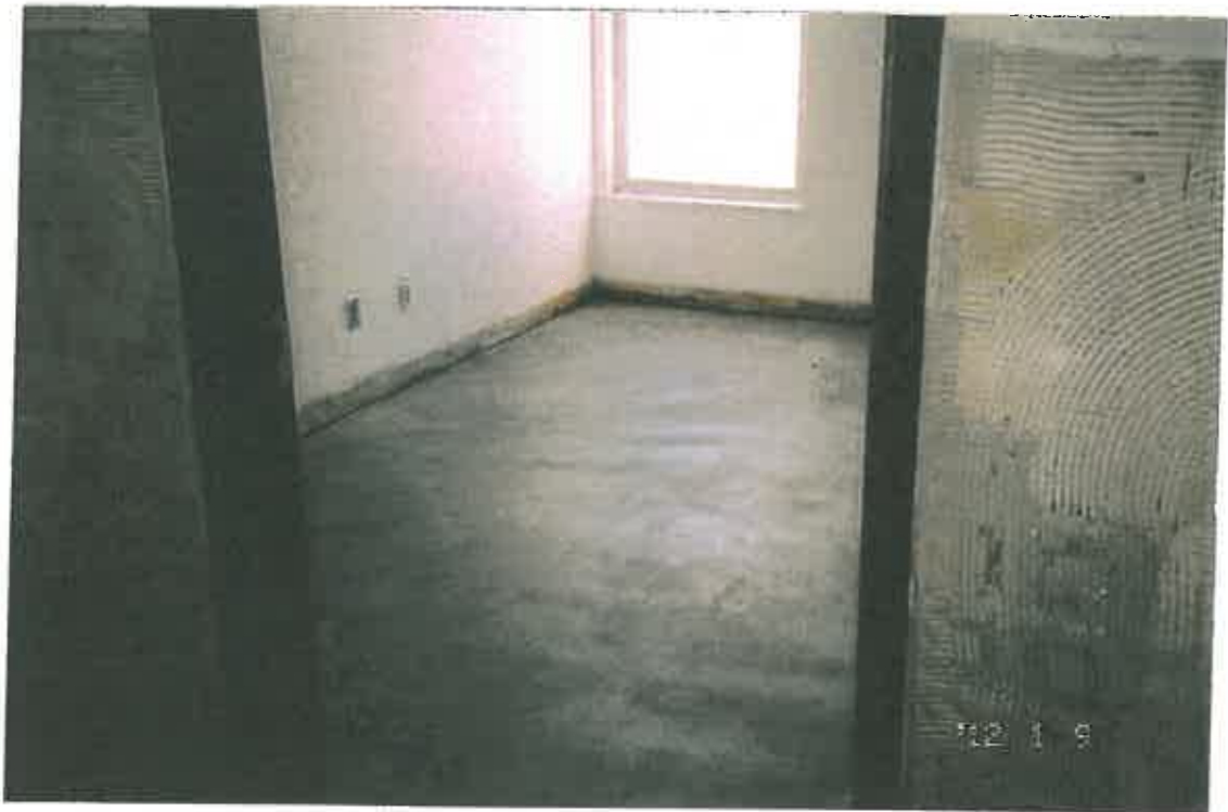
Floor tile and mastic removed, Room 13
