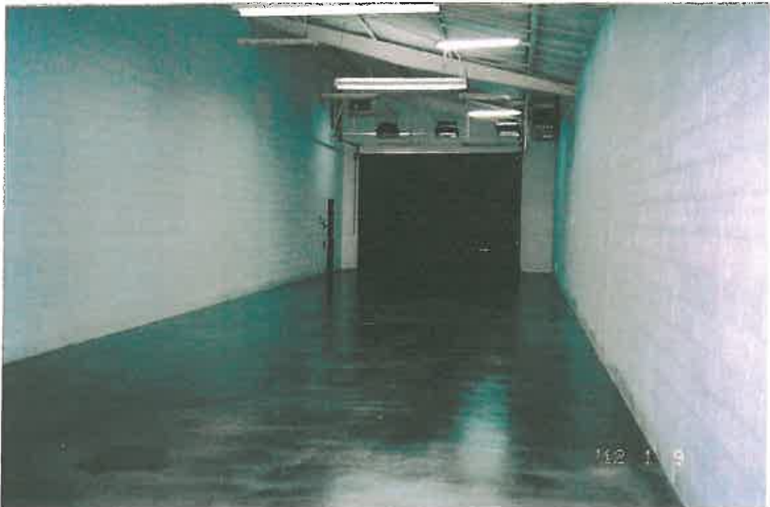
IFR, cleaned and sealed (view to the East)
