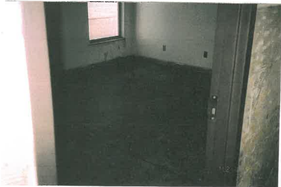
Floor tile and Mastic removed, Room 12
