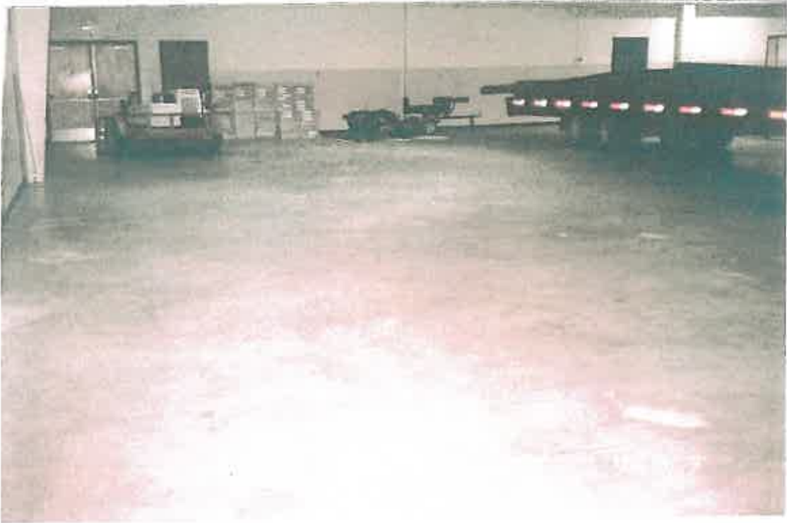
Drill floor, Mopped and HEPA-vacuumed
