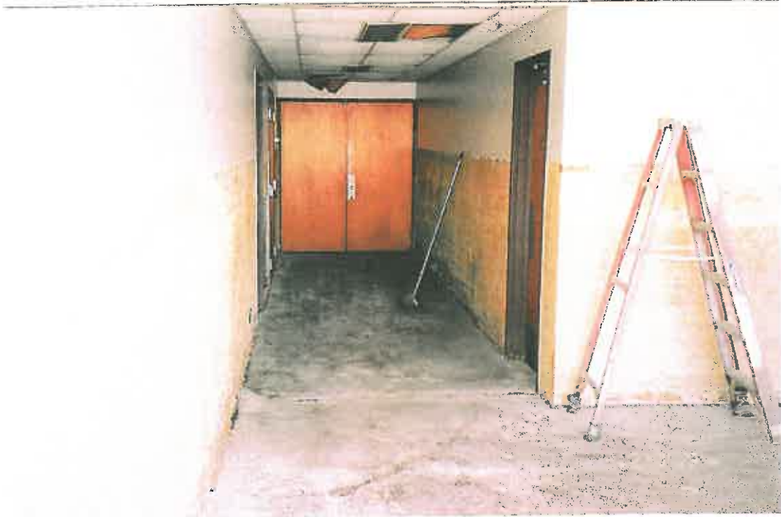
Floor tile and Mastic removed, Main Entry and hallway
