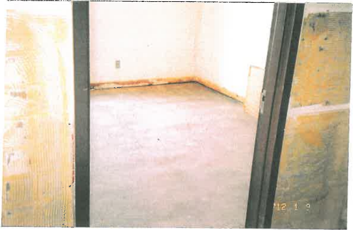
Floor tile and Mastic removed, Room 15
