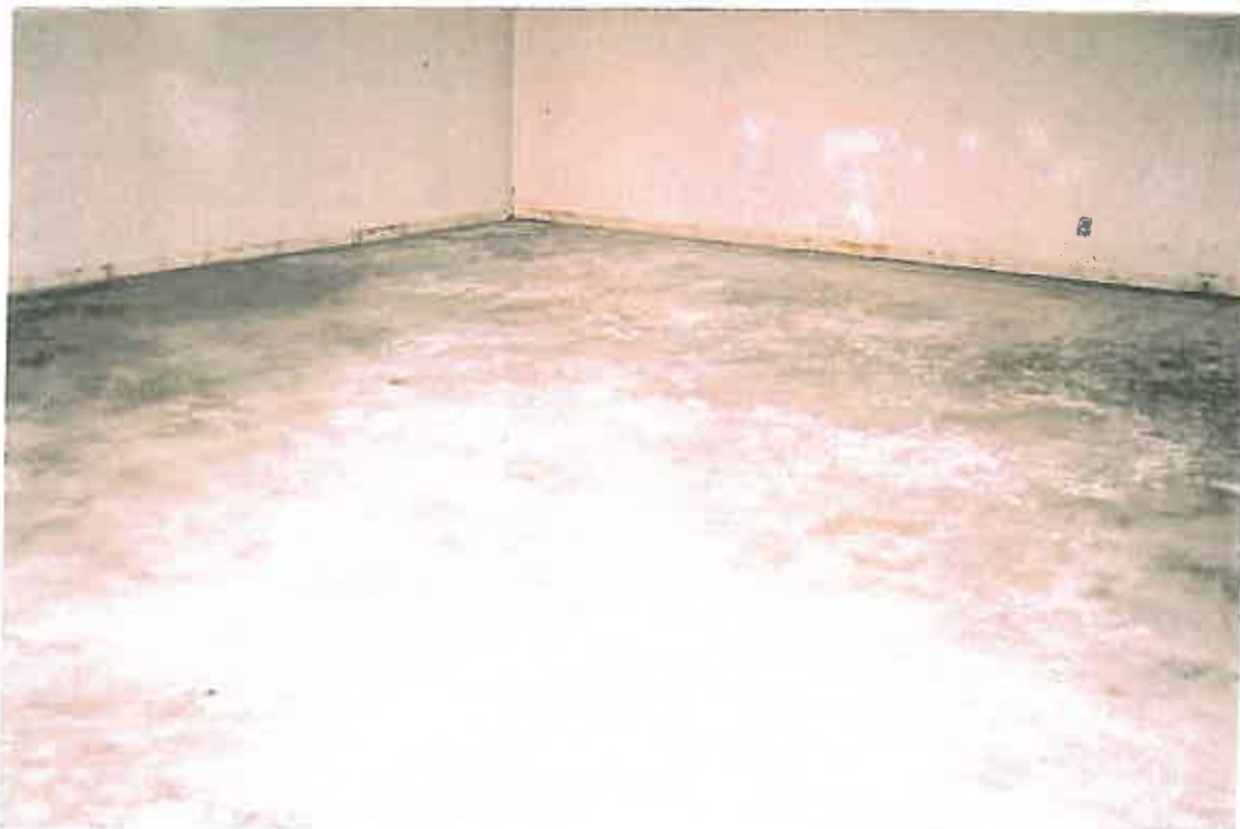
Mastic removed, Room 4
