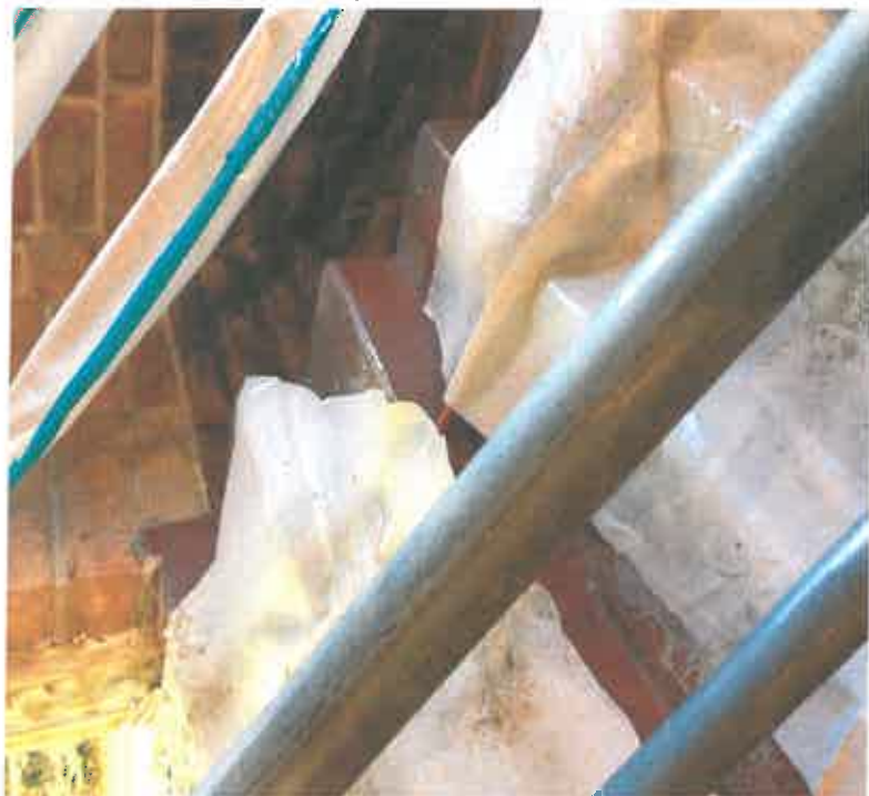
Typical conditon of a striped metal handrail.
