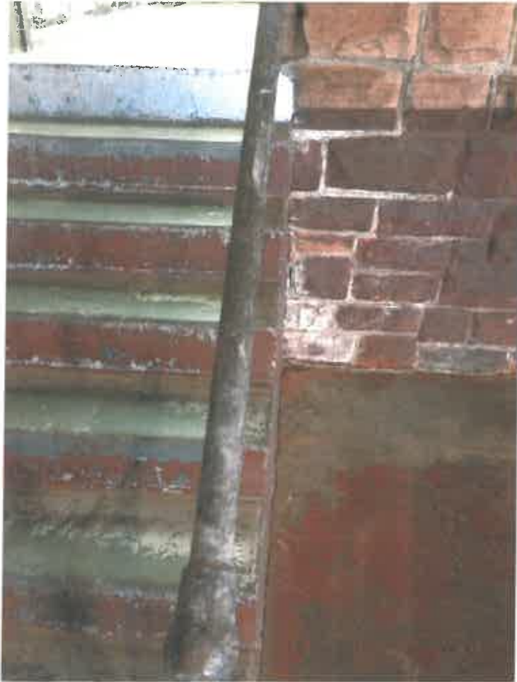
Typical condition of a striped metal handrail.
