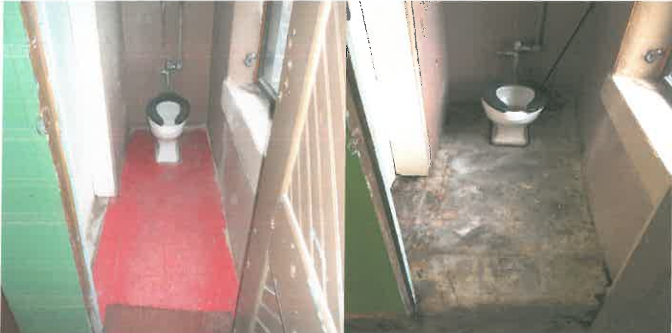
(Bottom) Adjacent bathroom
