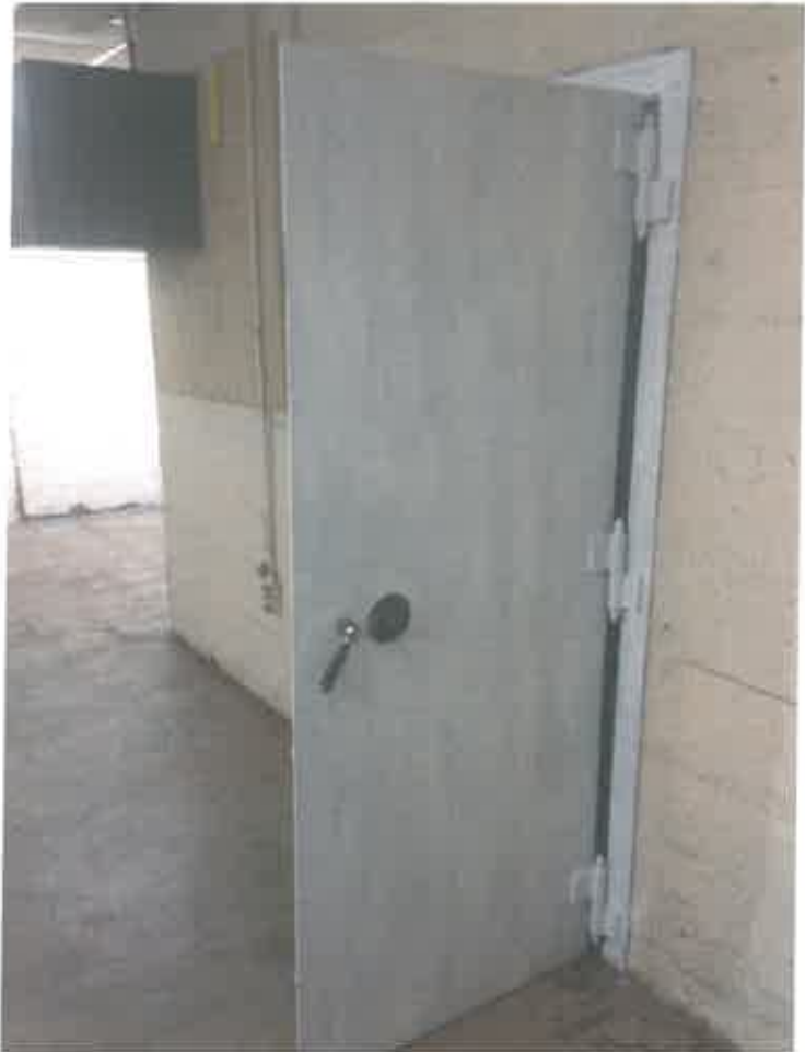
Safe door after lead paint was removed and primer.
