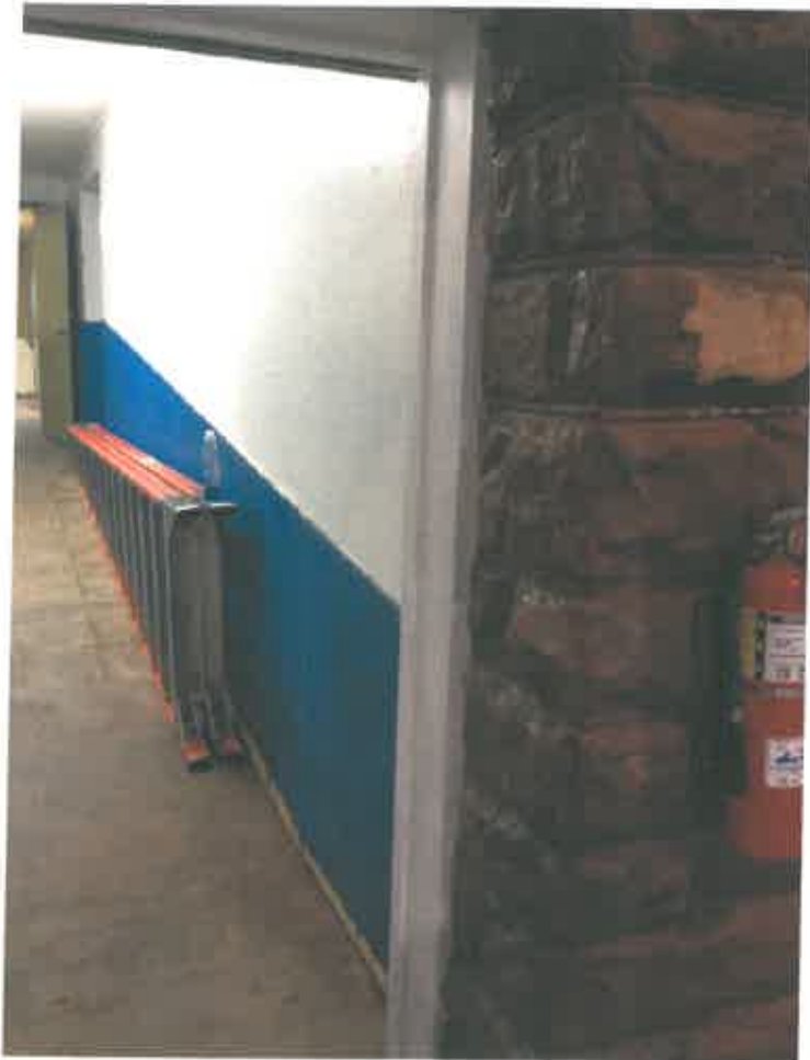
Typical conditon of a primed metal door jamb
