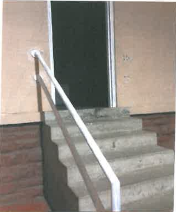
Typical primed metal handrail.
