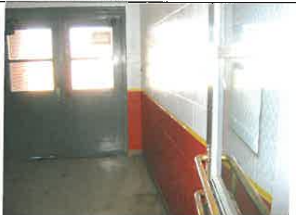
Photo #12: Gray Metal Entrance Doors – Side A Exterior – LBP
