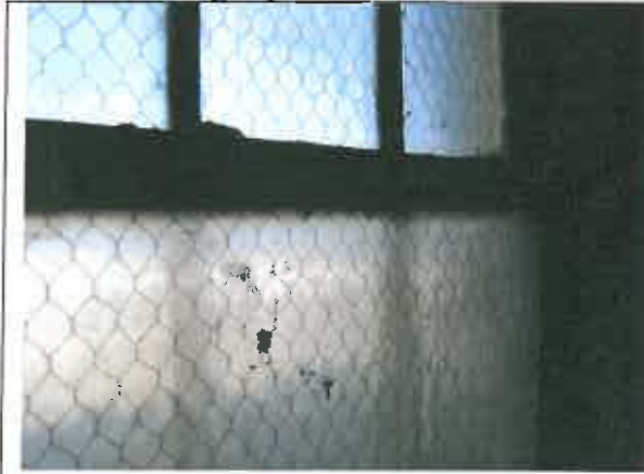
Photo #1: Green Window Frame Room 1 – LBP.
