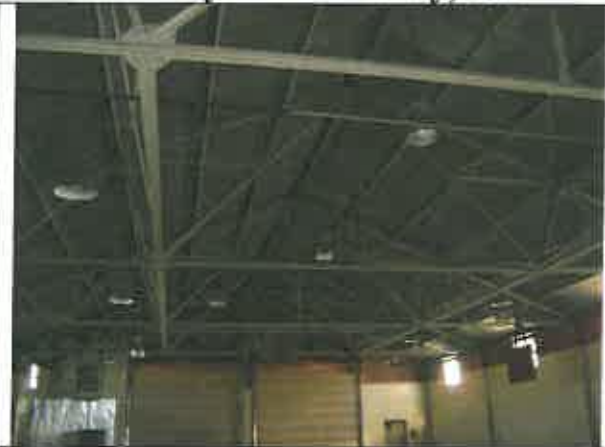
Photo #2: Roof Support Trusses Room 1 – LBP.
