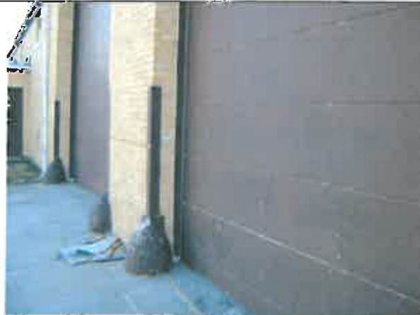
Photo #9: Brown Edge Protectors and Modified Bollard Side C Exterior –LBP.
