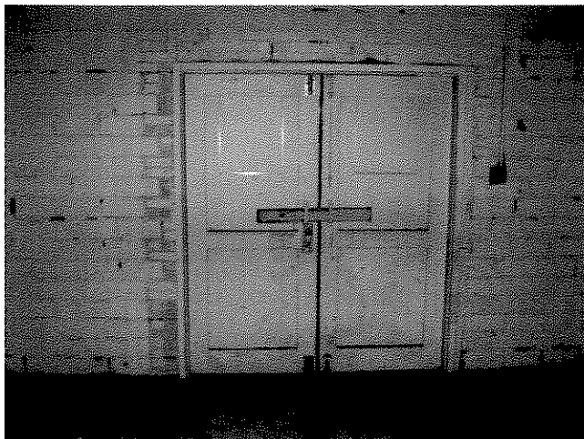
Photo #9: South doors inside the Maintenance Area
