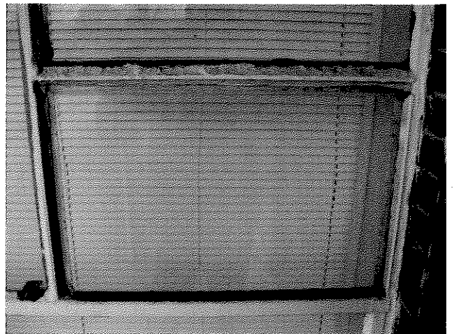
Photo #4: Close-up view of putty on an outside window
