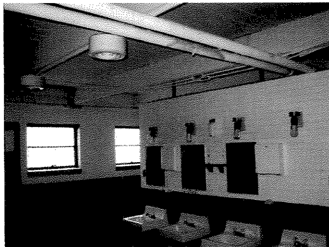
Photo # 17: TSI inside the Enlisted Latrine
