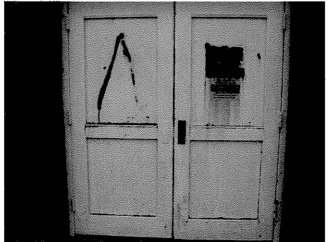
Photo #8: South doors outside the Maintenance Area
