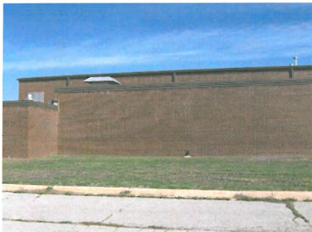
Photo #5: View of IFR vent on the south side
