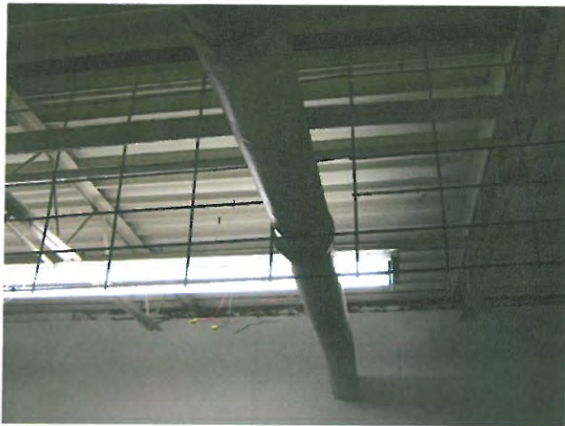
Photo #21: TSI inside the Mop Room
