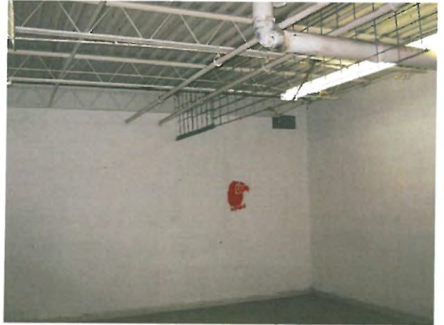
Photo #20: Mop Room with TSI
