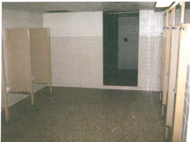
Photo #42: Men's Latrine
