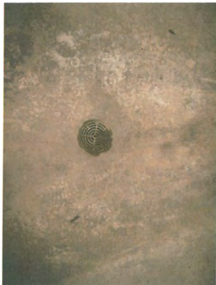
Photo #56: Drain inside IFR
