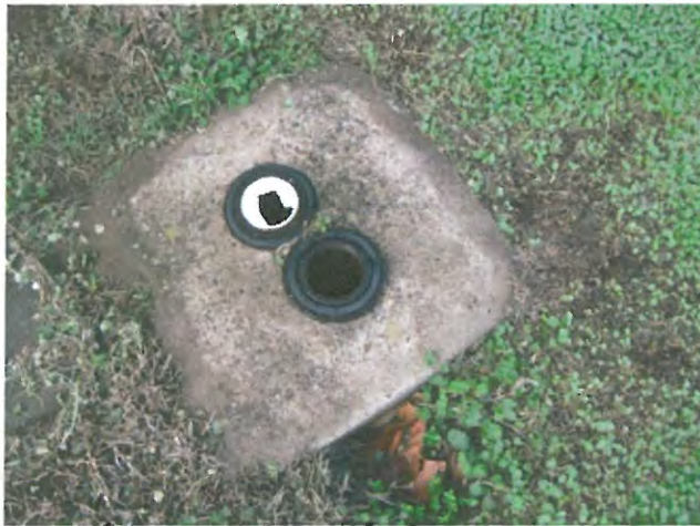
Photo #9: Sewer pipes located on the north side.
