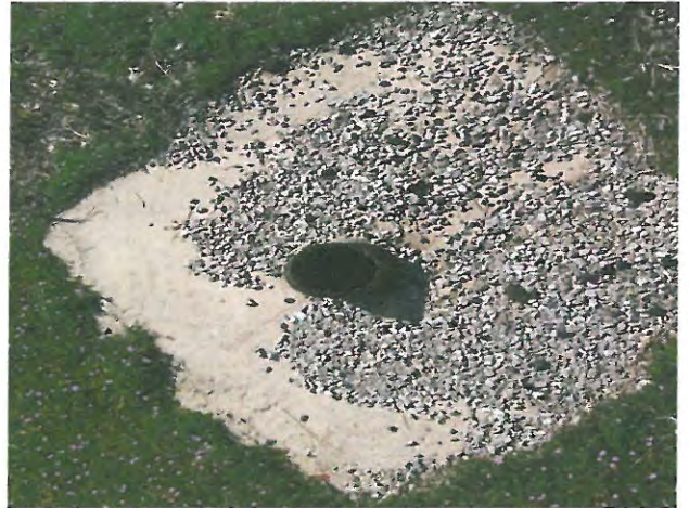
Photo #8: Pipe where the American Flag pole used to be southwest of the Armory.
