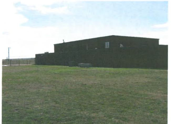
Photo #4: North side facing southeast
