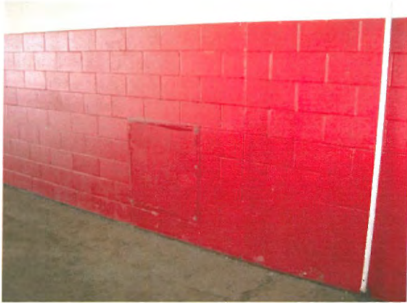
Photo #52: Metal Door opening on the Drill Floor side, which leads underneath the bullet trap.
