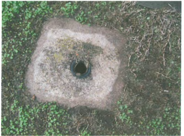
Photo #10: Sewer pipe located on the north side.
