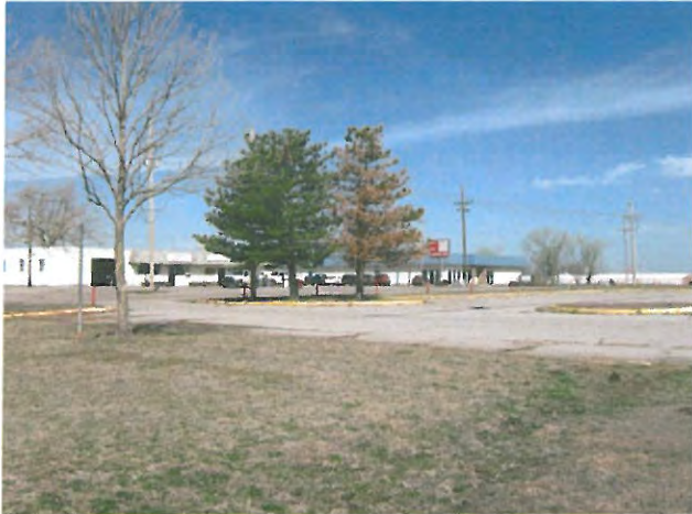
Photo #13: Phipp's BBQ, E & M Oil Company, and the National Rural Water Association across South 13 th Street to the west.
