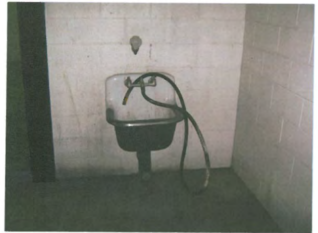
Photo #22: Sink inside the Mop Room
