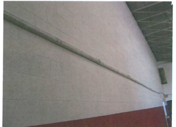
Photo #49: TSI on the south wall of the Drill Floor
