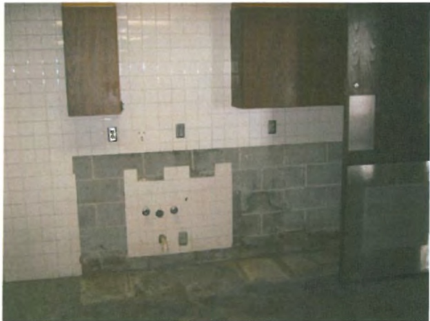
Photo #45: Kitchen with exposed mastic
