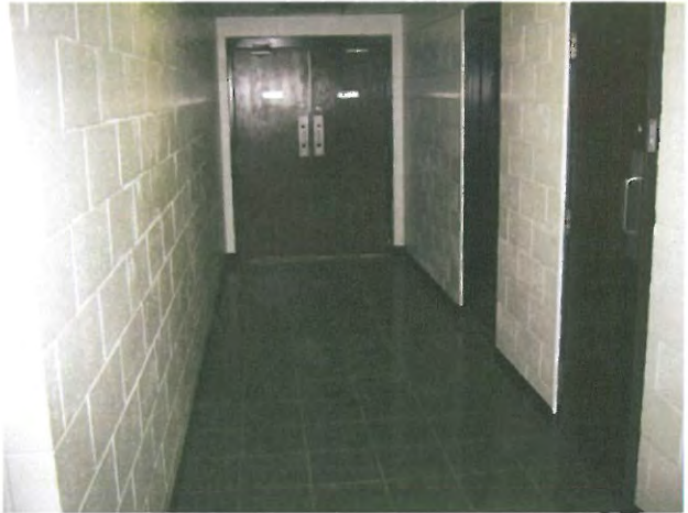
Photo #39: Southwest Hallway
