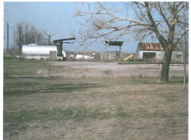
Photo #12: AST's across South 13 th Street.
