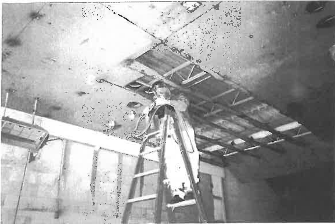
Metal ceiling removal - Indoor Firing Range
