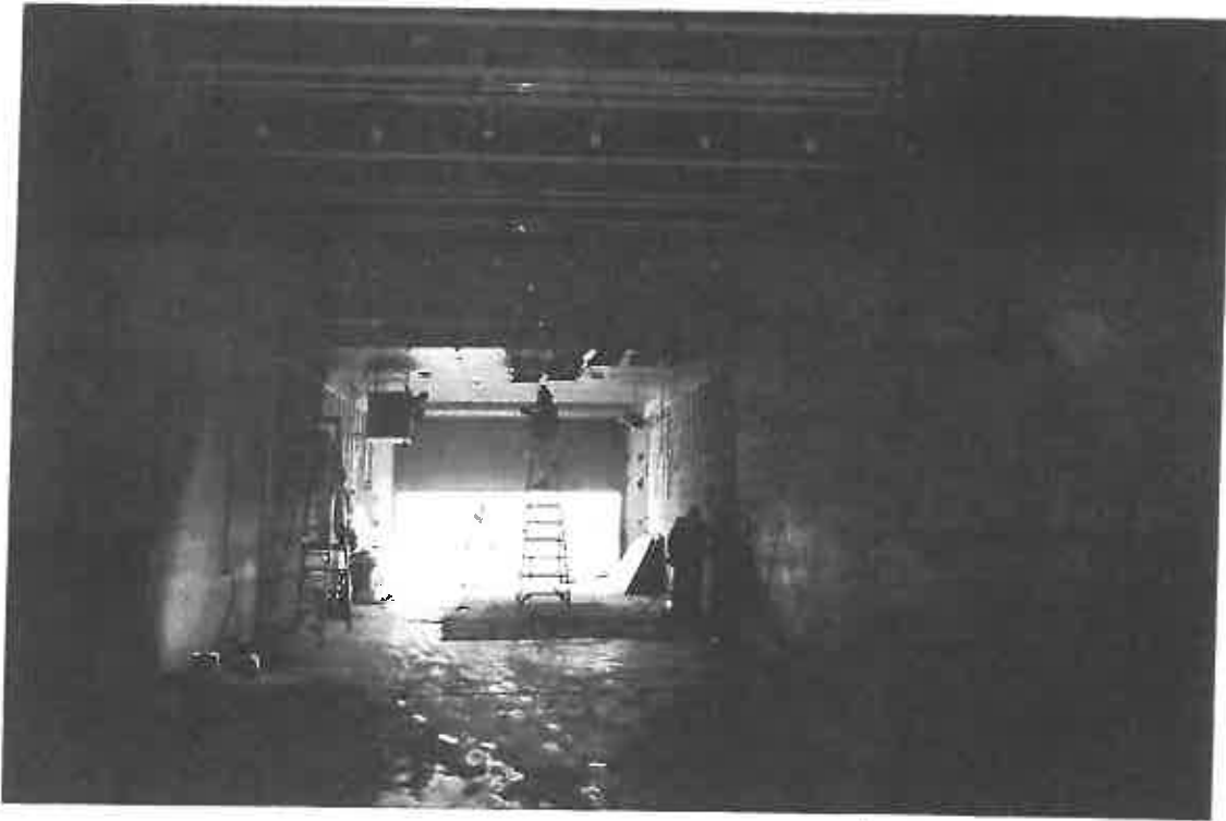
Decontamination/cleaning - Indoor Firing Range
