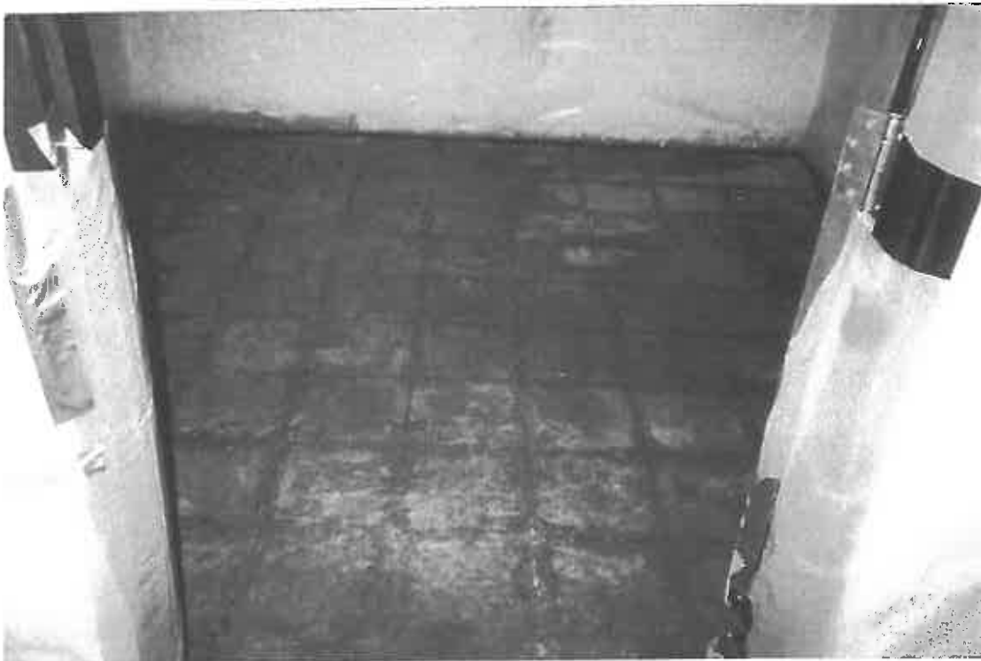
Floor tile and mastic removal - Main building
