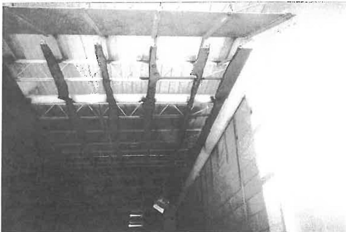
Partial removal of metal ceiling - Indoor Firing Range
