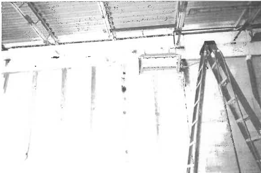
Wall/sound board removal - Indoor firing range
