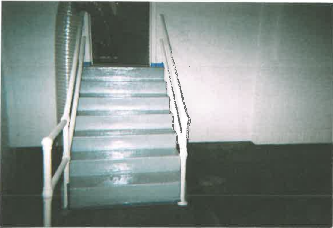
HAND RAILS AND STEPS - SCRAPED AND SEALED
