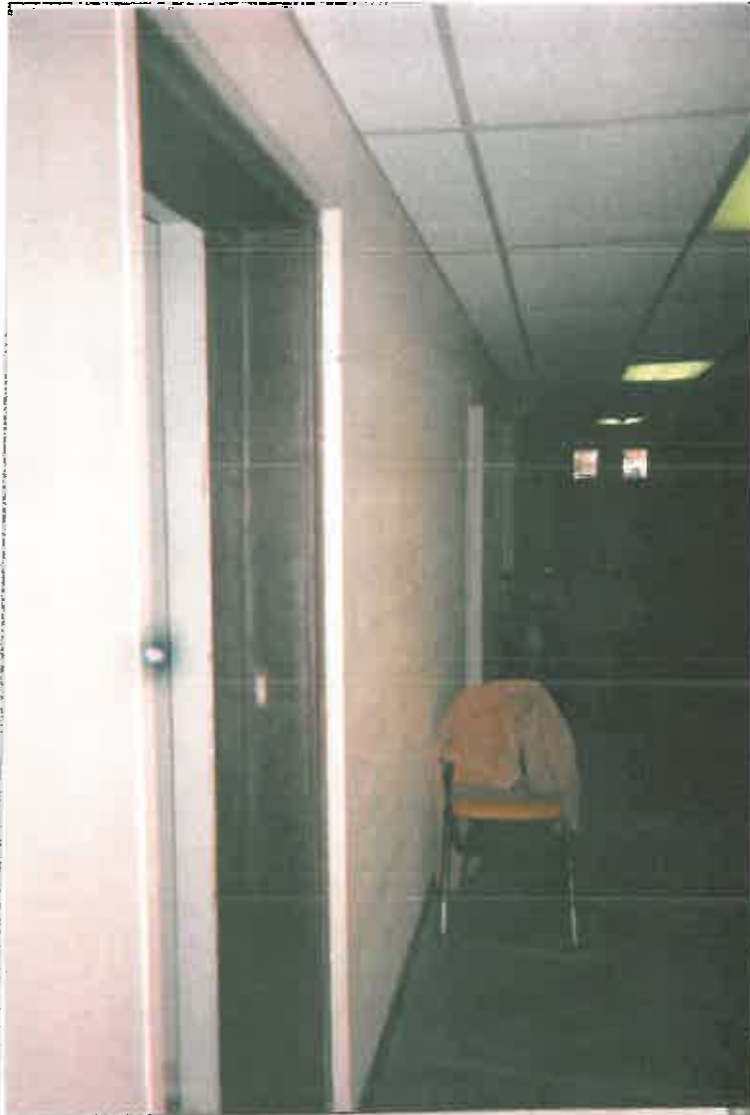
DOOR FRAME, MAIN BUILDING, STRIPPED TO METAL
