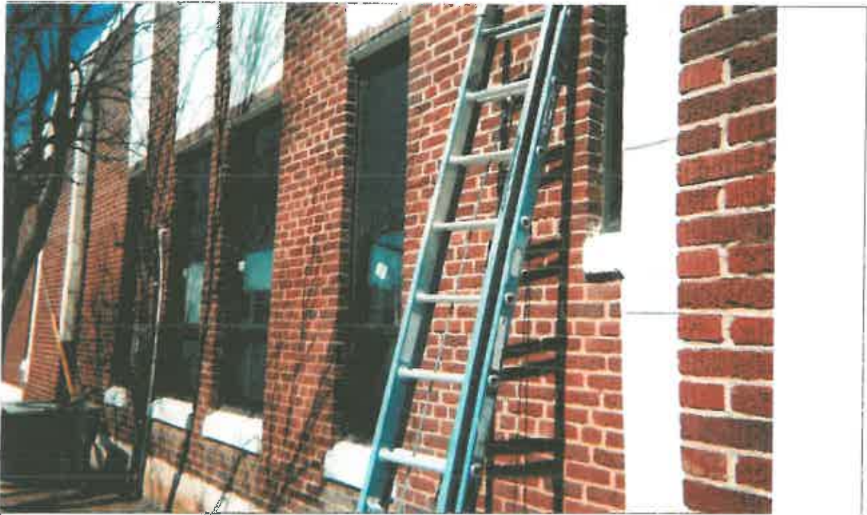
WINDOW LENTELS - SCRAPED AND SEALED
