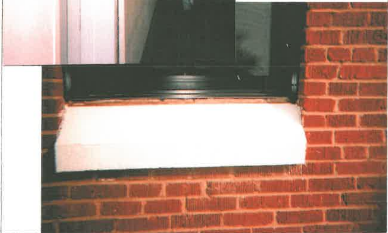
WINDOW LINTELS - SCRAPED AND SEALED
