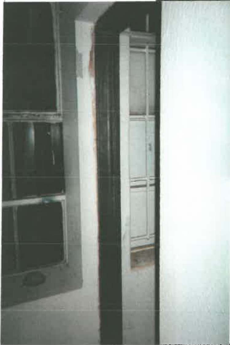
DOOR FRAME, MAIN BUILDING, STRIPPED TO METAL
