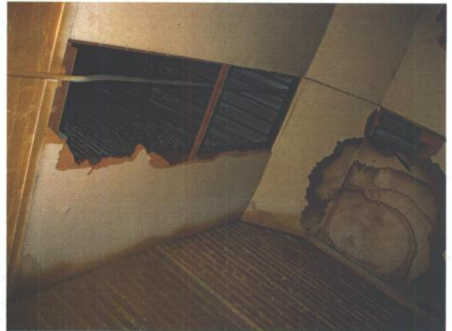
Photo #14: Ceiling in the Stage area.
