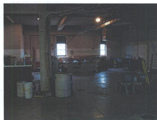
Photo #6: West side of the Battalion Supply Room. 55-gallon drums located on the northwest corner.
