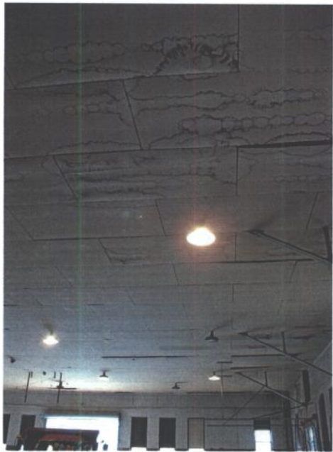
Photo #13: Ceiling in the Drill Hall.
