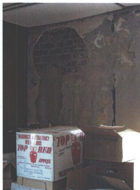
Photo #12: West wall of the CDR's Office on the second floor.
