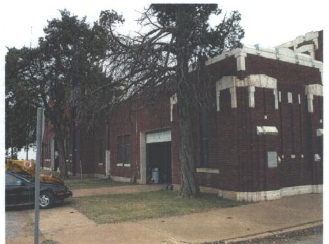
Photo #18: East and northeast corner view of the armory building.
