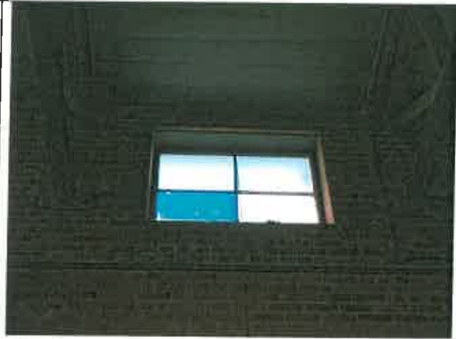
Reading 368, Room 18, Metal Window Headers
