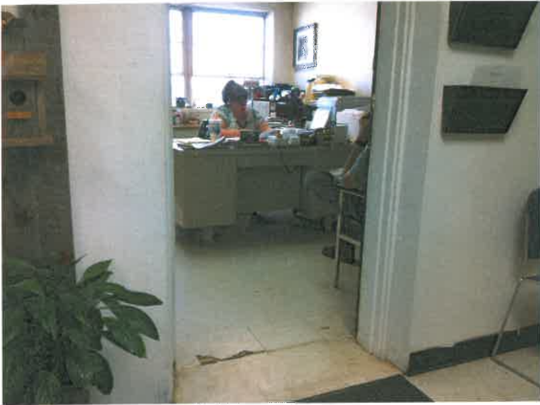
Non-Friable Gray Floor Tile (Sub-Layer) in Room 12 (Sample # BA-04A)
