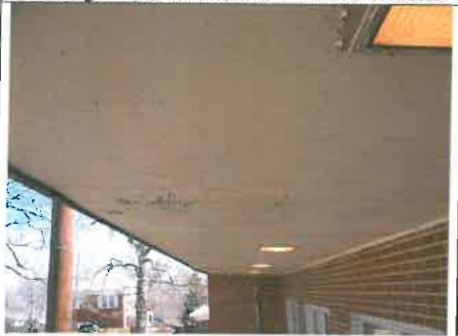
Reading 537, Exterior, Metal Porch Ceiling
