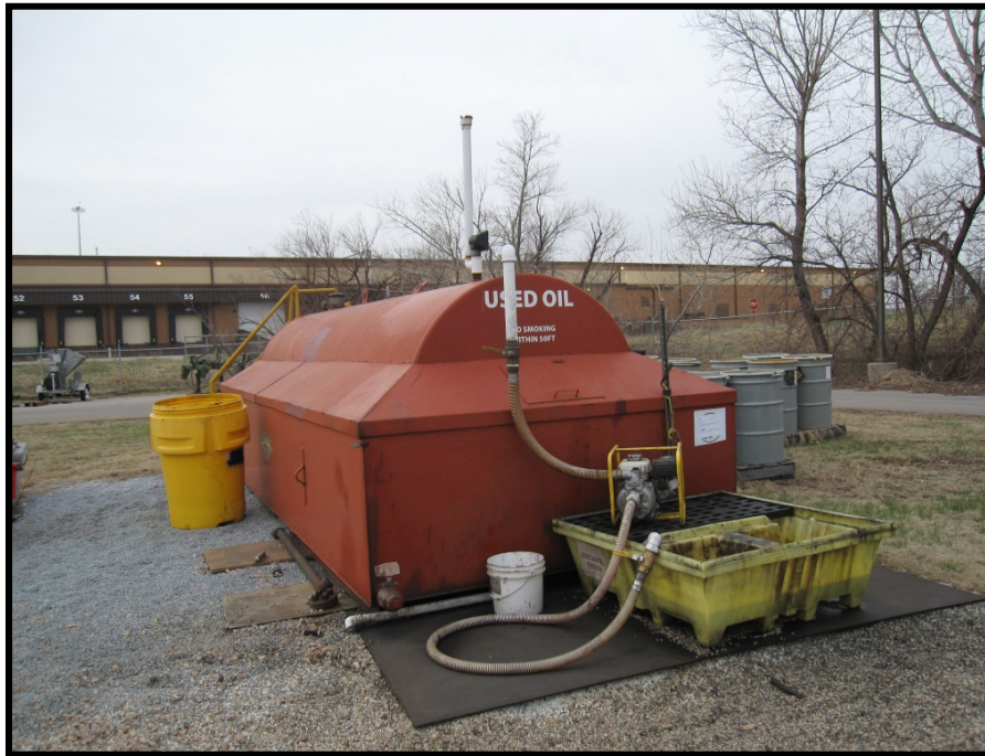
Barrel Yard Storage Tank 809-1
