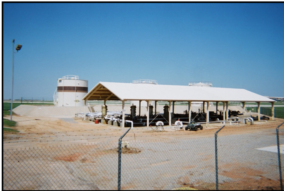
AWACS Alert Area Building 995 Pumphouse Filter Separators located inside
