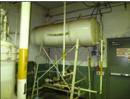
Tank: 3234-B South
