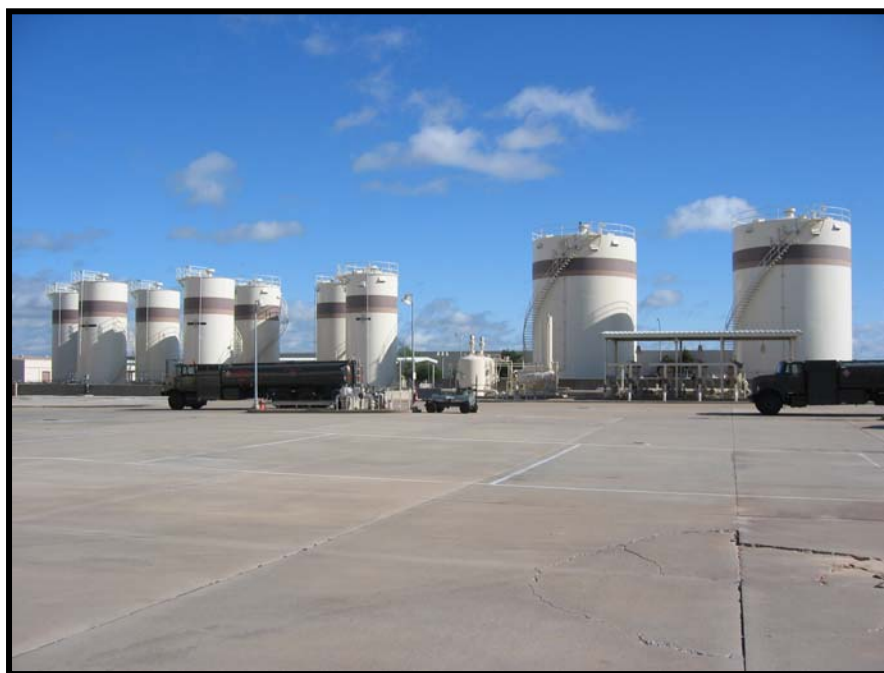
290 Fuel Yard Tanks 337, 335, 338, 334, 341, 332, 333, 331, 330 (from left to right) R-11 Fill-stand (foreground) Filter Separators (in front of Tanks 331, 330)
