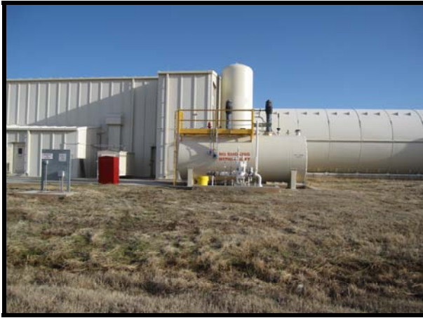
TAC Area T-9 Test Cell Fuel Daytank
