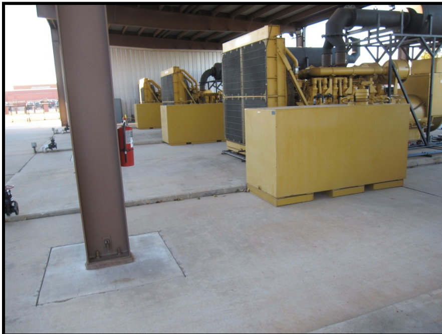
DISA Tanks 3900-DT-1, 2, and 3
