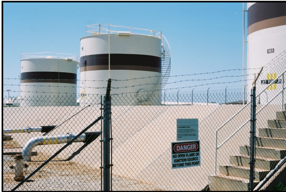
AWACS Alert Area Tanks 999, 998, 965 (left to right)
