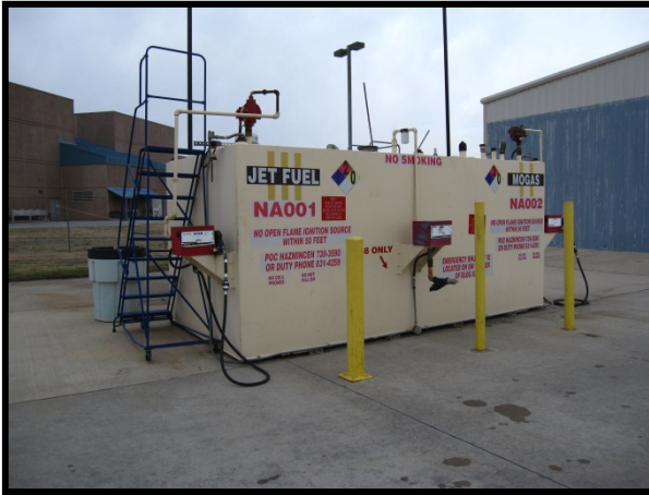
Navy Stratcom AGE Equipment and Fueling Facility: Fuel Tanks NA001 and NA002.
