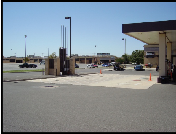
AAFES Shoppette Vaulted ASTs to supply fuel pumps.
