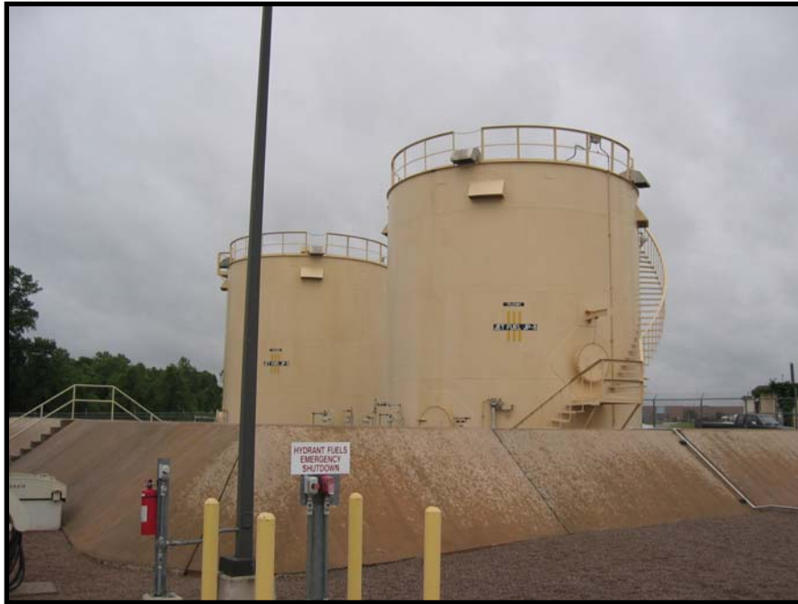
507th Fuel Yard Emergency Shutoff Switch at Foreground
