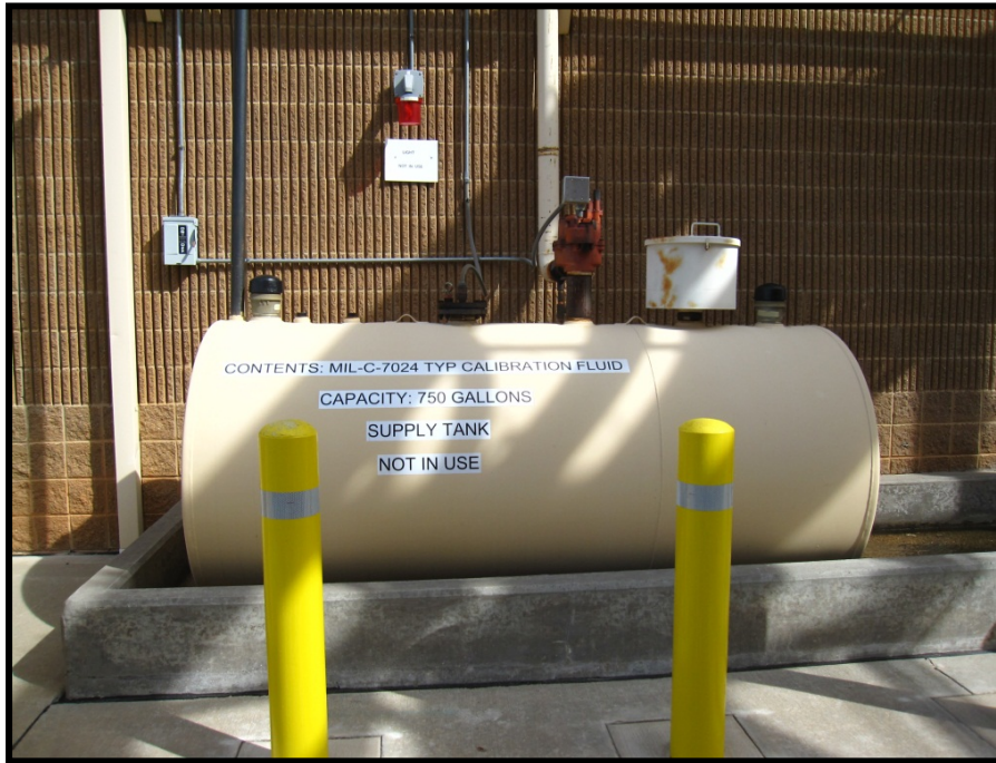
Building 200, Air Driven Accessories Test Tank 200A – New Calibration Fluid Supply Tank Not in Use
