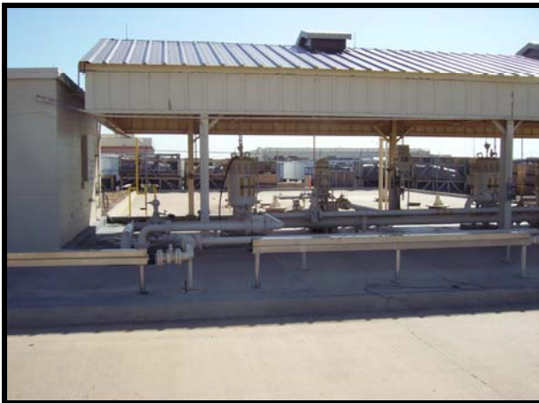
Purge Facility Pump House (Building 2112) and Truck Loading Area. UST area in background.
