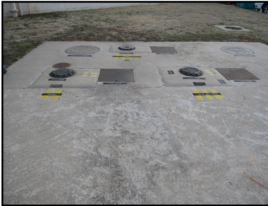
Transient Alert Tanks 286 and 287
