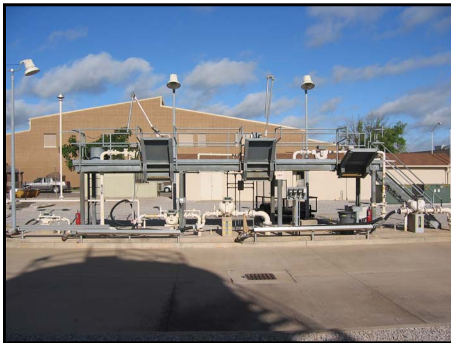
290 Fuel Yard Multi-Product Loading Rack
