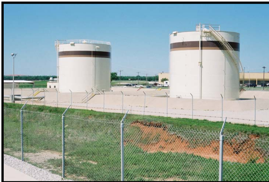
Phillips System - Tanks 483 & 484
