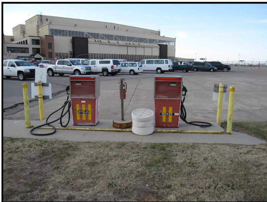
Transient Alert Fuel Pumps served by Tanks 286 and 287
