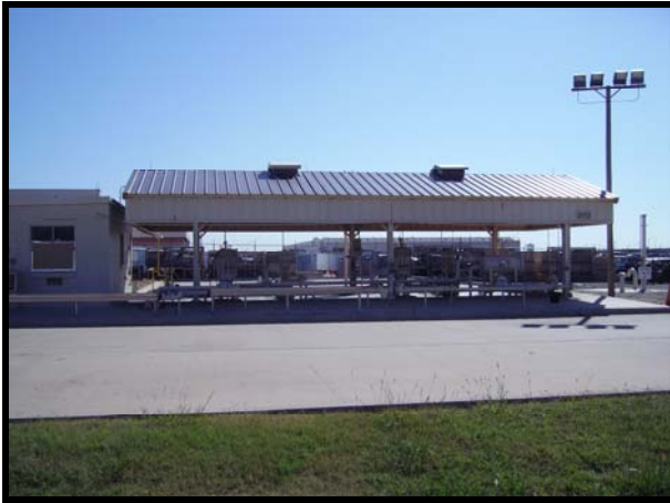
Purge Facility Pump House (Building 2112) and Truck Loading Area
