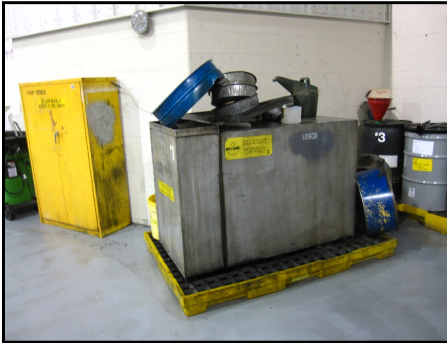
Motor Pool, Building 1130 Used Oil Tank 1130-1
