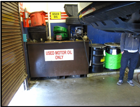
AAFES Shoppette Firestone Shop – Waste Oil Tank: 472-FS1
