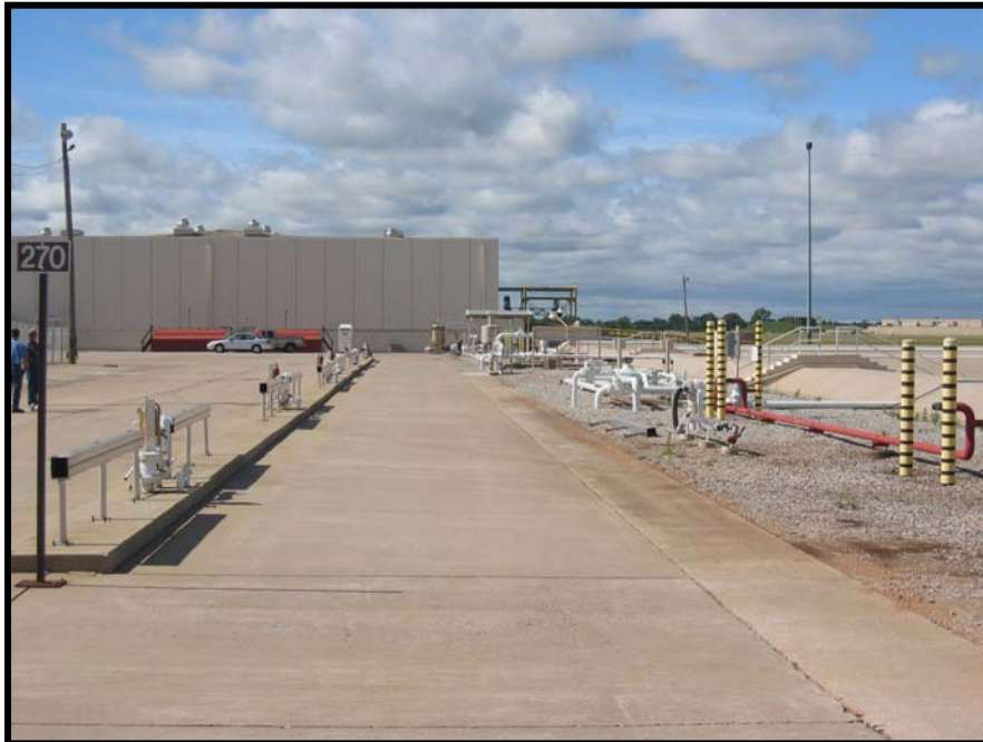
273 Fuel Yard Jet A and Fuel Oil Offloading Headers
