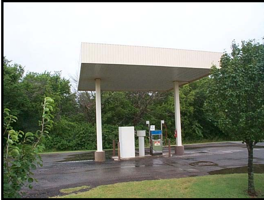
Building 1090 CNG Fill Station
