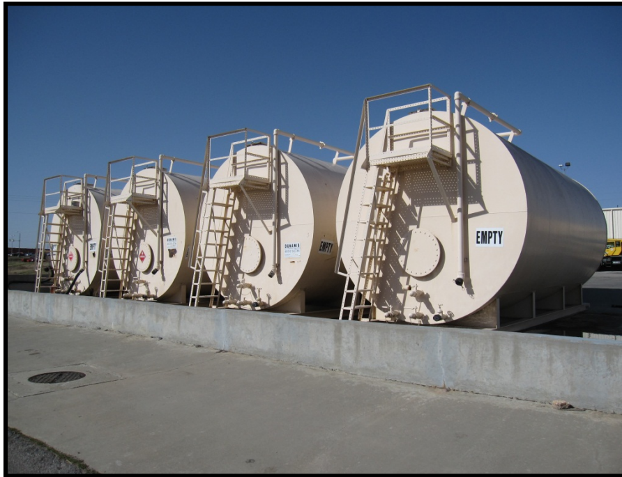
Industrial Waste Treatment Plant (IWTP) Used Oil Tanks 62501-1, -2, -3, and -4
