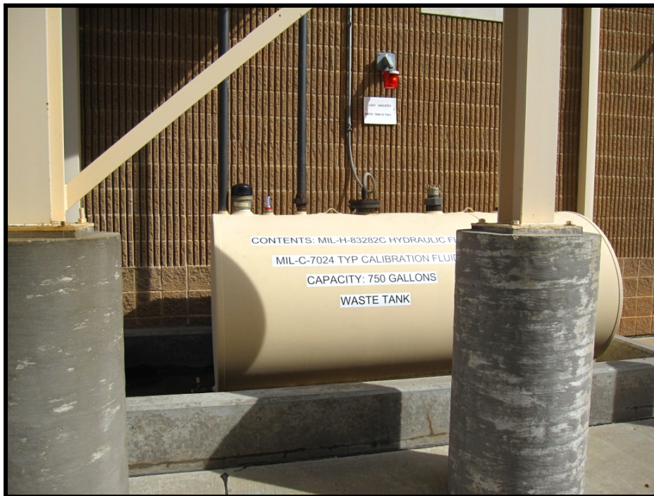
Building 200, Air Driven Accessories Test Tank 200B – Waste Calibration Fluid
