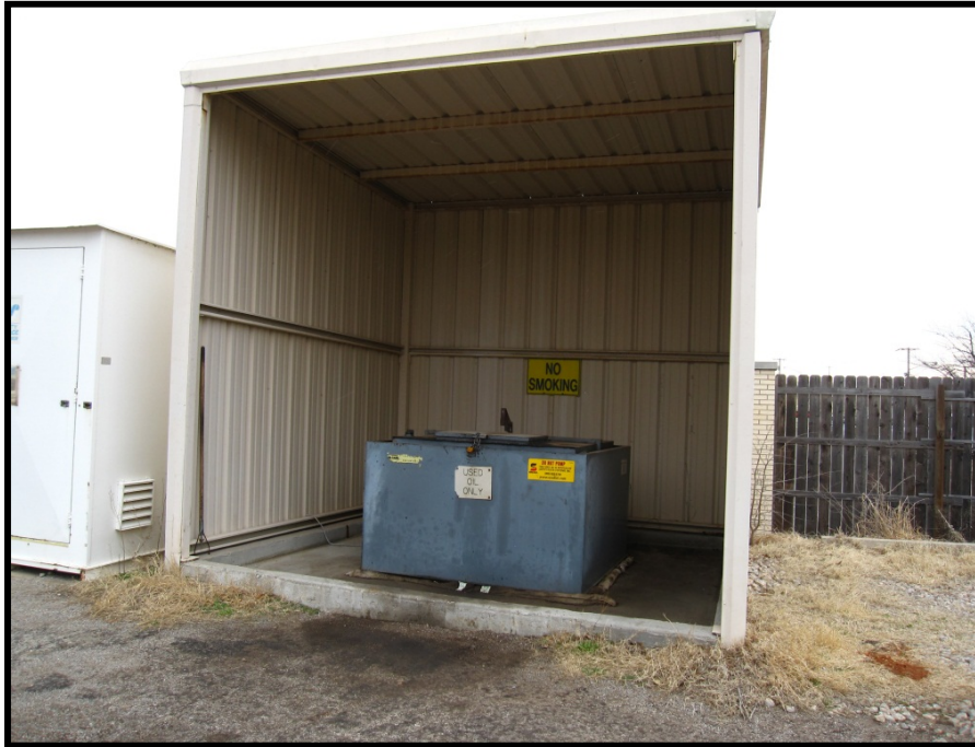
Skills Development Center Used Oil Tank 6002
