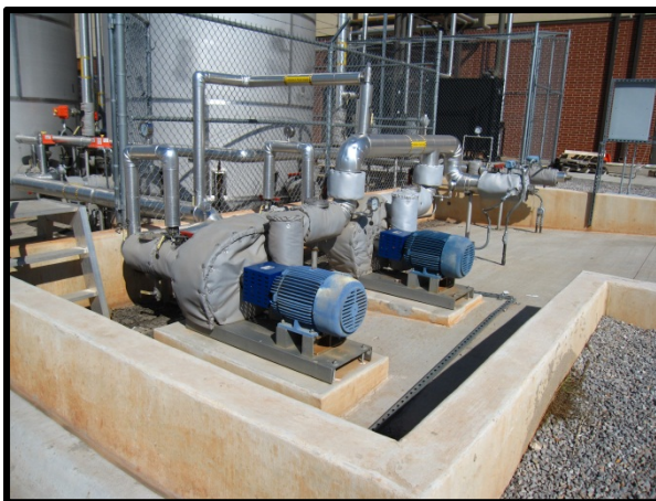
Loading area for AST at Building 3907
