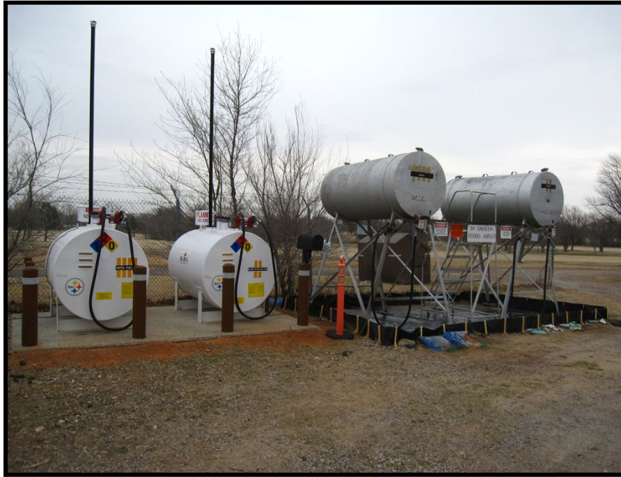
Tinker Golf Course Maintenance Tanks 5935-1 and 5935-2 (Tanks on the right are obsolete as of the time of this photo)
