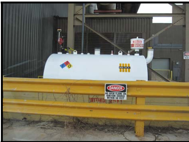
TAC Area Representative Generator
