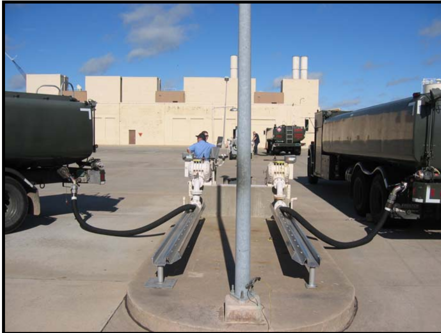
290 Fuel Yard R-11 Refuelers at Jet A Fill-stand
