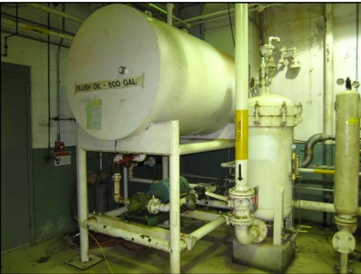
Tank: 3234-A South
