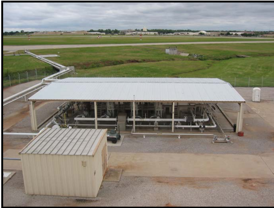
Building 486 Pumphouse Filter Separators inside Fuel lines to Phillips System at upper left corner
