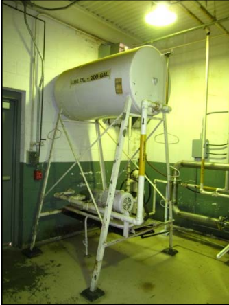
Tank: 3234-C South
