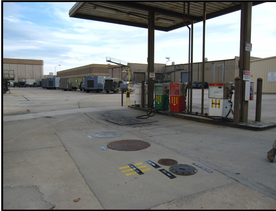
AWEMS/AGEN Tank 264R and fuel pumps
