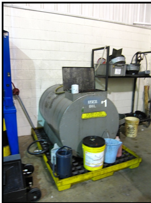
Motor Pool, Building 1130 Used Oil Tank 1130-2
