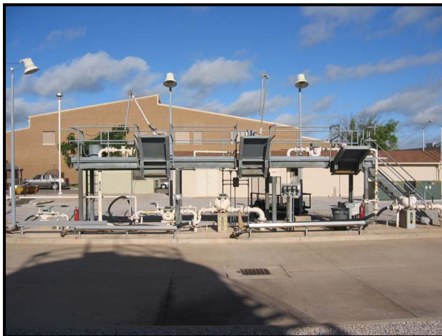
290 Fuel Yard Multi-Product Loading Rack
