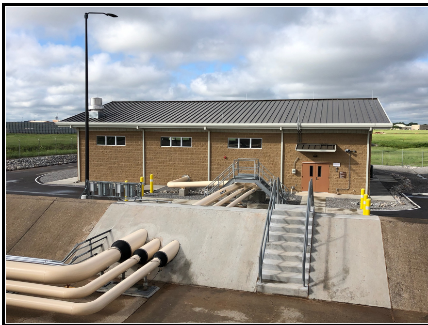
Building 481 Pumphouse Filter Separators inside Fuel lines to MAC System at upper left corner
