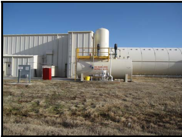
TAC Area T-9 Test Cell Fuel Daytank
