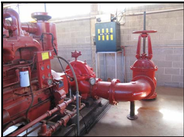
Typical Fire Pump Arrangement, shown with 75-gallon day tank (1032- FP-DT-1)
