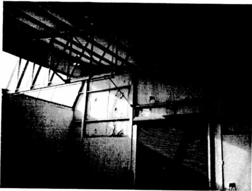
Figure 47. Drill floor looking southwest. Note IFR entrance door left of bay door.
