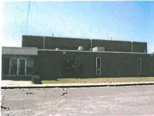
Photo #1: Alva National Guard Armory.
