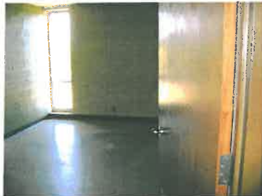
Photo # 6: View of a typical office space.
