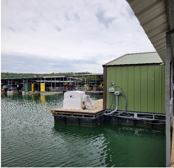
Photo Series #2. Strayhorn Marina on Lake Tenkiller. July 21, 2023 New Pump-out Station for Strayhorn Marina.
