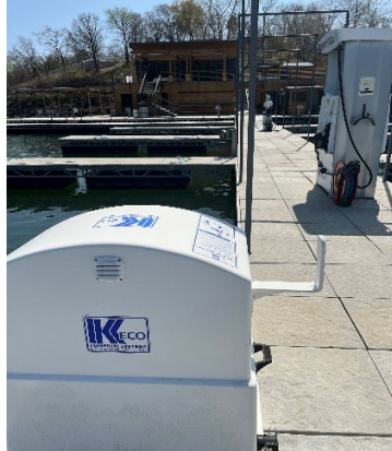
Photo Series #2. Barnacle Bills Marina & Resort September 4, 2024 Holding Tanks, Pump-out systems, shut-off valves, piping under the marina connecting to the aerobic system on land.
