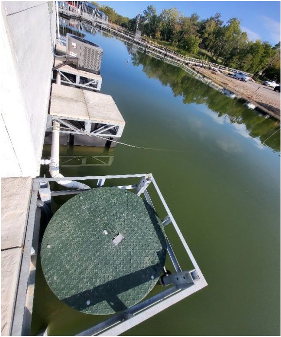
Photo Series #2 Bluewater Bay Marina on Lake Tenkiller. October 5, 2023 New Pump-out Station holding tank and electrical outlet for Bluewater Bay Marina.
