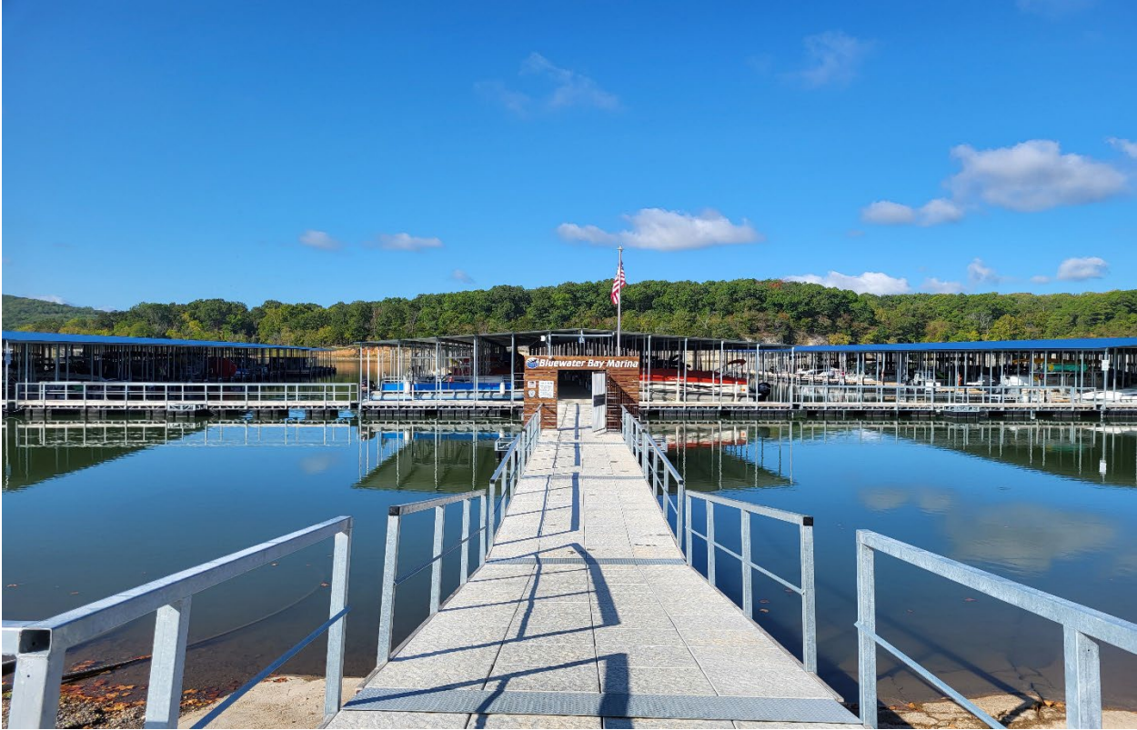
Photo Series #1. Bluewater Bay Marina on Lake Tenkiller. October 5, 2023 Bluewater Bay Marina and Front Entrance and Floating Restrooms
