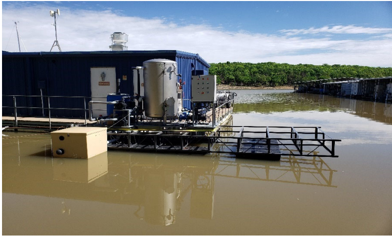
Photo Series #2. Redbud Marina & RV Park. May 5, 2021 New Pump-out station with new piping to boat dock & lateral lines
