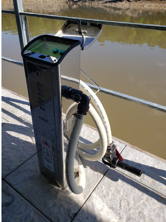
Photo Series #3. Redbud Marina & RV Park. May 5, 2021. Pump-out dock with hose for boats to hook up their tank to dispose of their sewage.
