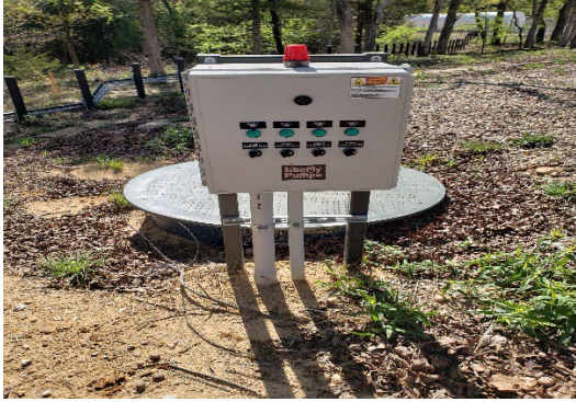
Grinder pump for sewage/Connecting pips from lift station to grinder pump.
